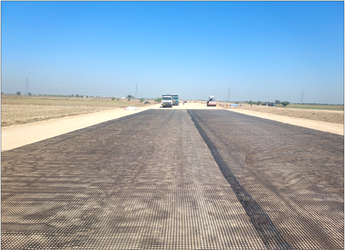
Photo 6 : Road view after laying of TechGrid Geogrid
