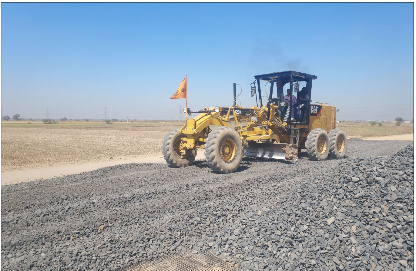
Photo 5 : Compaction of the Base Course Material
