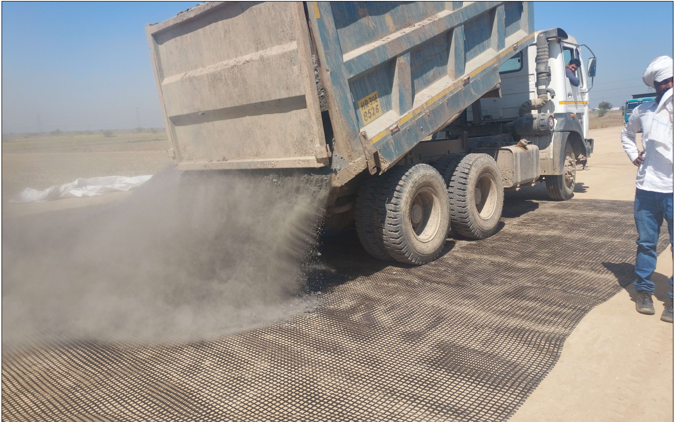
Photo 4 : Placing the Base Course Material on the Geogrid Layer
