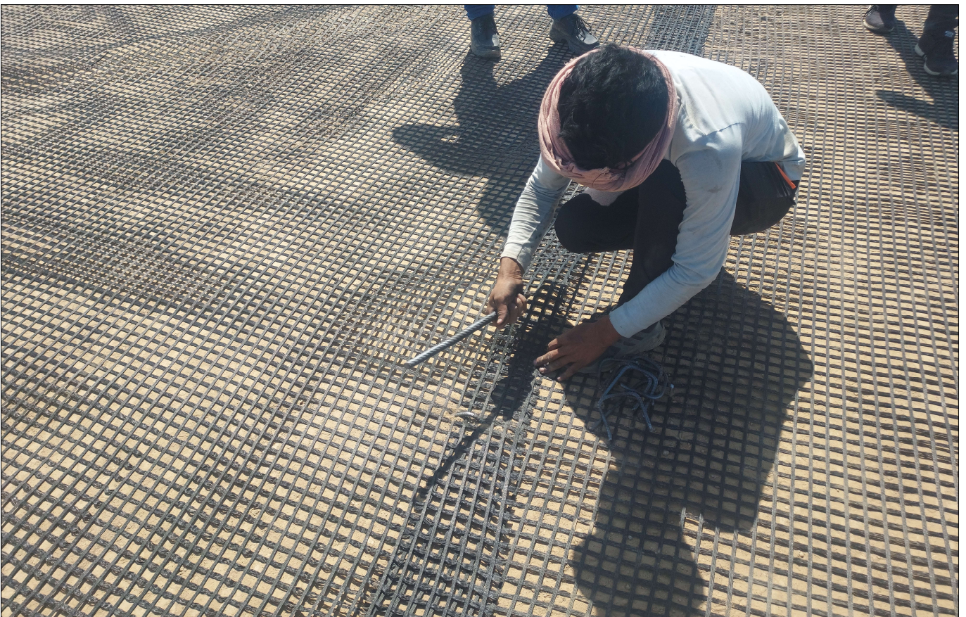
Photo 3 : Overlap of 300mm maintained for adjacent rolls
