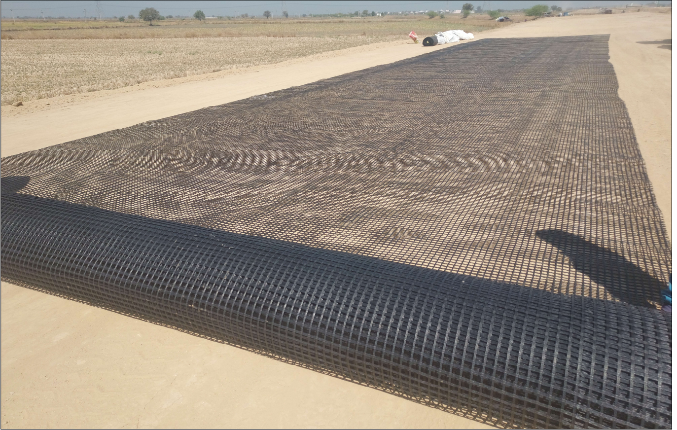
Photo 2 : Laying of TechGrid Geogrid
