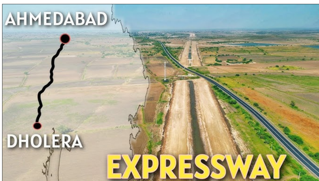
Photo 1 : Ahmedabad - Dholera Expressway
