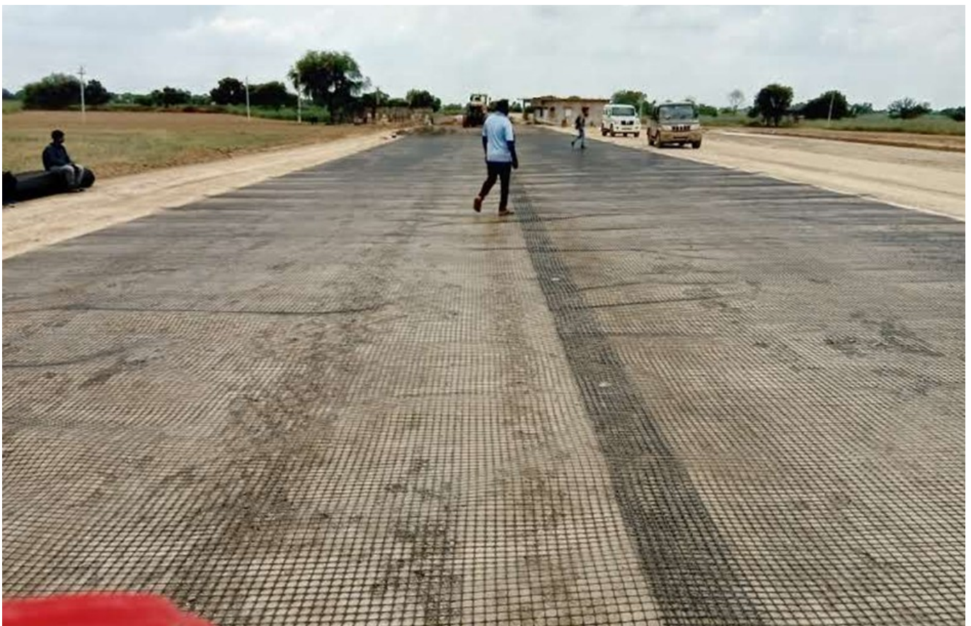
Photo 4 : Laying of the geogrid over prepared GSB layer with a minimum overlap of 300 mm
