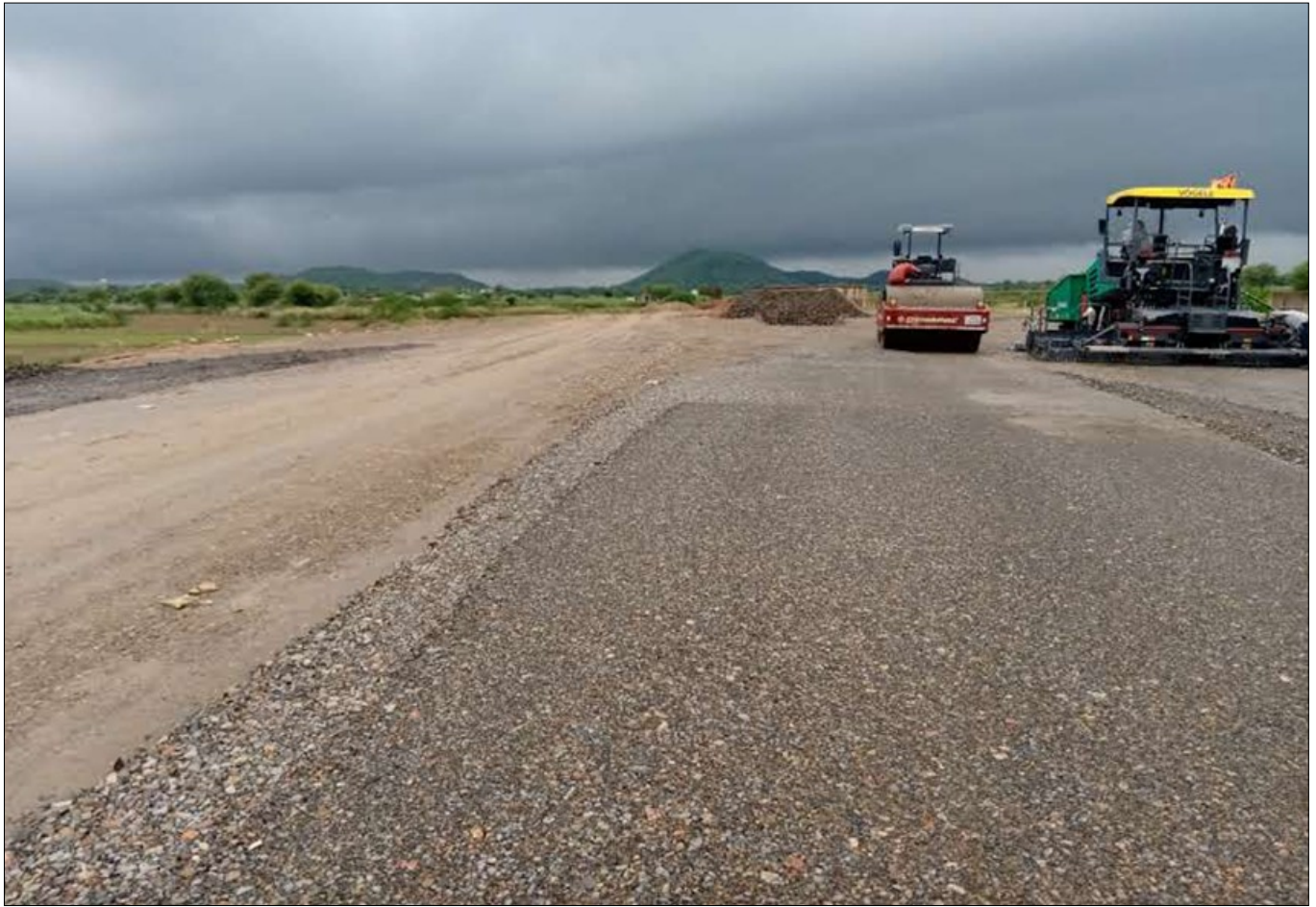
Photo 6 : Compacted WMM Layer
