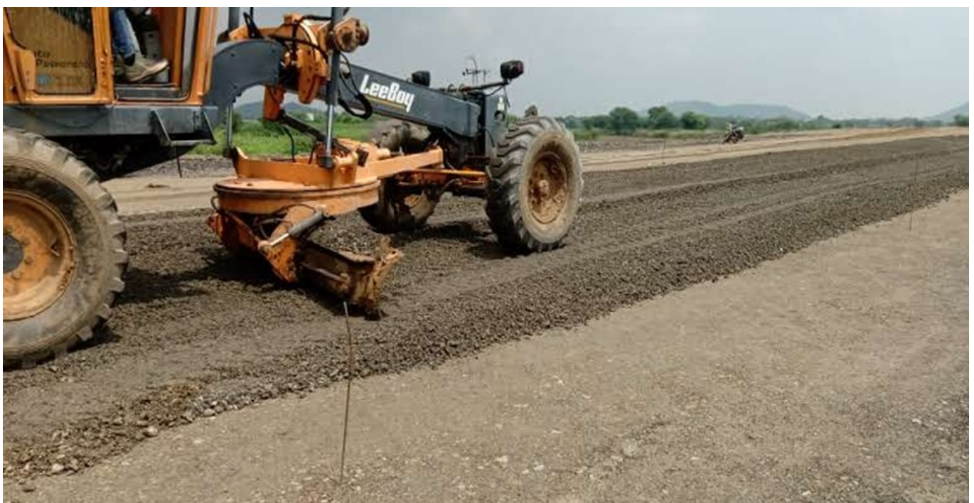
Photo 5 : Dumping and spreading of WMM material over Geogrid
