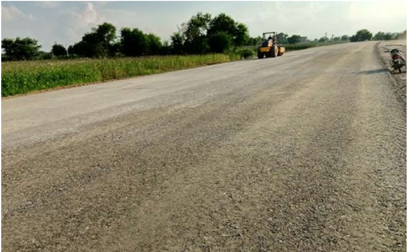
Photo 3 : Finished GSB layer
