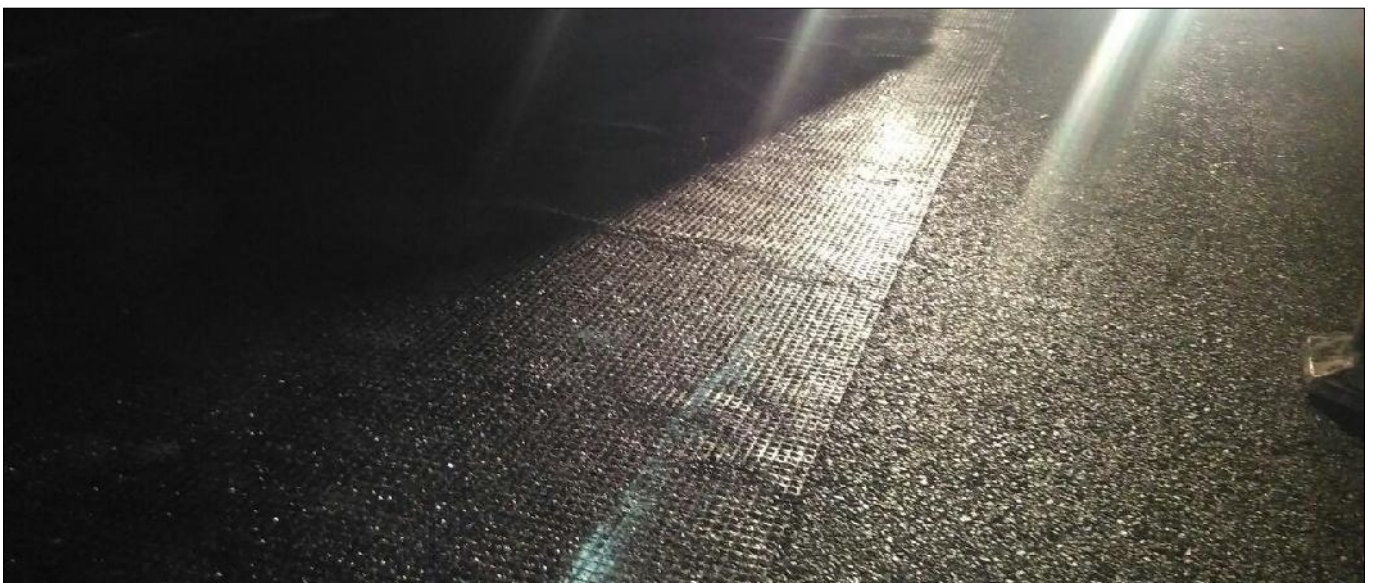
During Construction Photographs
