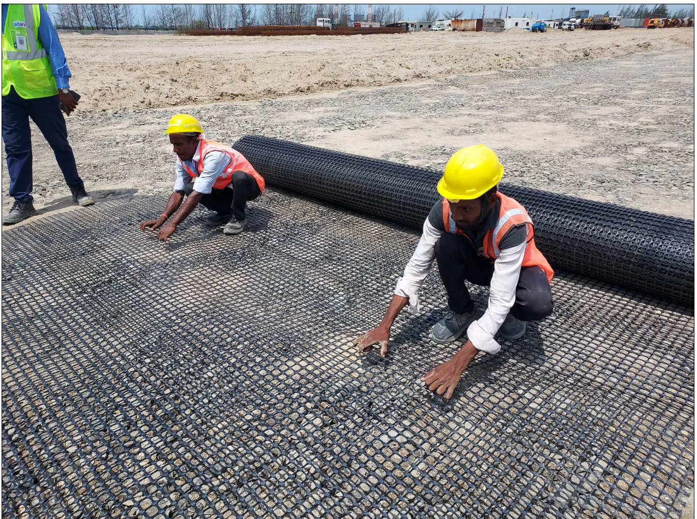
Photo 8 : Applying tension by hand to minimize wrinkles in Geogrid
