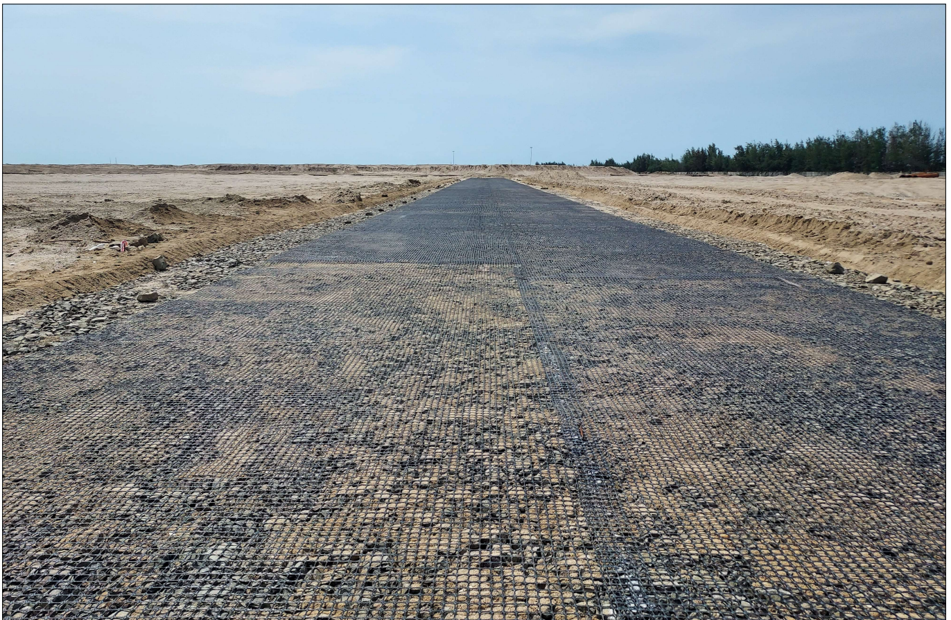
Photo 7 : - Installed geogrid over GSB layer
