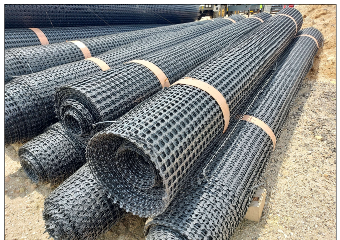
Photo 4 & 5 : Rolls of Techgrid PP biaxial Geogrid ready to install
