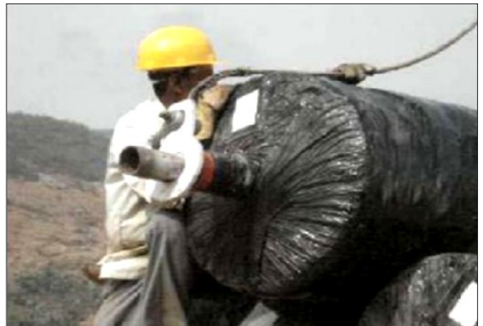
Photo 2 & 3 : Handling of Geosynthetic roll
