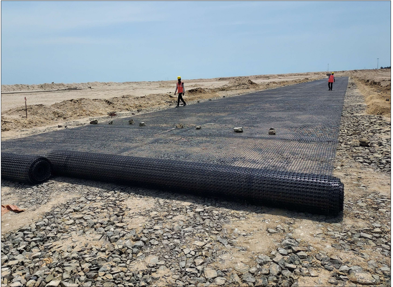
Photo 10 : During Construction Photograph
