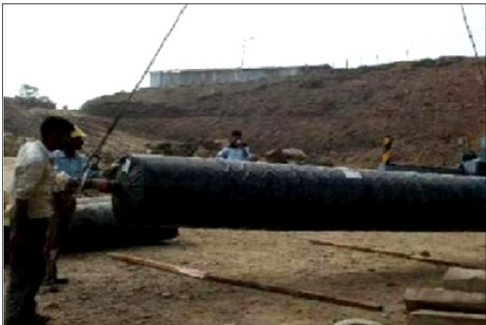
Photo 2 & 3 : Handling of Geosynthetic roll
