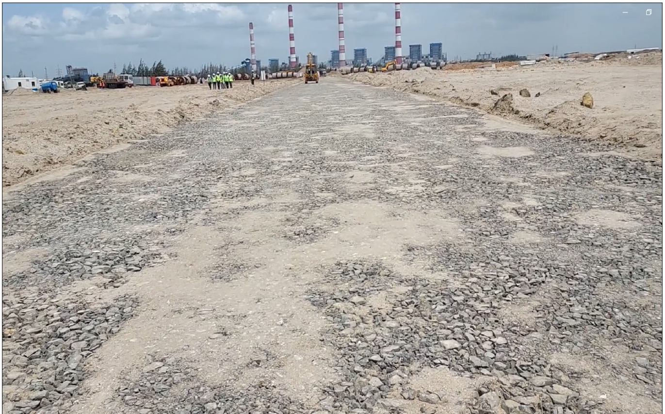
Photo 1 : Prepared Surface for Laying Geogrid
