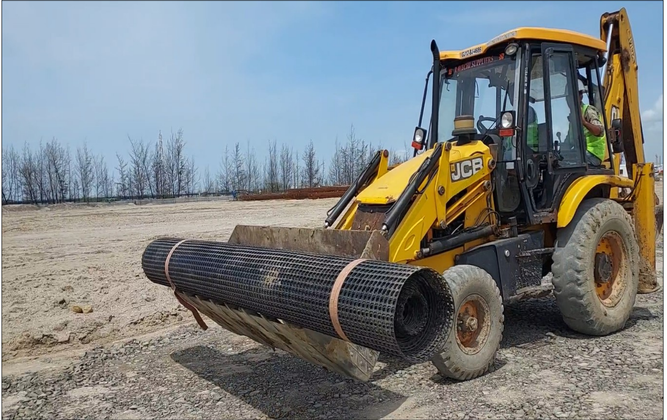
Photo 6 : Carrying Geogrid for installation
