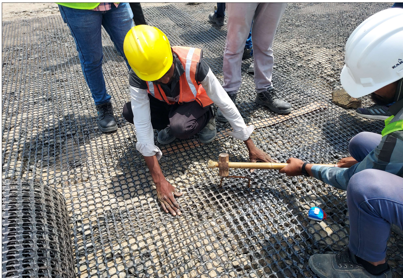
Photo 9 : Overlapping of 150 mm Geogrid at the edge and fixing it with 12 mm U bar
