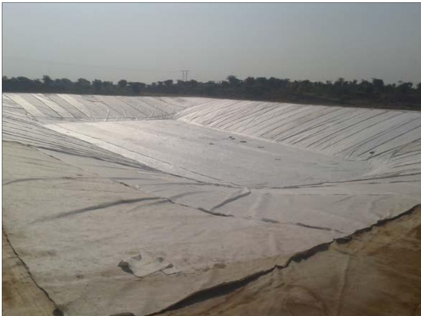
TechGeo Laying Completed at Landfill Site
