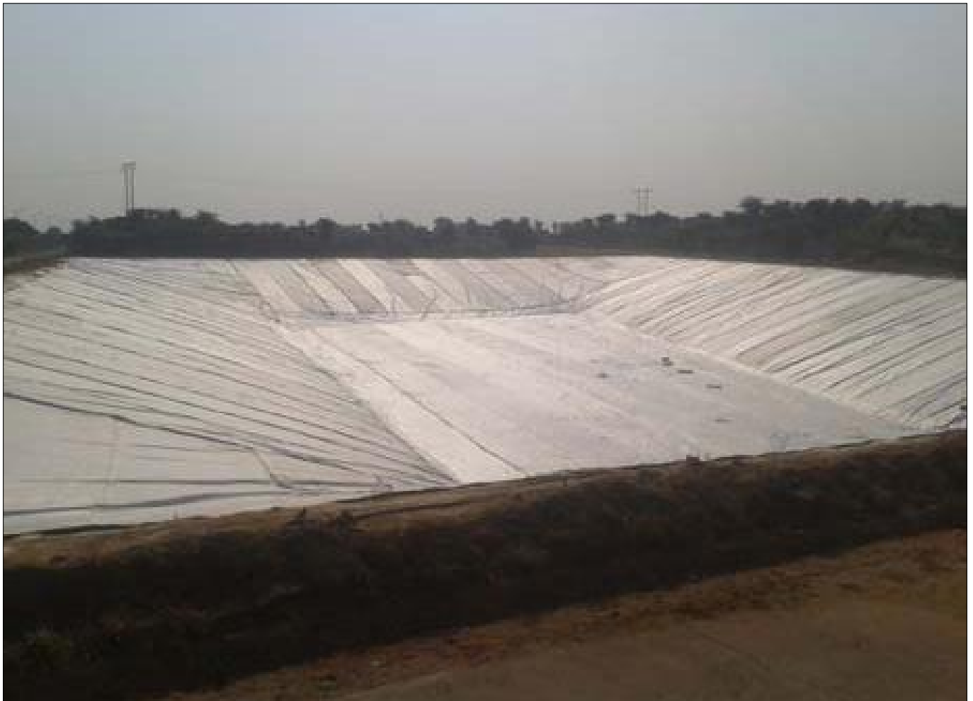
Top View – Himmatnagar Landfill Site
