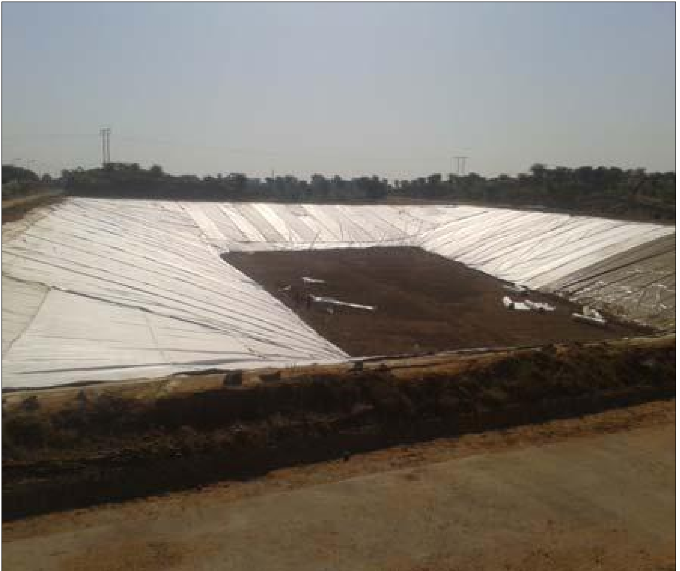
Top View – Himmatnagar Landfill Site
