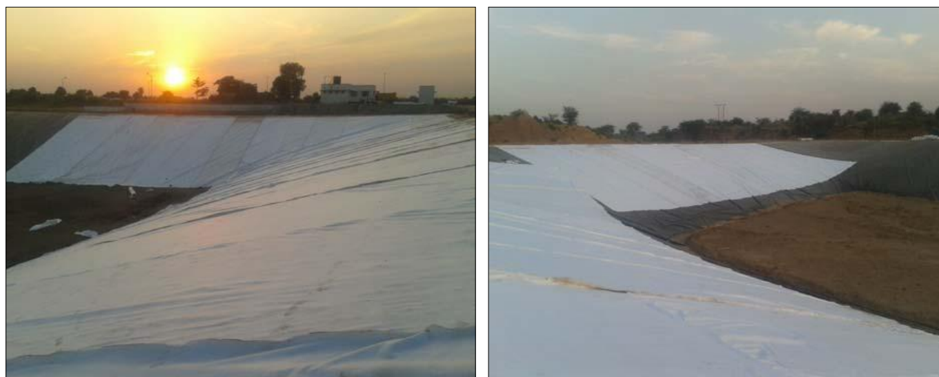
TechGeo laid over the Side Slopes of Landfill
