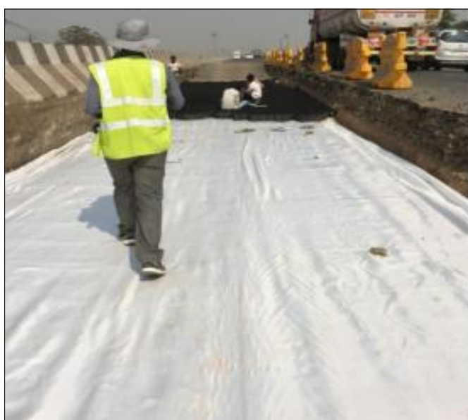
High Strength Woven PET Geotextile laid
