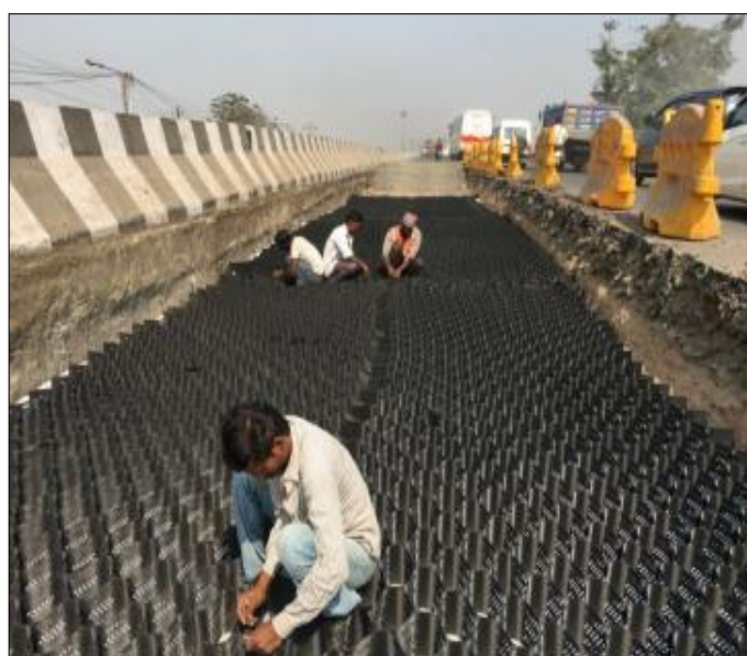
Techcell geocell tying in progress
