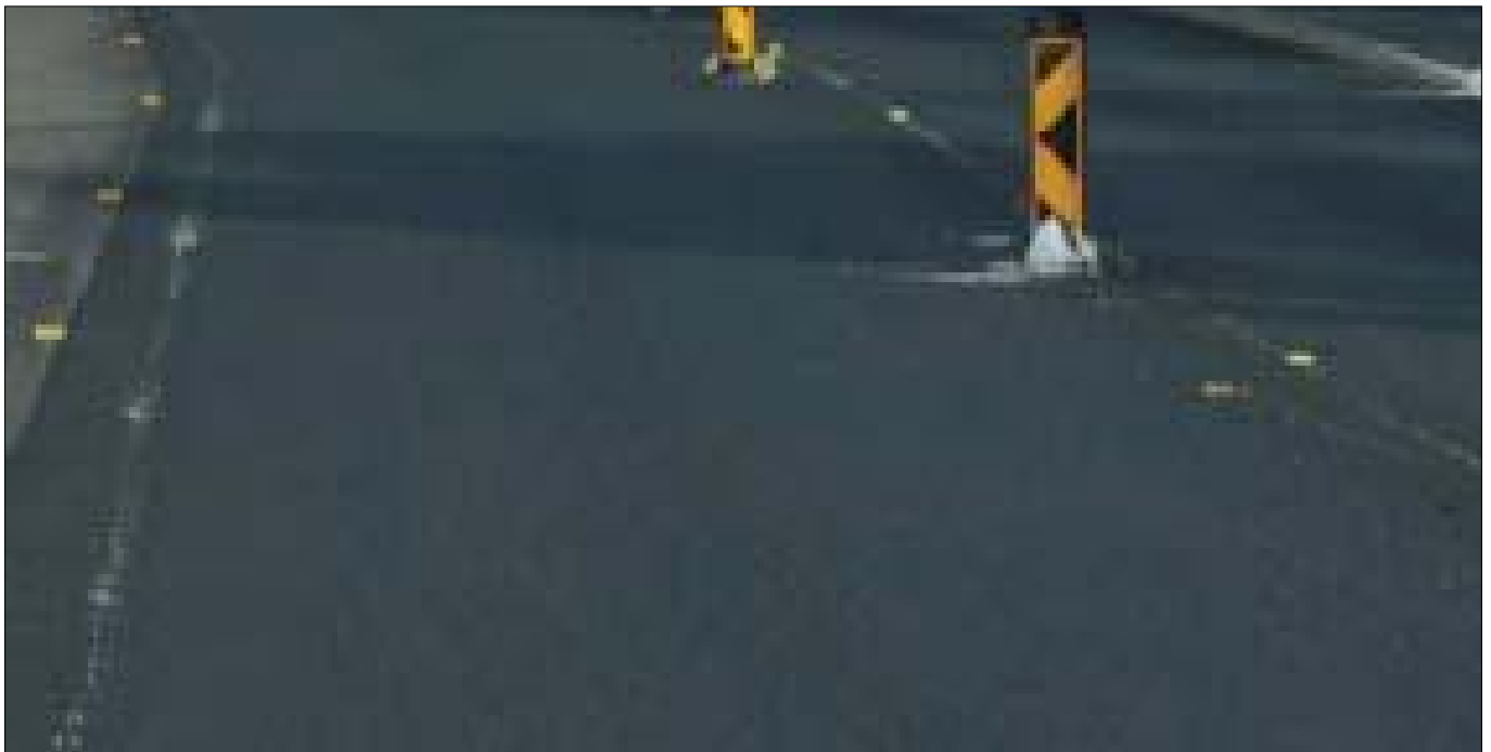
Road Condition – After 4 Months
