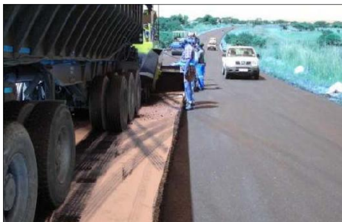
Asphalt Overlay over TechGlass AIC 50
