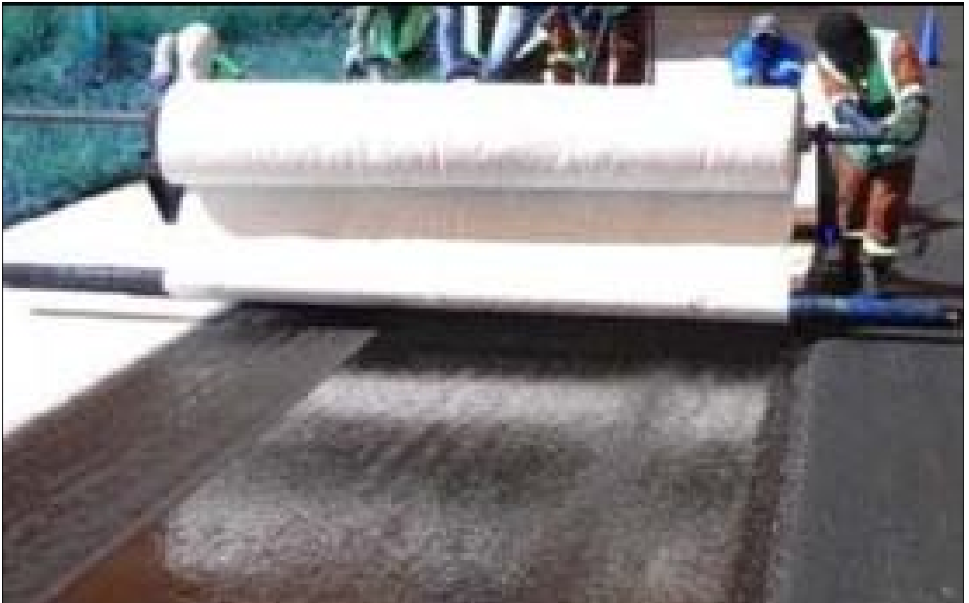
TechGlass AIC 50 over Tack Coat 80/100
