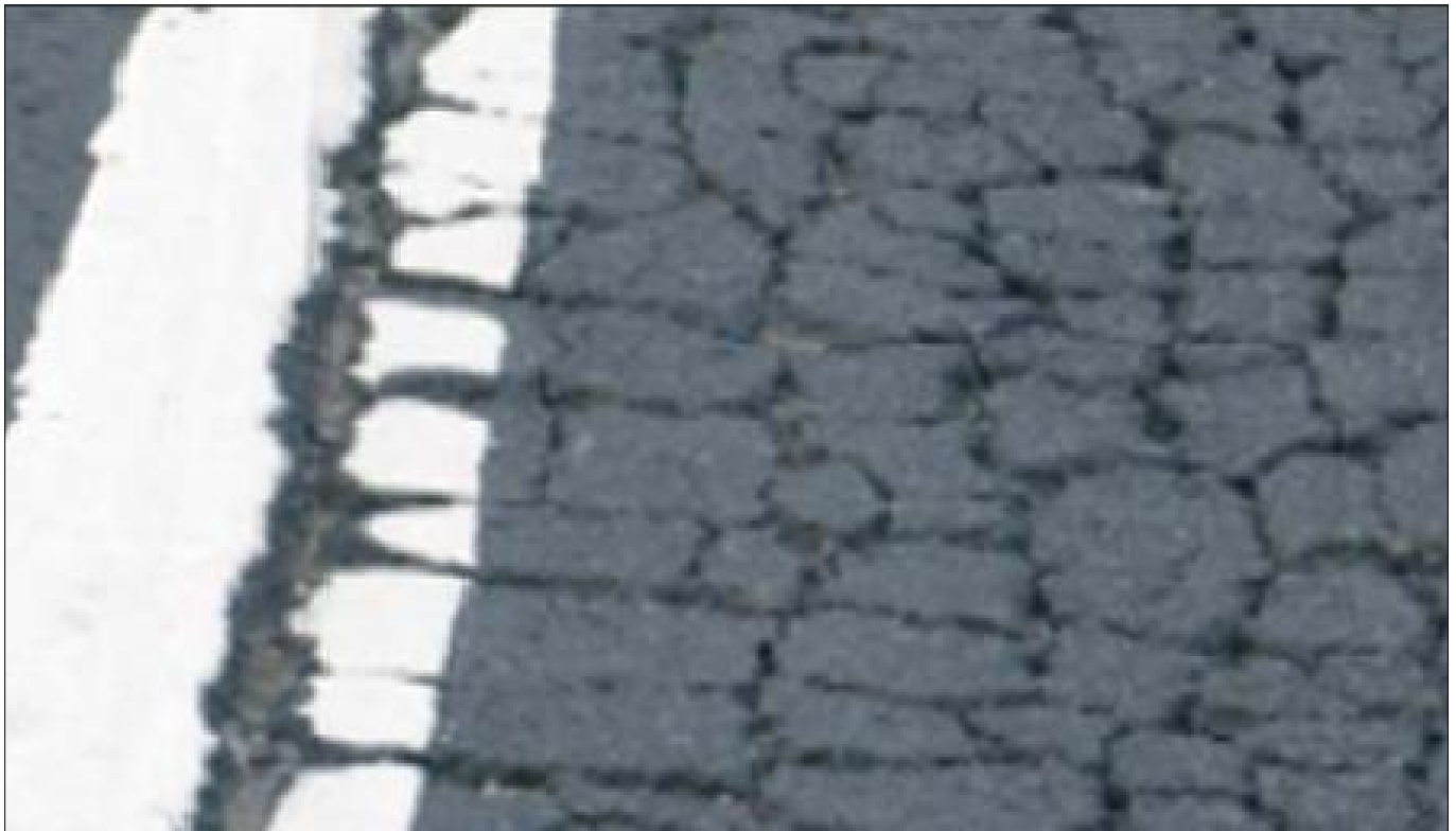
Initial Condition of Road
