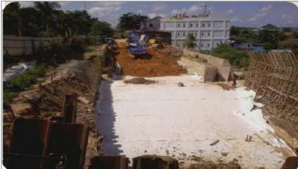
Installation of TGC Geotextile
