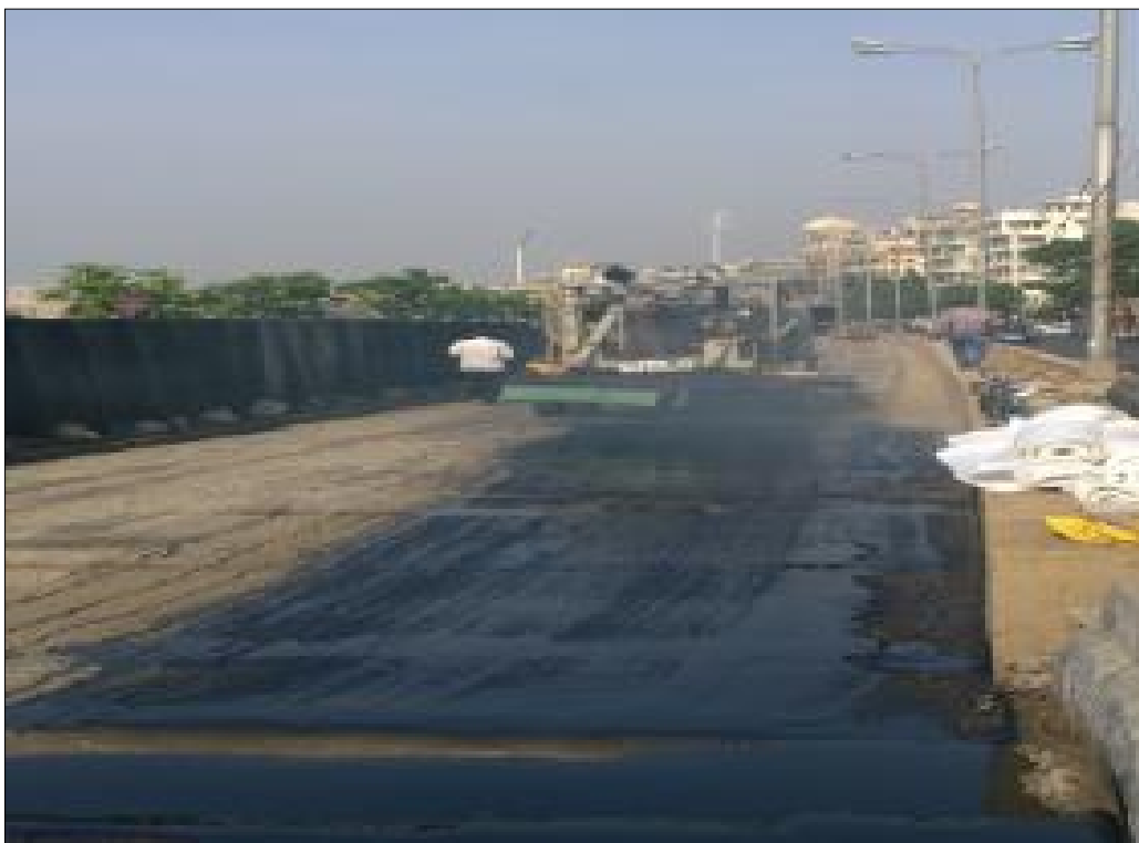
Spraying of Bitumen – Before TechPave
