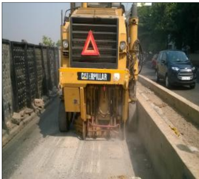
Milling Operation – Before Installation
