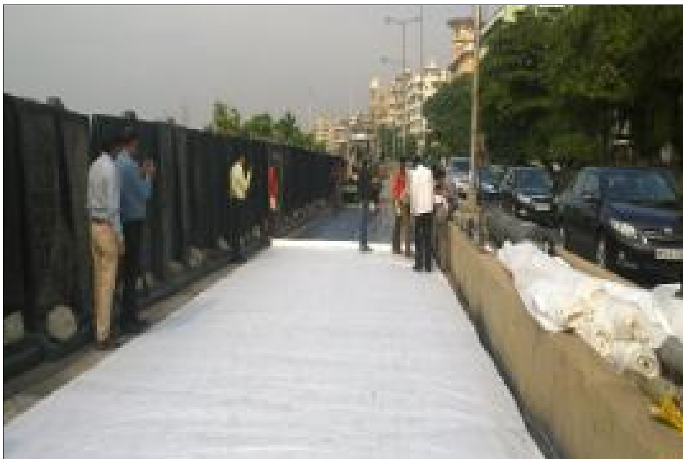
Installation of TechPave
