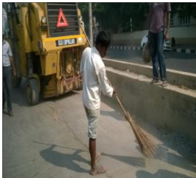
Surface Preparation Before Laying TechPave
