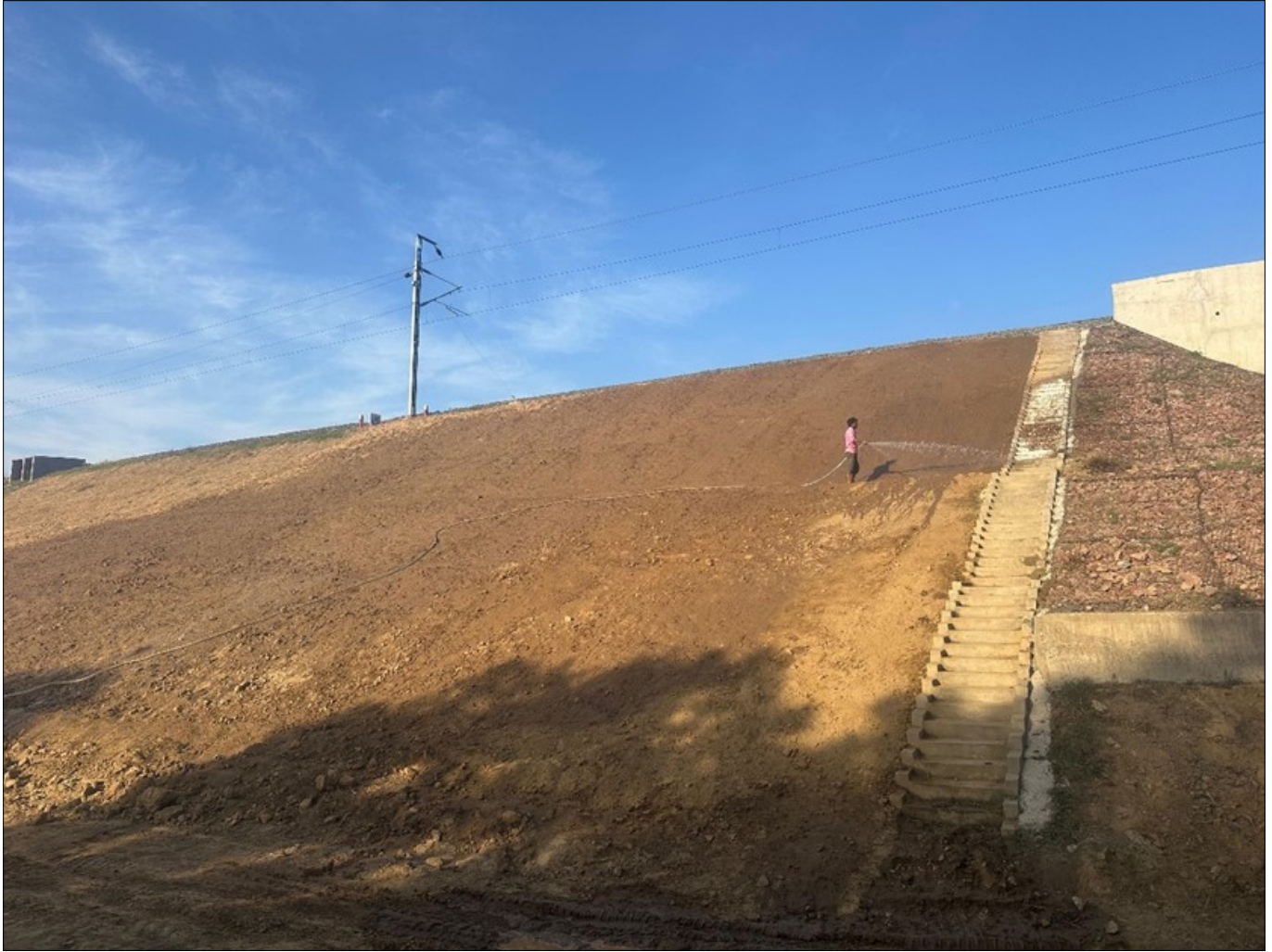
Photo 6 : Slope After Application of Vegetative Soil
