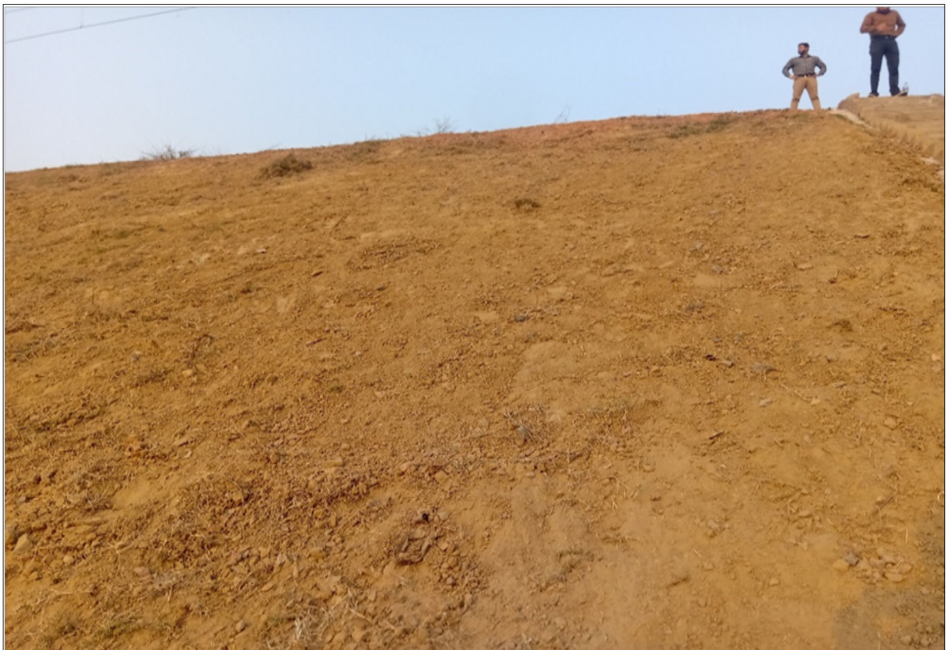
Photo 1 : Preparation of Slope (1V : 2 H)
