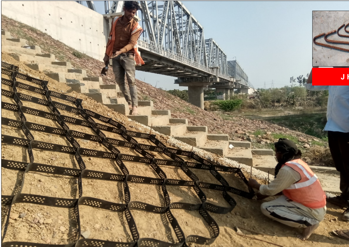
Photo 3 : Anchoring of J Hooks
