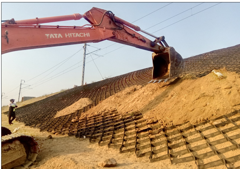
Photo 4 : Placing Vegetative Soil onto the Geocell
