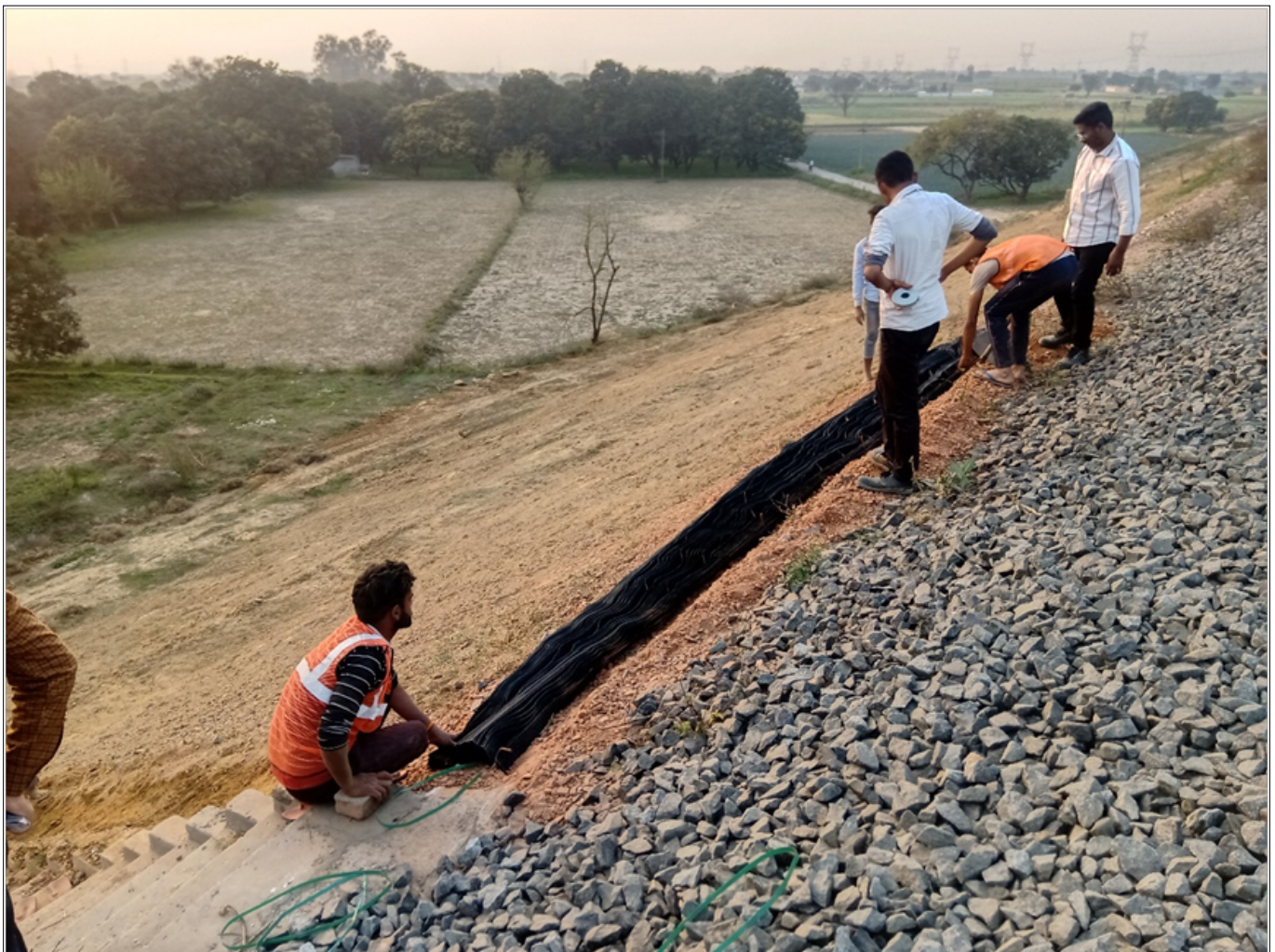
Photo 2 : Spreading of Geocell on Slope Surface
