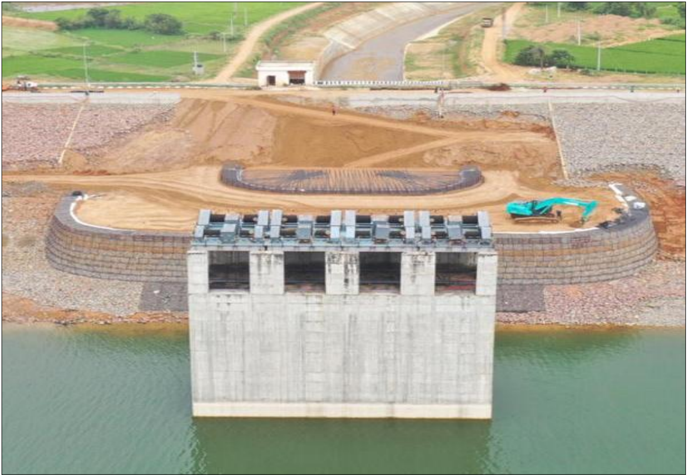
Photo 2 : During Construction - TechStrap Geostrips installation
