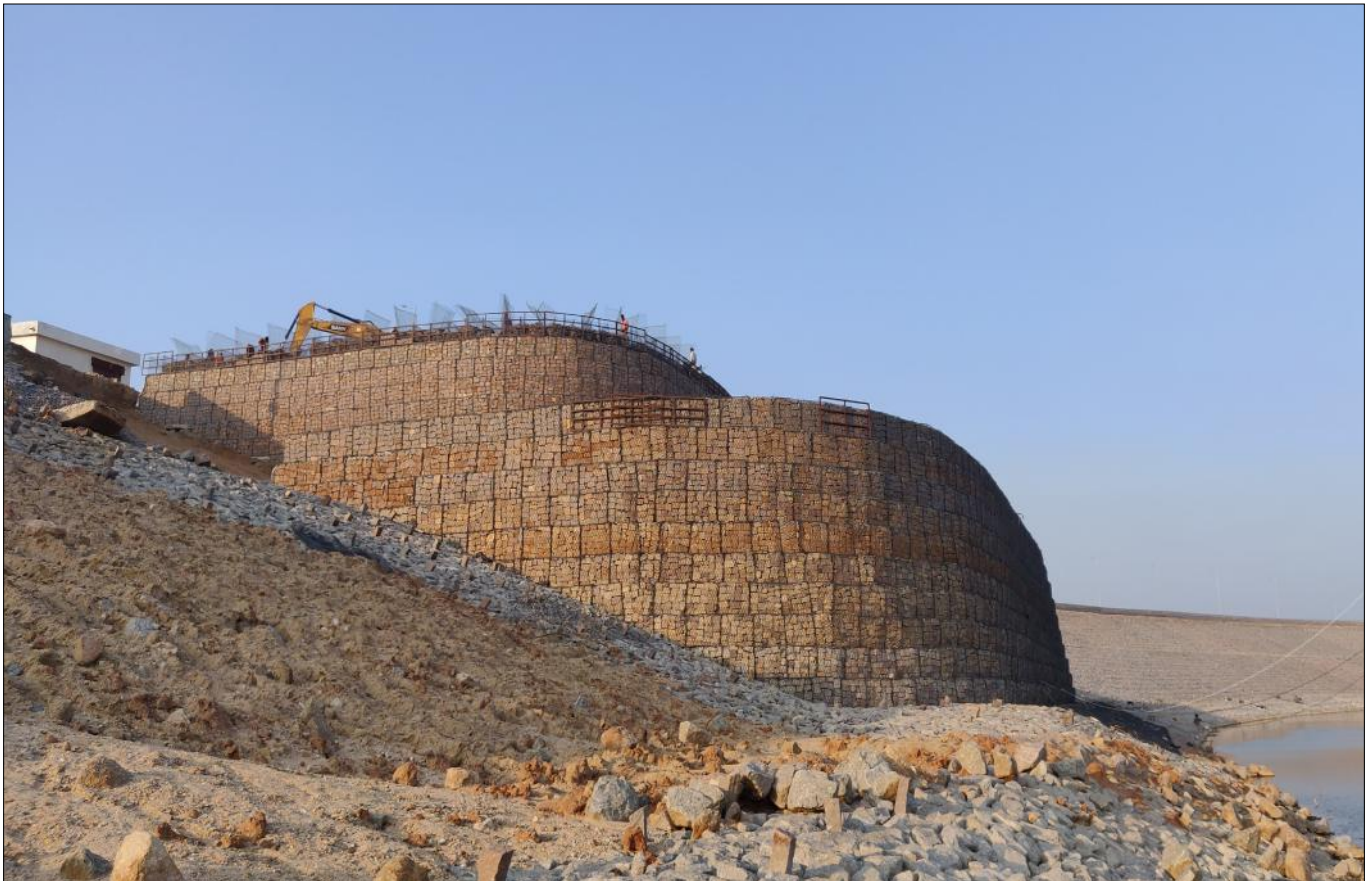
Photo 4 : During Construction - Top Wall
