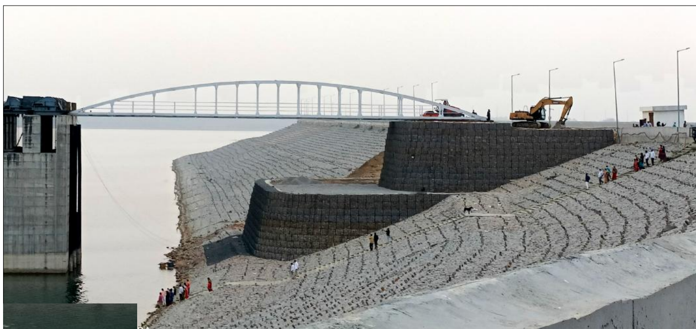
Photo 7 : Photograph of Completed Structure
