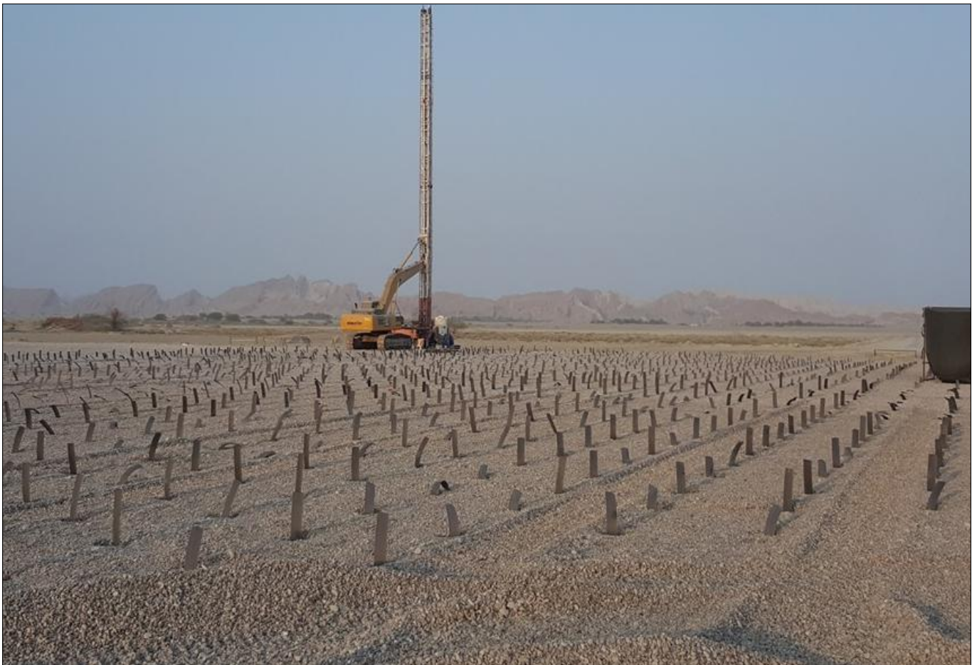
Photo 4 - TechDrain PVD installation is in progress
