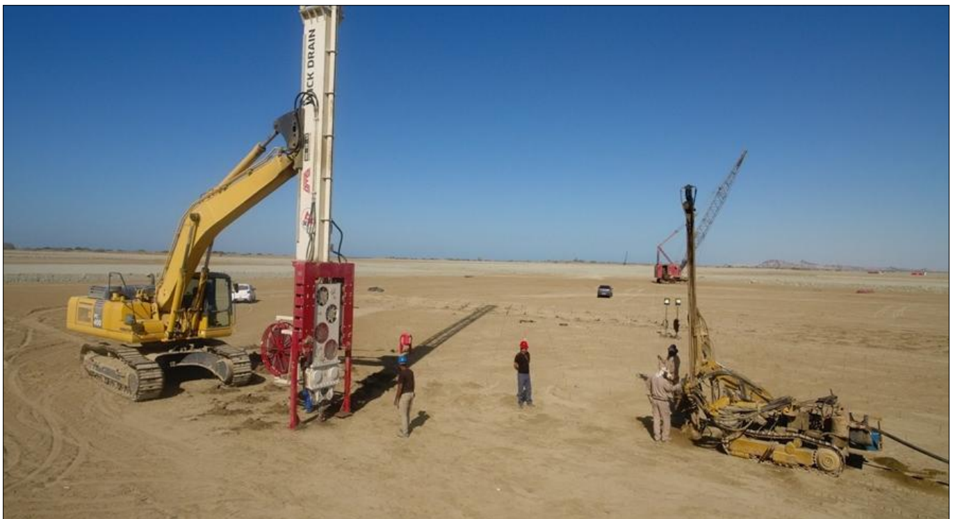
Photo 1 : TechDrain PVD installation starting at site
