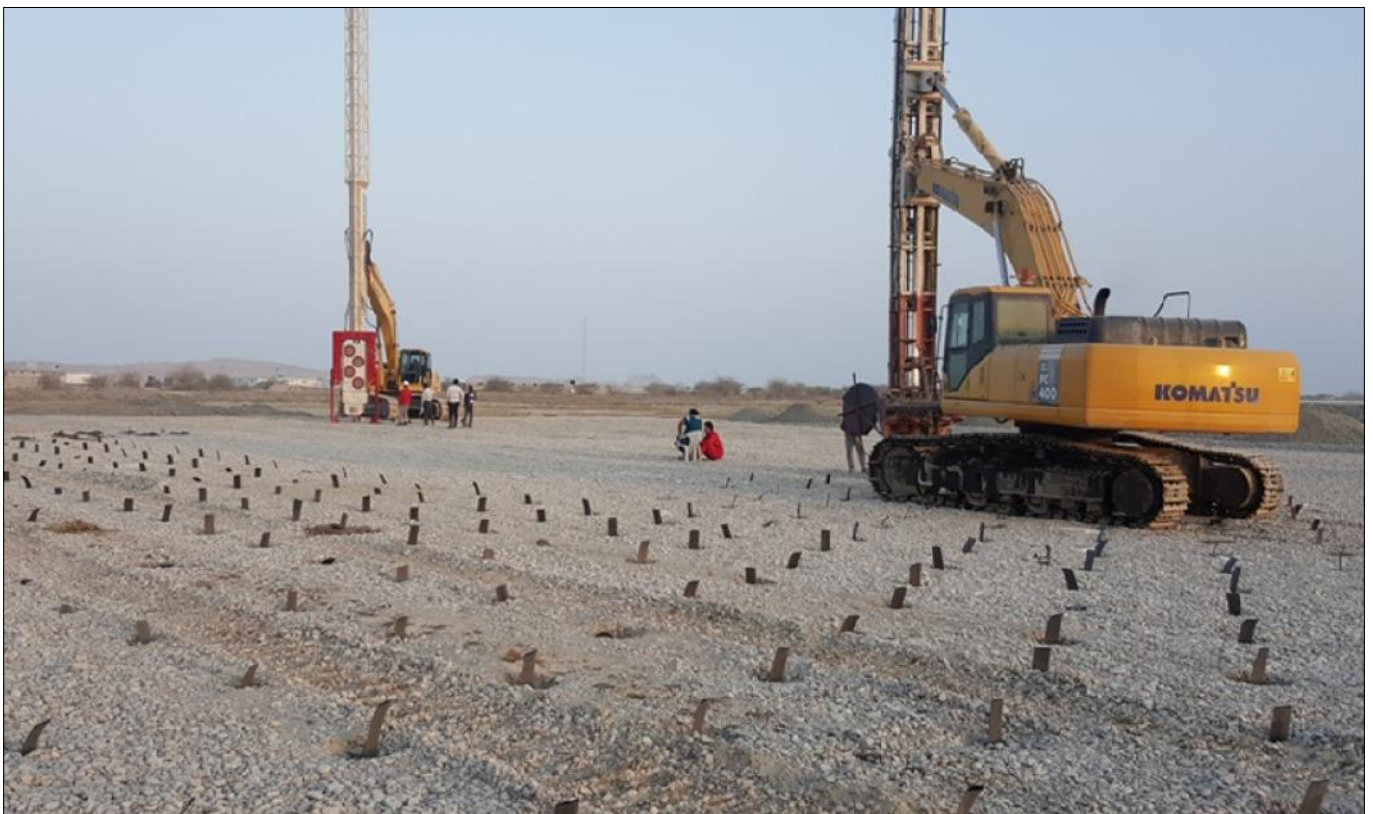
Photo 2&3 - TechDrain PVD installation is in progress
