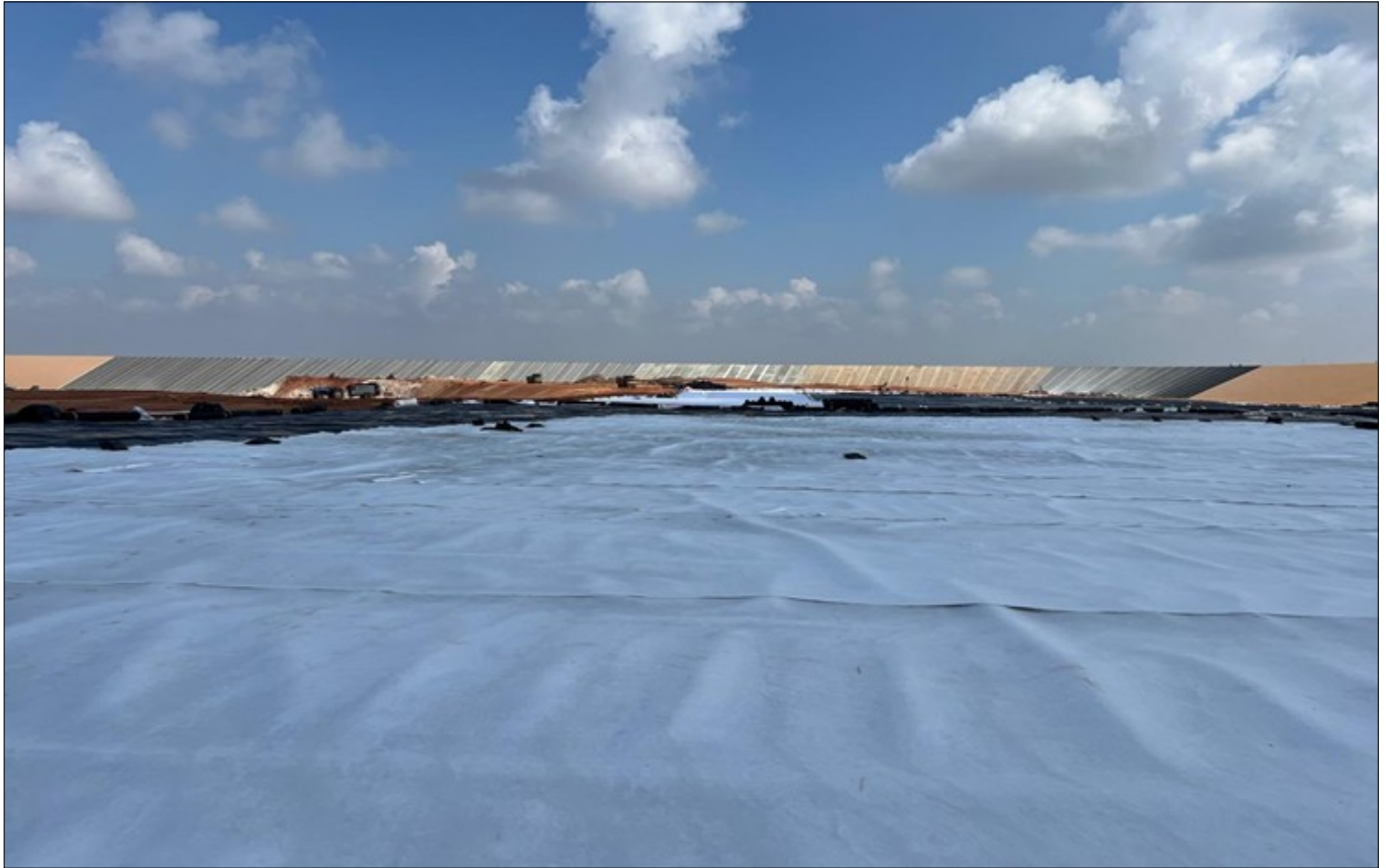
Photo 4 : Installed Geotextile Layer
