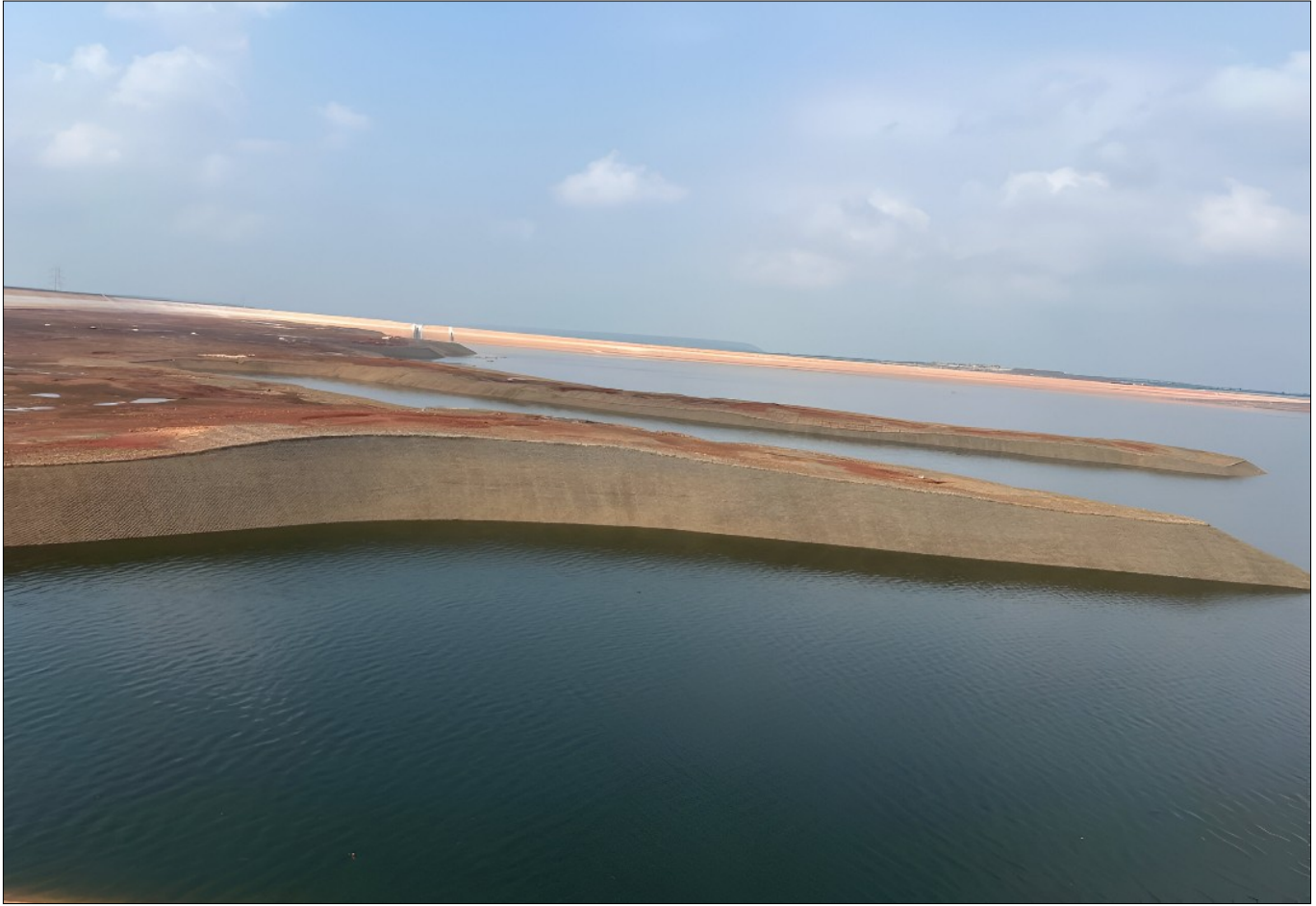
Photo 7 : Completed Reservoir with Advanced Geosynthetic Protection
