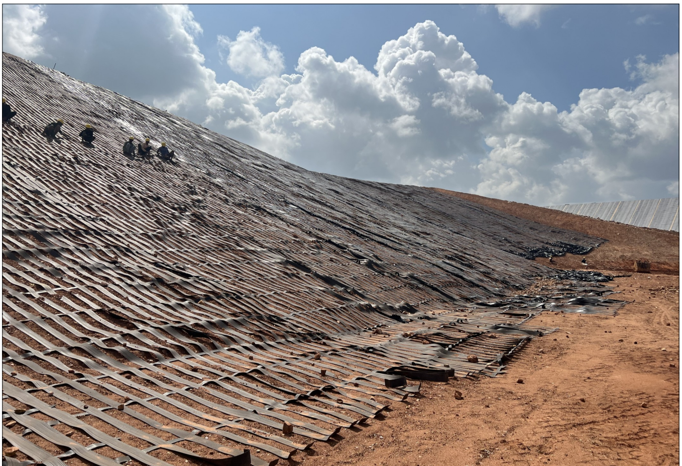
Photo 6 : Installed TechLink TL 350 Geogrid on Slope
