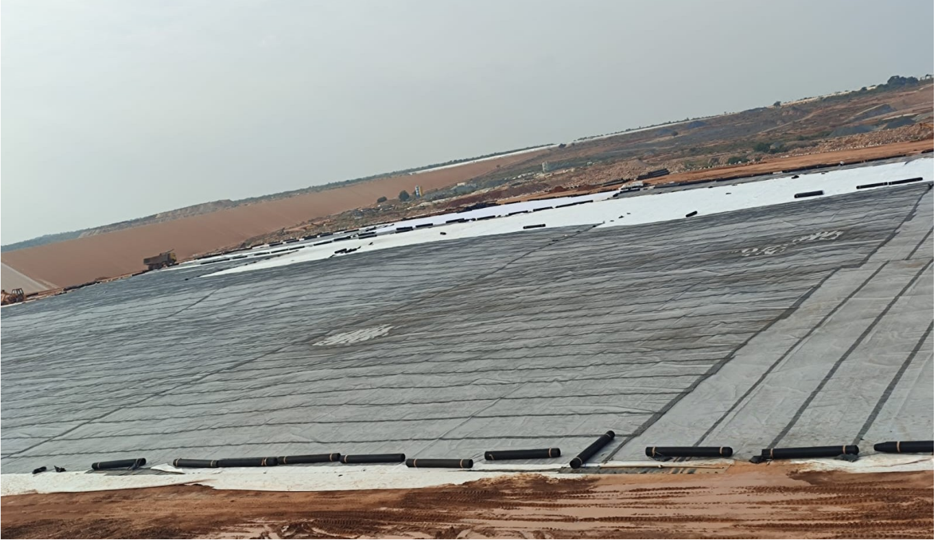
Photo 5 : Installed Geosynthetic Layers
