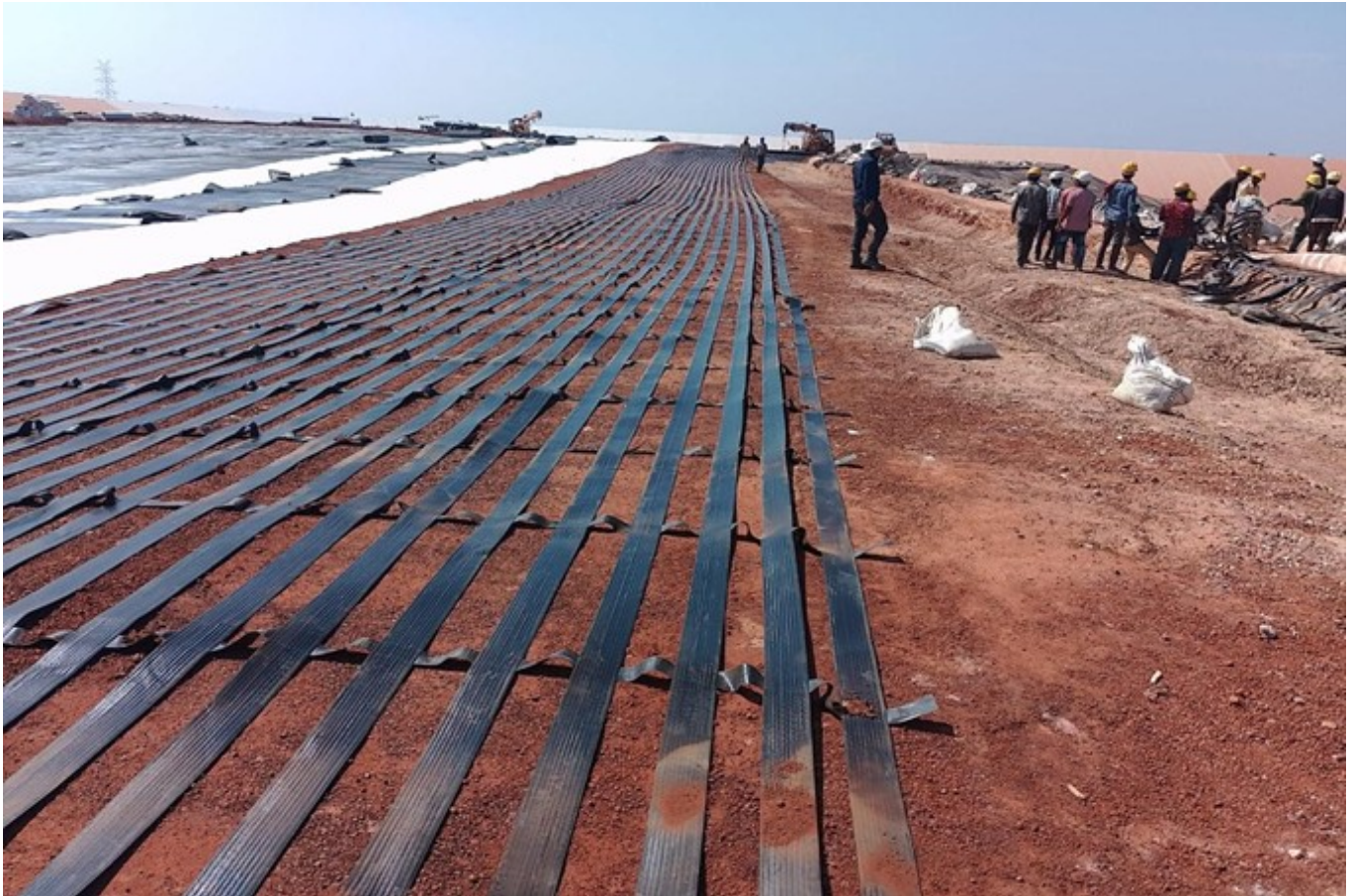
Photo 3 : Installation of TechLink TL 350 Geogrid and TechGeoPN 70 Geotextile on Insitu Strata
