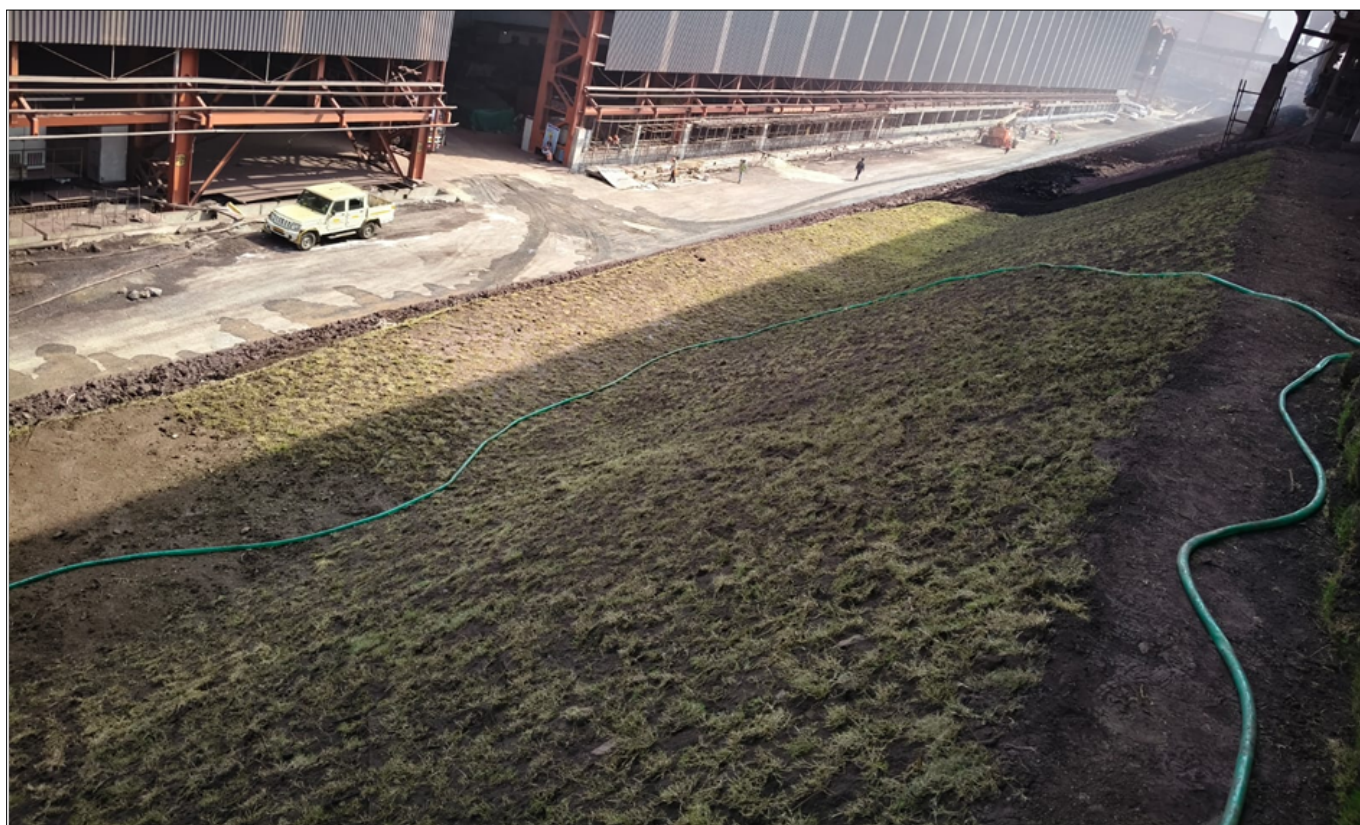
Photo 6 : Sustainable Slope Protection, Greenery Begins
