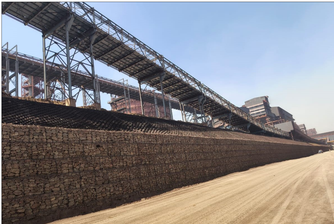
Photo 5 : Installation of Geocell above Gabion Wall
