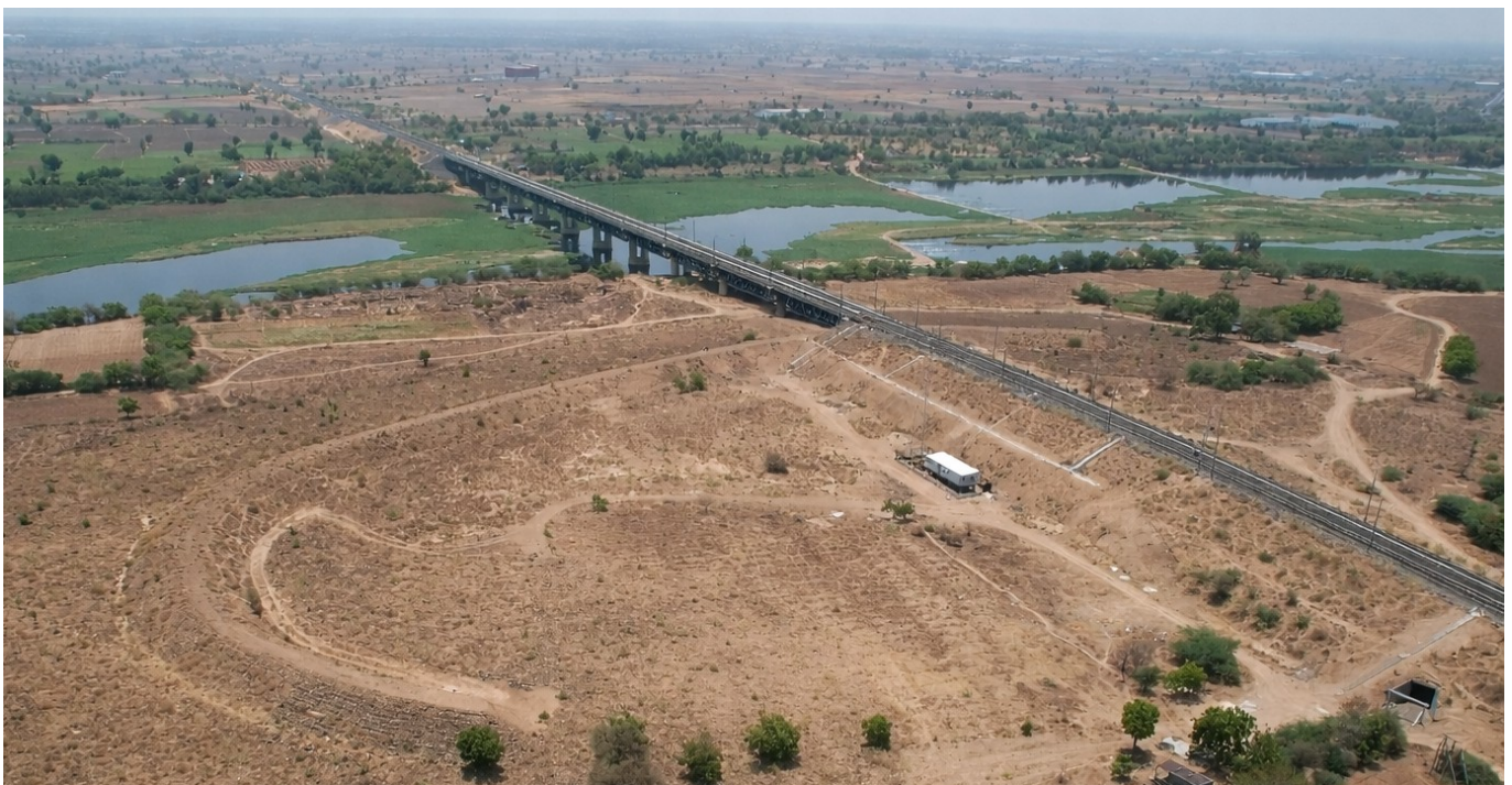
Photo 1 : Site Condition Before Protection Works
