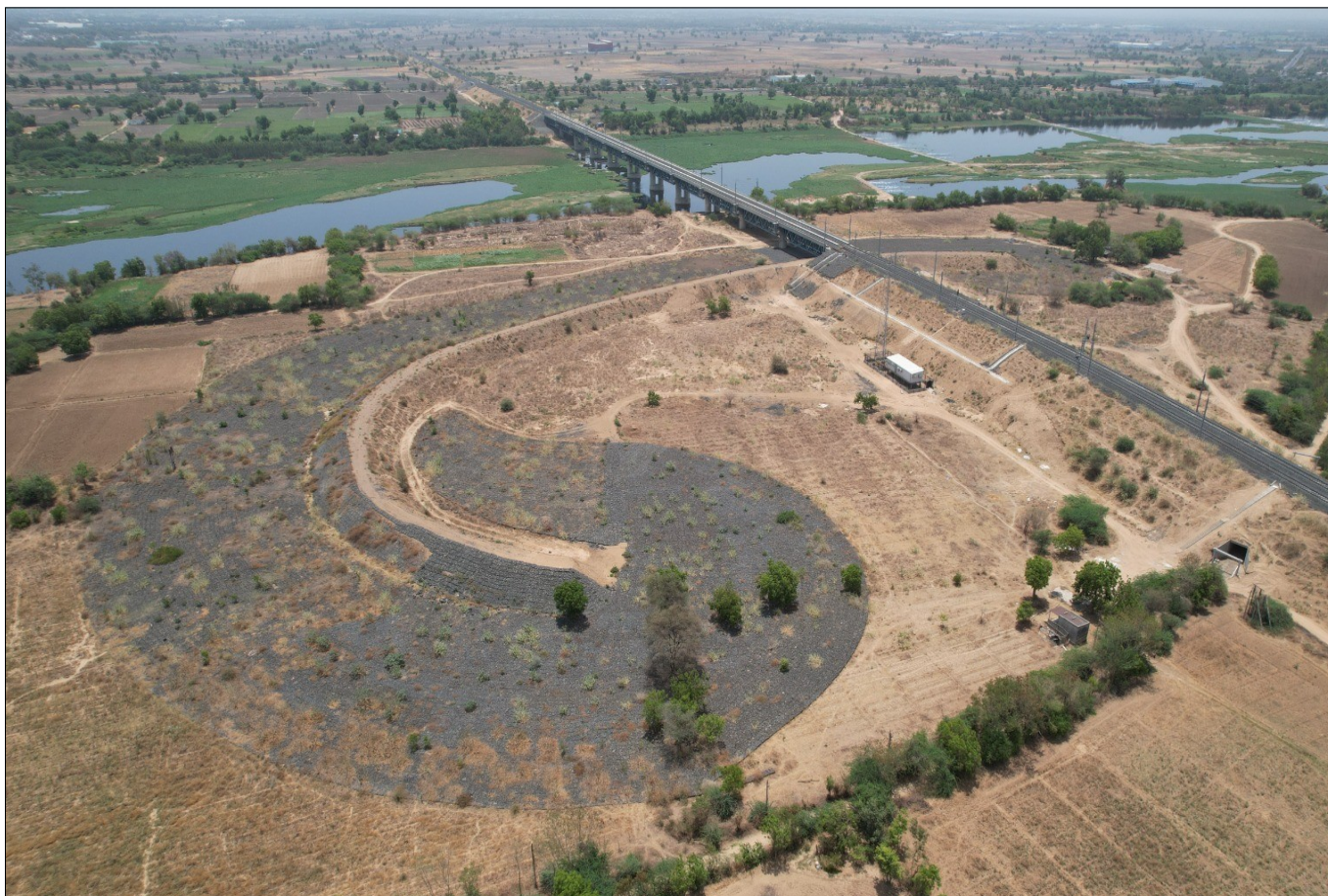
Photo 5 : Gabion Solutions Blending Seamlessly with the River Landscape
