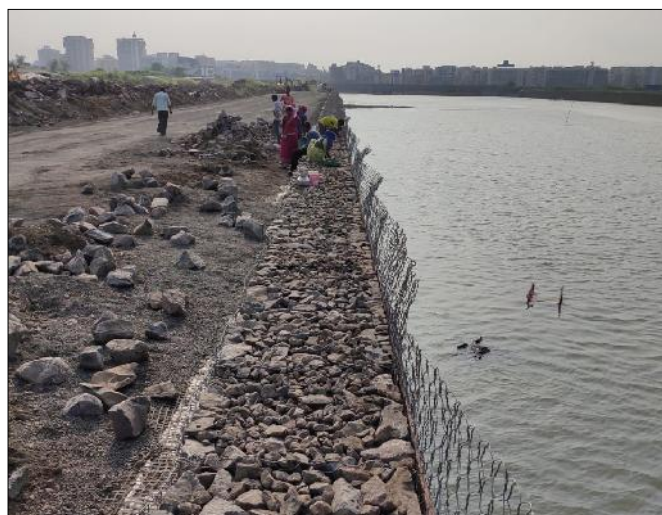
Figure 8 & 9 : Installation, Filling of Gabion mesh with stone in progress
