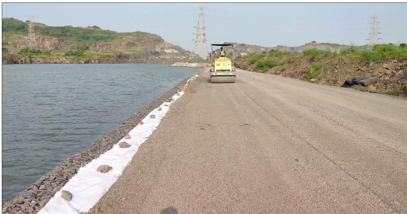
Figure 7 : Compaction behind the wall in progress
