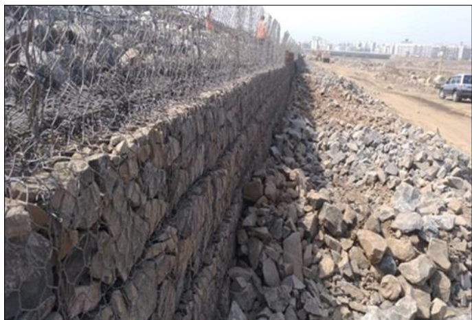
Figure 5 & 6 : Installation, Filling of Gabion mesh with stone in progress
