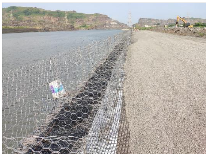
Figure 8 & 9 : Installation, Filling of Gabion mesh with stone in progress
