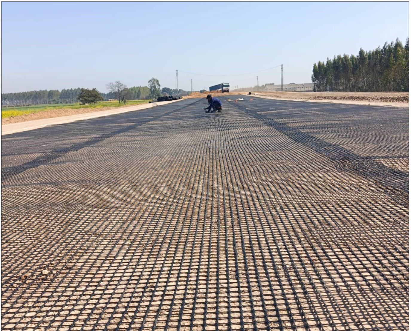
Photo 4 : Overlapping of Geogrid at the edge and fixing it with U bar
