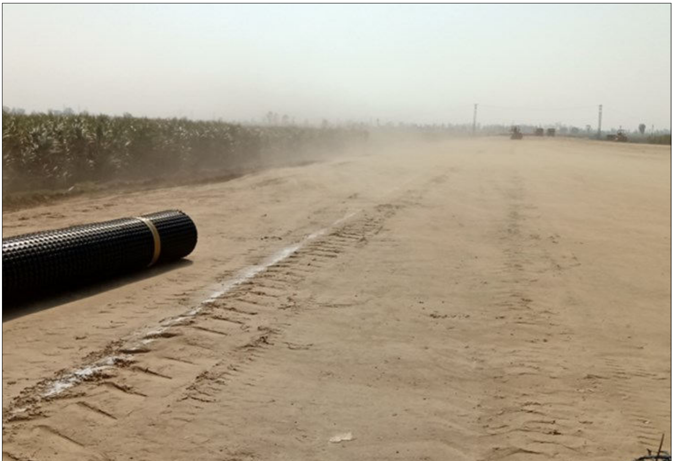
Photo 1 : Prepared Subgrade Layer as per the Design
