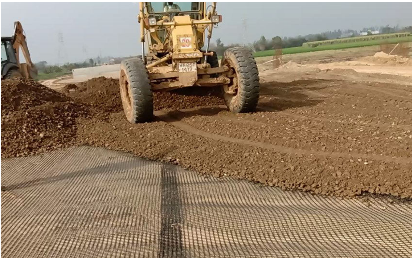
Photo 5 : Spreading of GSB Material over the Subgrade
