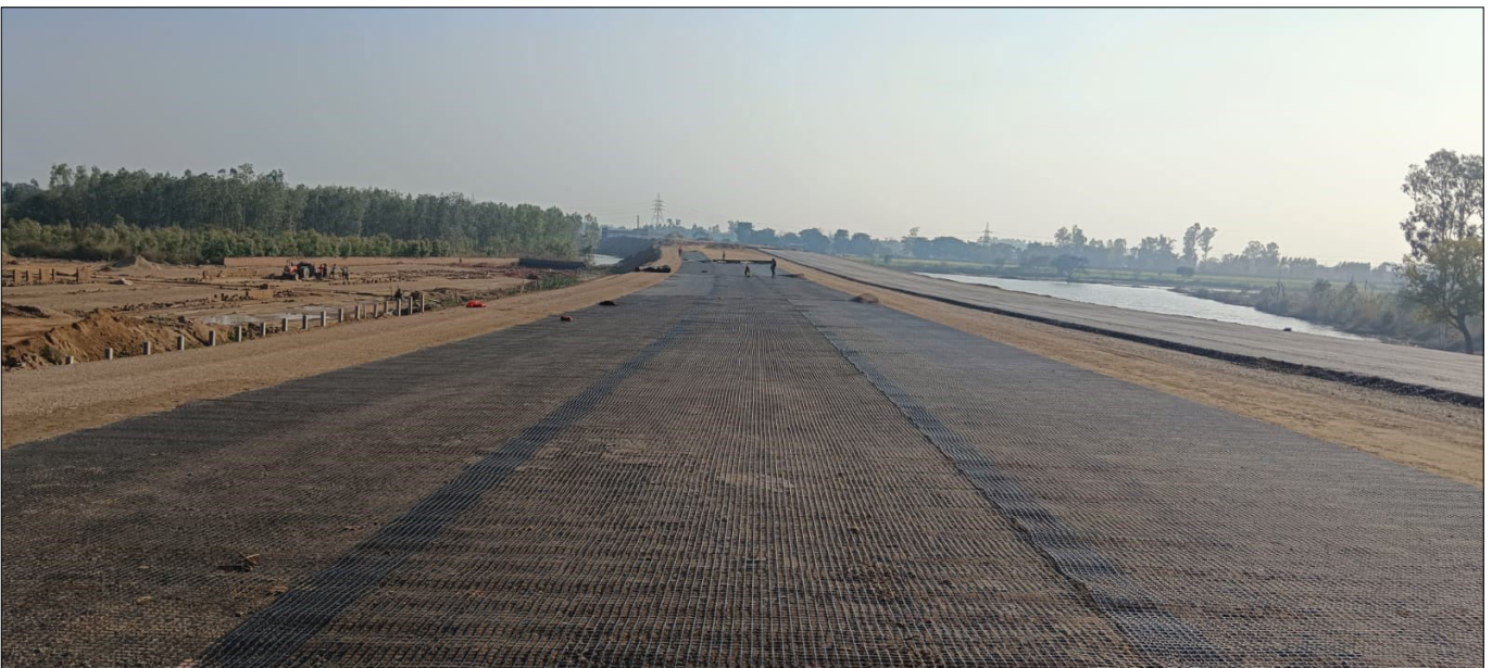
Photo 2 & 3 : Laying of Geogrid on the Subgrade
