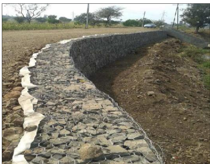
Gabion Retaining Wall
