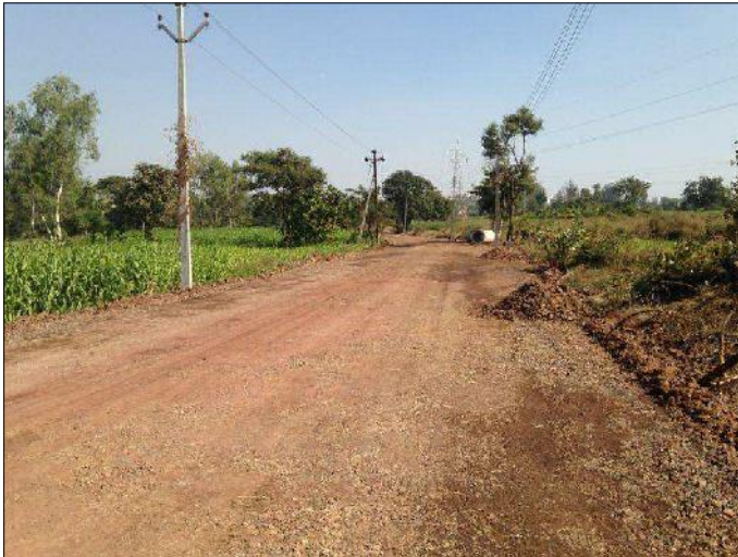
Earthwork after Scarifying Distressed
