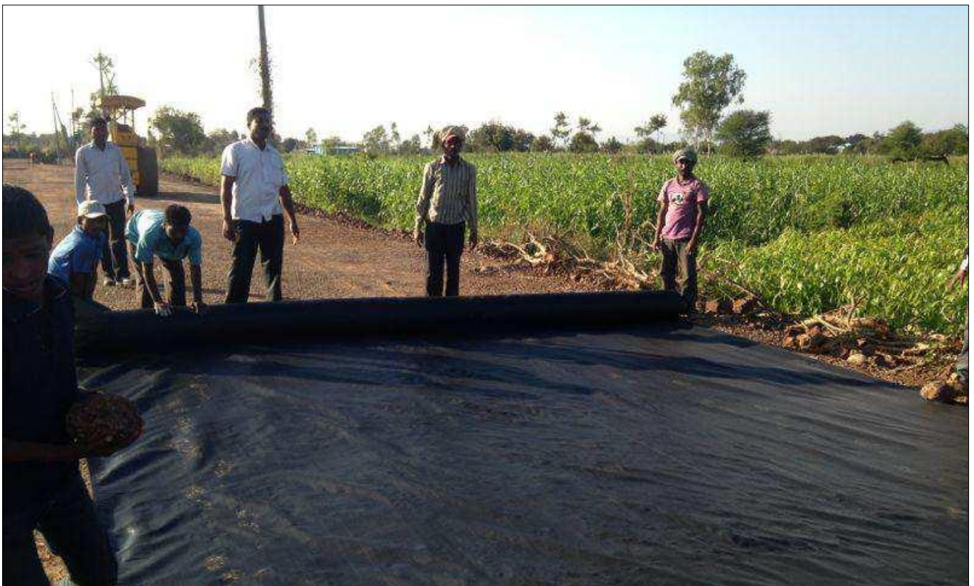
Laying of TFI-5300 Type-I
