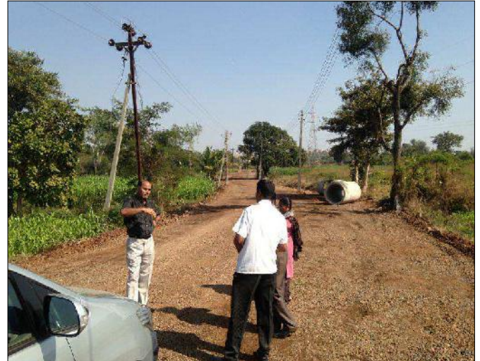
Checking of Subgrade – Exe. Engineer
