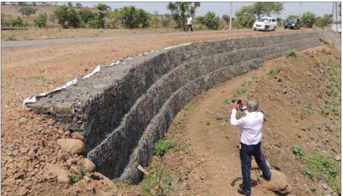
Gabion Retaining Wall
