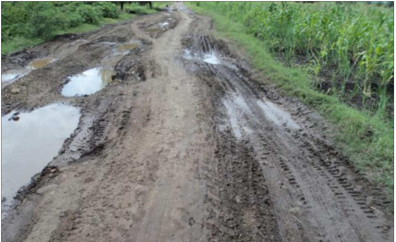
Original Site condition - In monsoon
