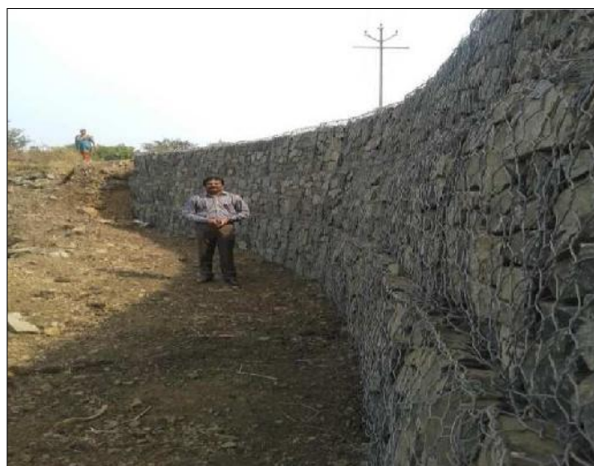
Construction of Gabion Wall
