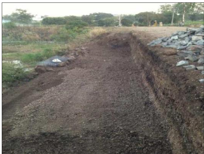
Excavation for Gabion Retaining Wall
