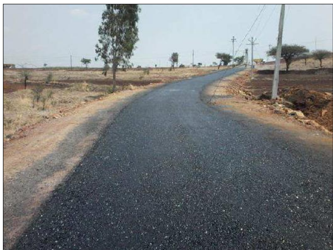
Laying of Seal-Coat
