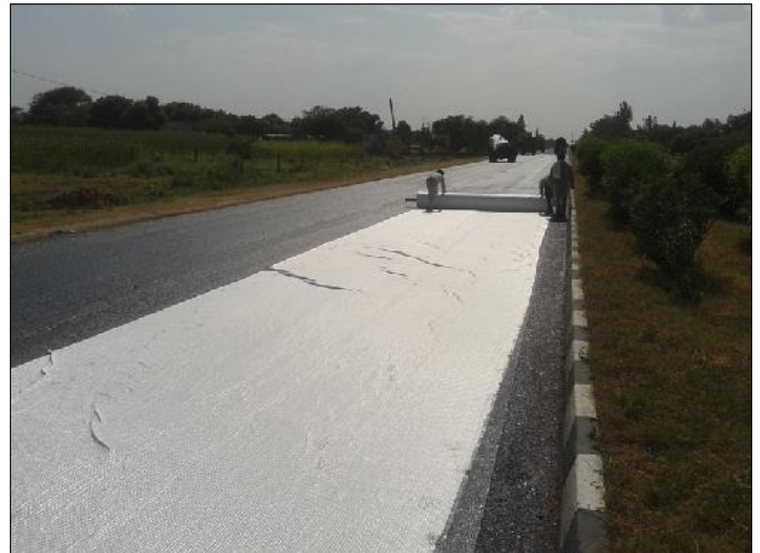
Laying of Geotextile
