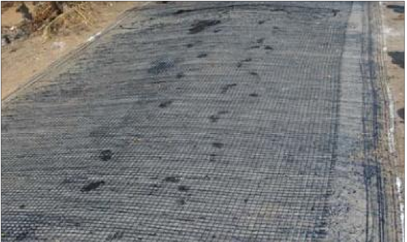
Laying of TechGlass 50
