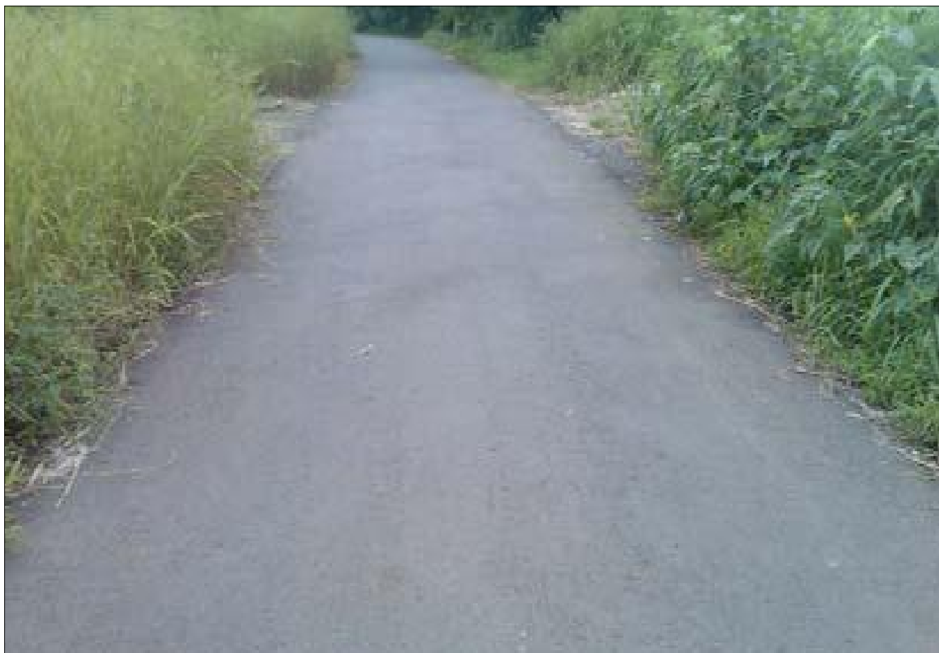
Road Condition after 12 Months (Including Monsoon)
