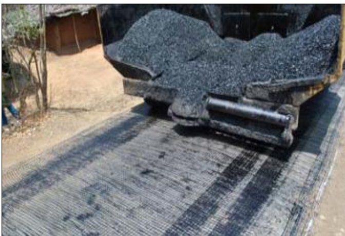
Over lay being laid over the TechGlass
