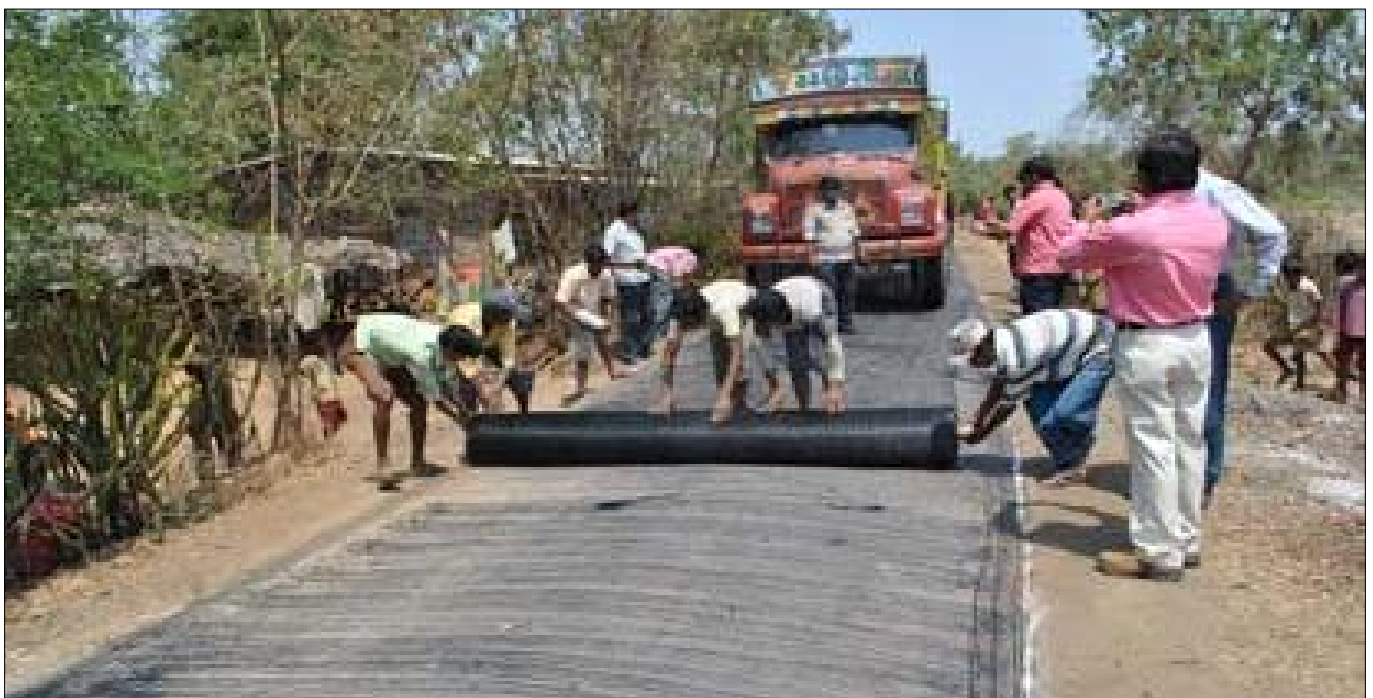
Unrolling of TechGlass 50 at the site
