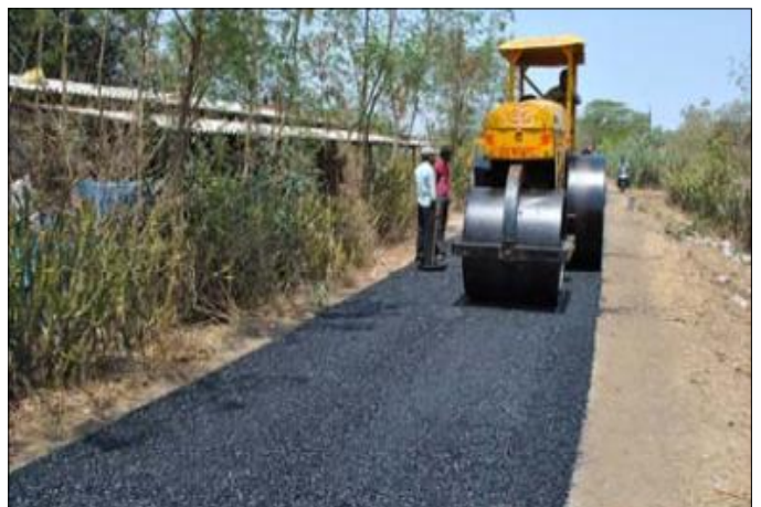
Compaction of Over Lay
