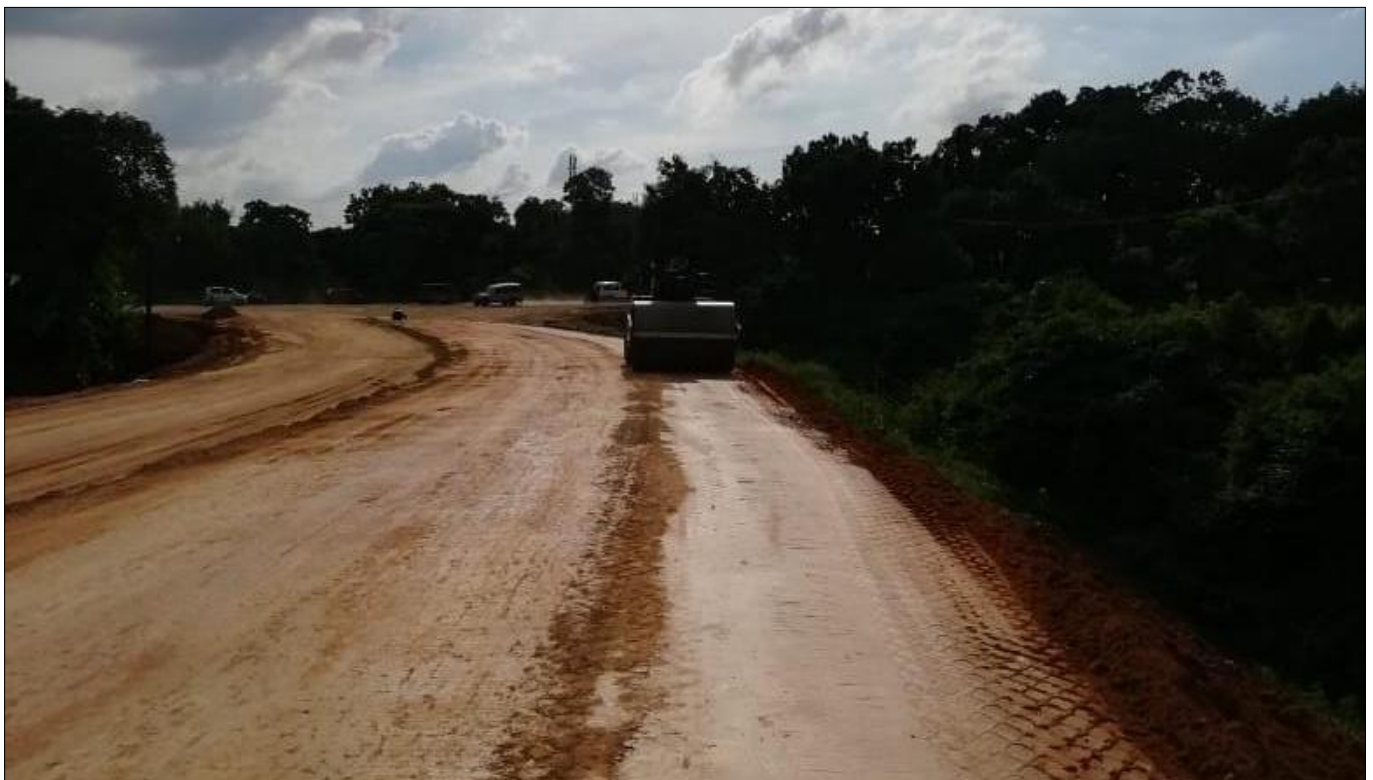
Fig 1 : Preparation of subgrade before laying granular layers.
