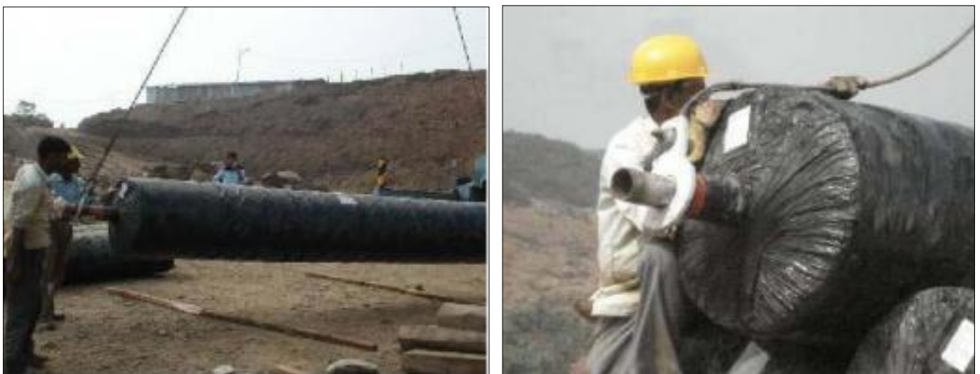
Figure 3 : Handling of Geosynthetic Rolls
