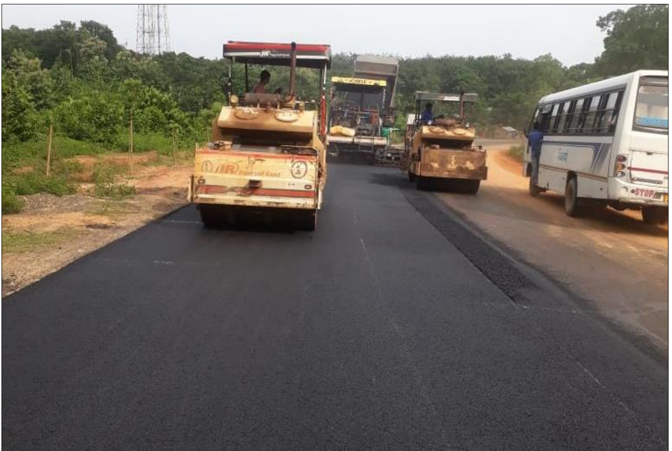
Fig 7 : Laying of Bituminous layers
