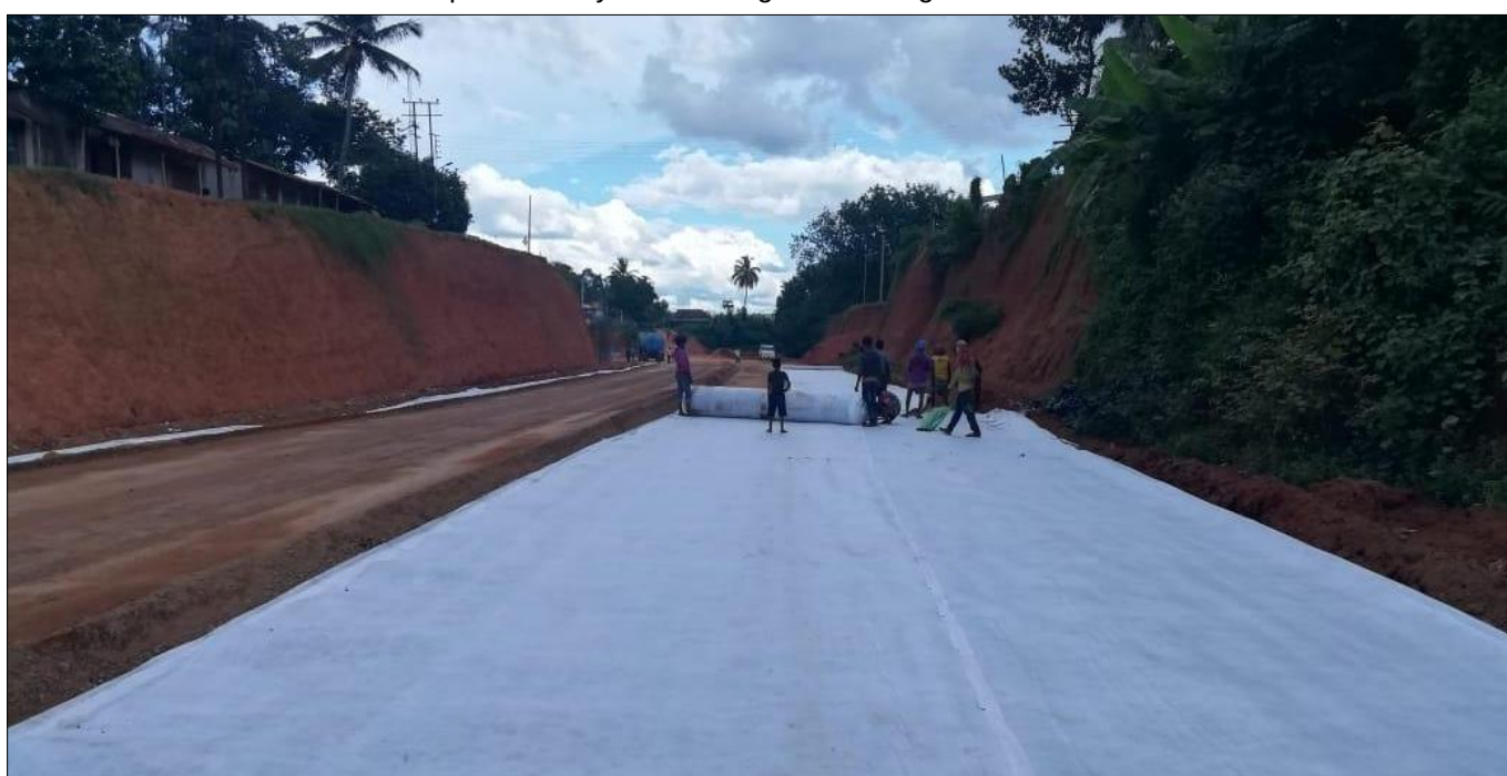
Fig 5 : Unrolling of TechDrain Drainage Composite on the Compacted GSB Layer
