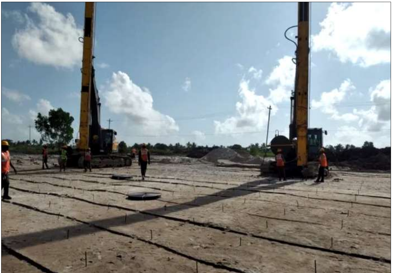
Photo 4 : Installation of PSC working piles below structure
