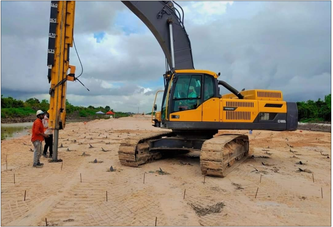
Photo 5 : Installation of PVD
