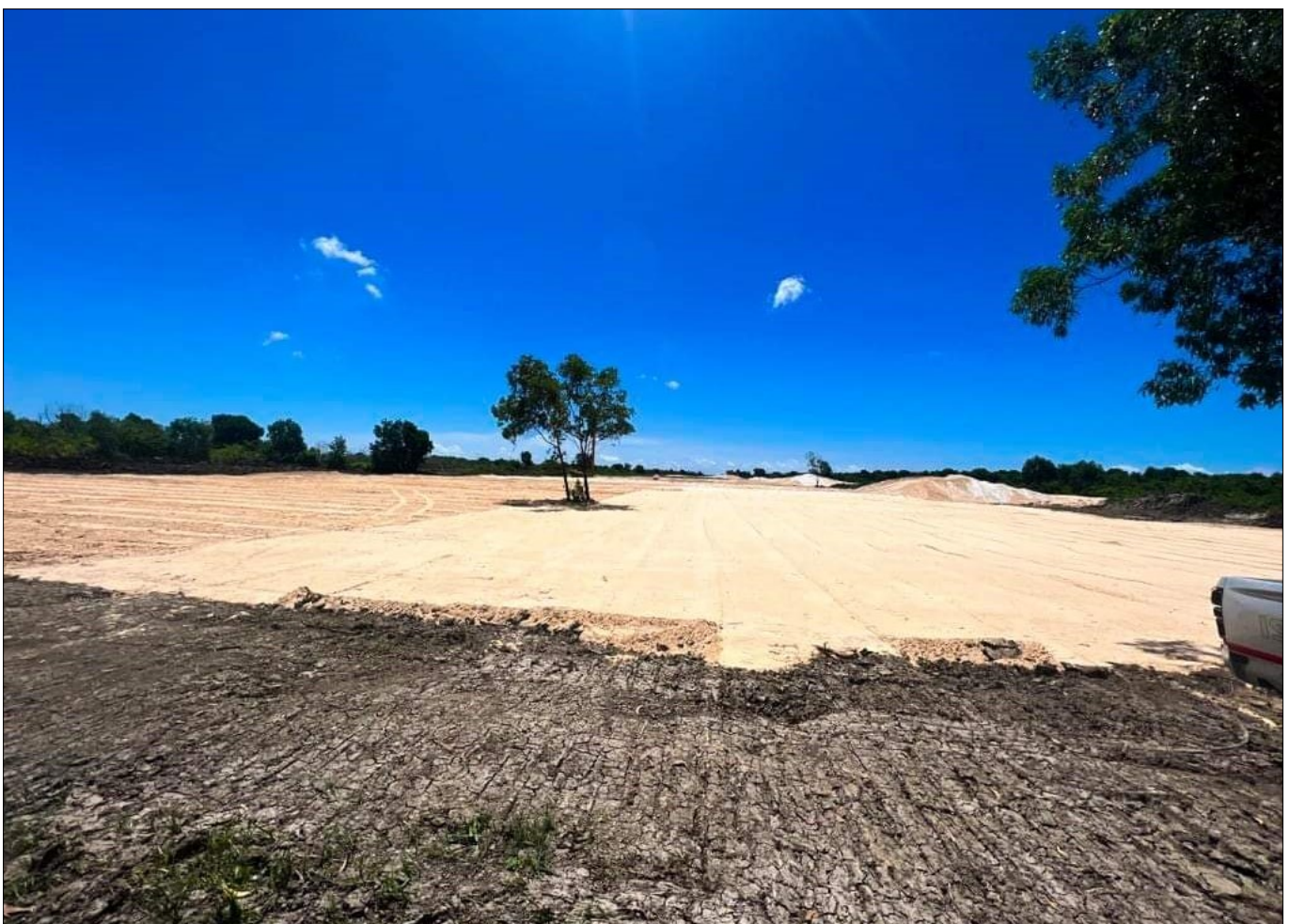
Photo 3 : - Filling of white sand for PVD base layer
