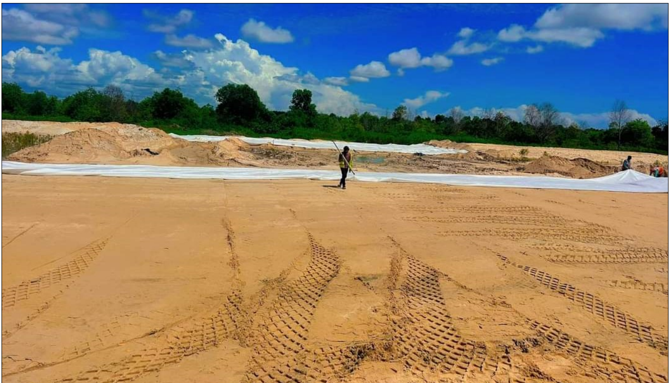
Photo 1 : Laying of Geotextile fabric on granular sand blanket layer
