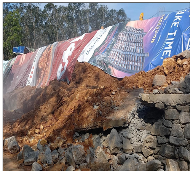
Photo 1 & 2 : View of the Collapsed Existing Stone Masonry Retaining Wall
