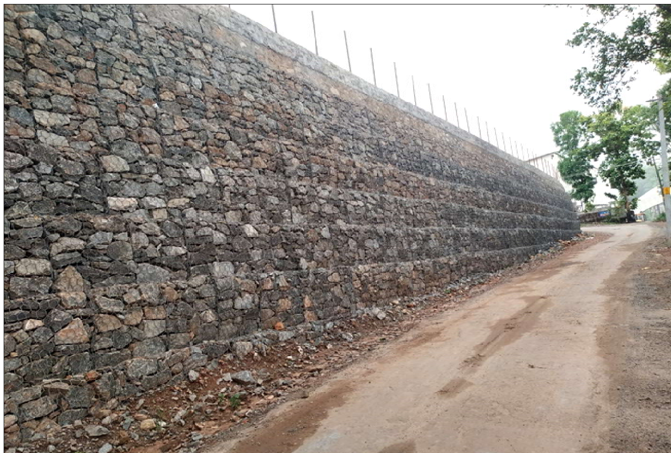
Photo 3 : After Completion of Project
