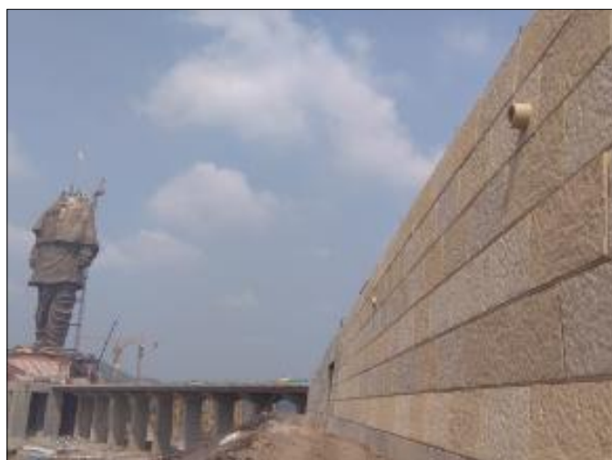
Finished view of RS Wall Panels
