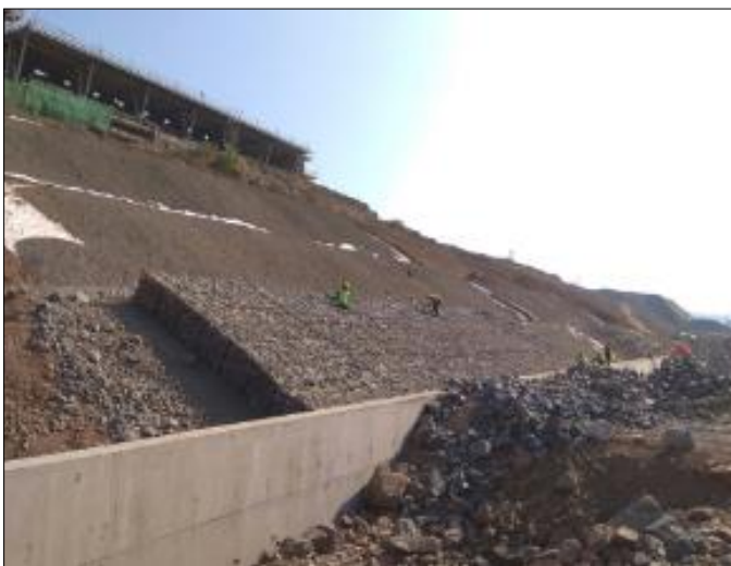
TechFab Metal Gabion Mattress laying in progress
