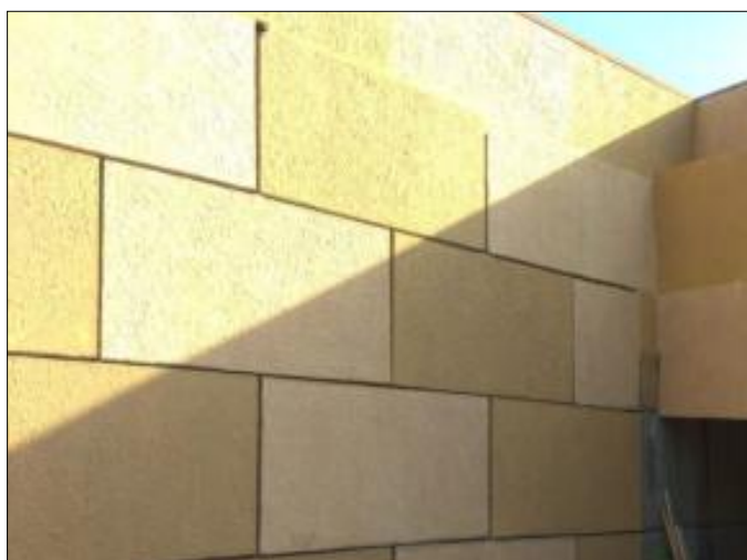
Finished view of RS Wall Panels
