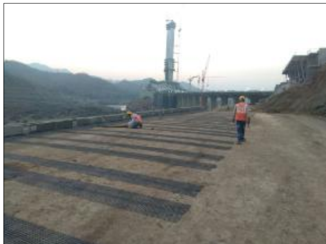
Geogrid Laying for RS Walls
