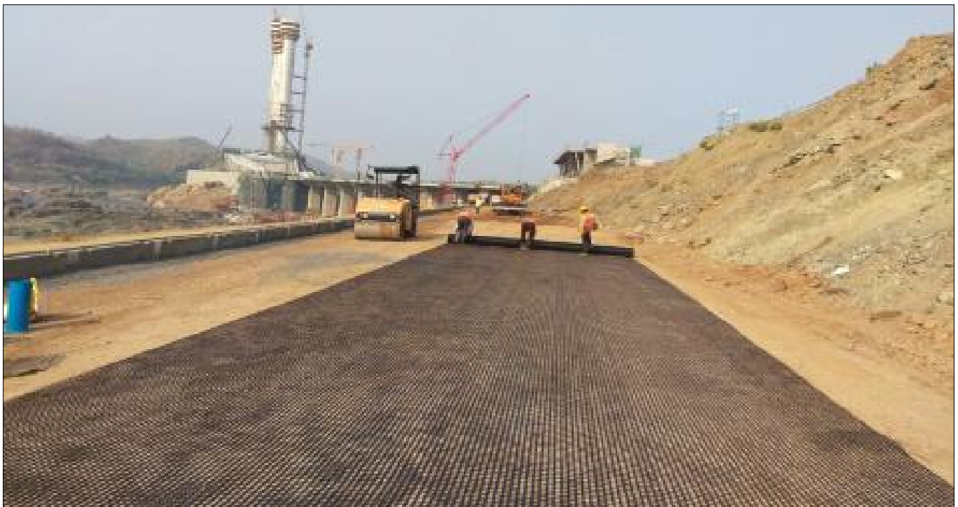
Laying of TechGrid Geogrid in Progress
