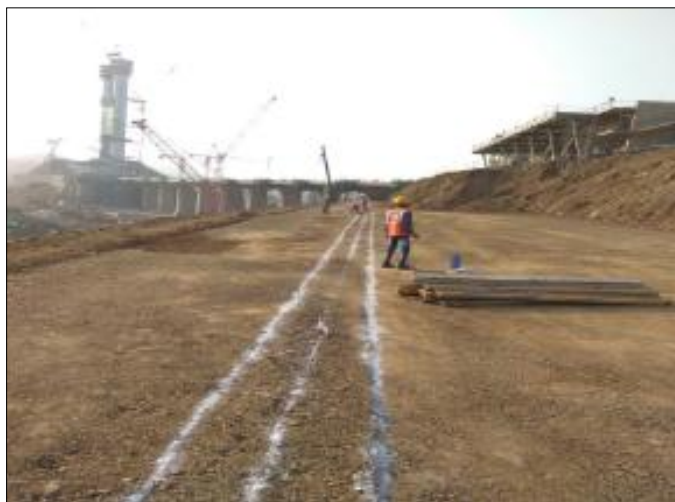
Marking in progress for RS Walls
