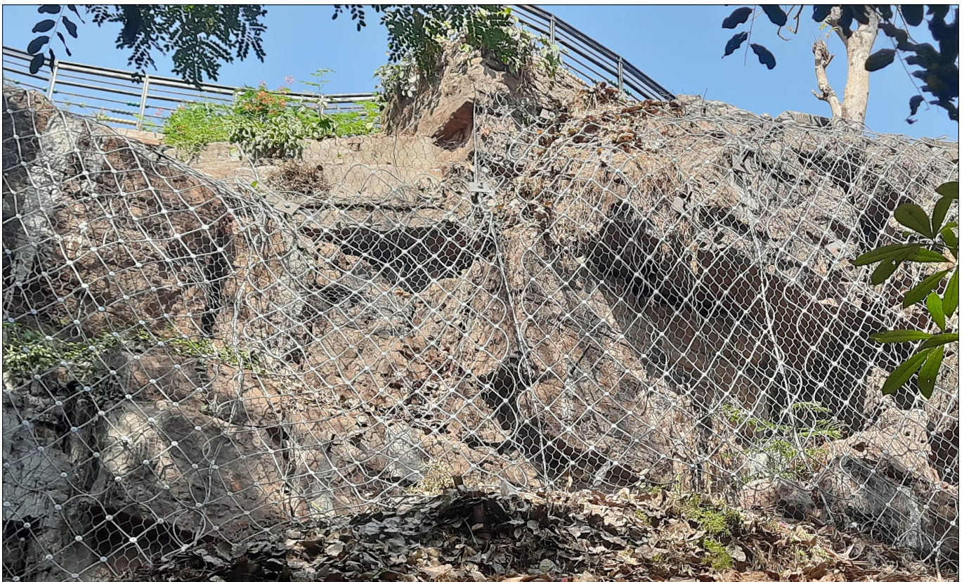
Installation works in progress
