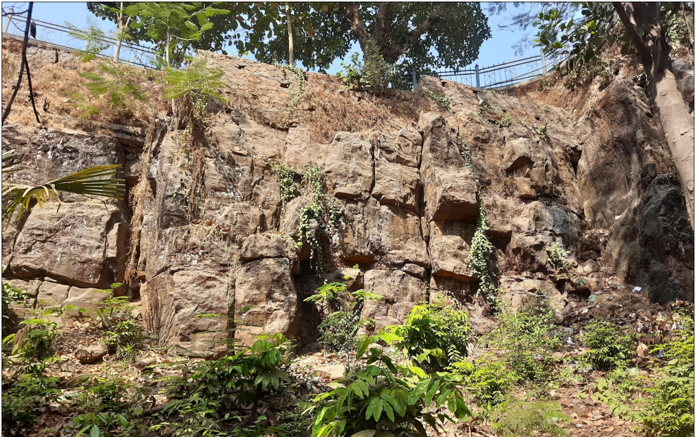
Slope Before Protection
