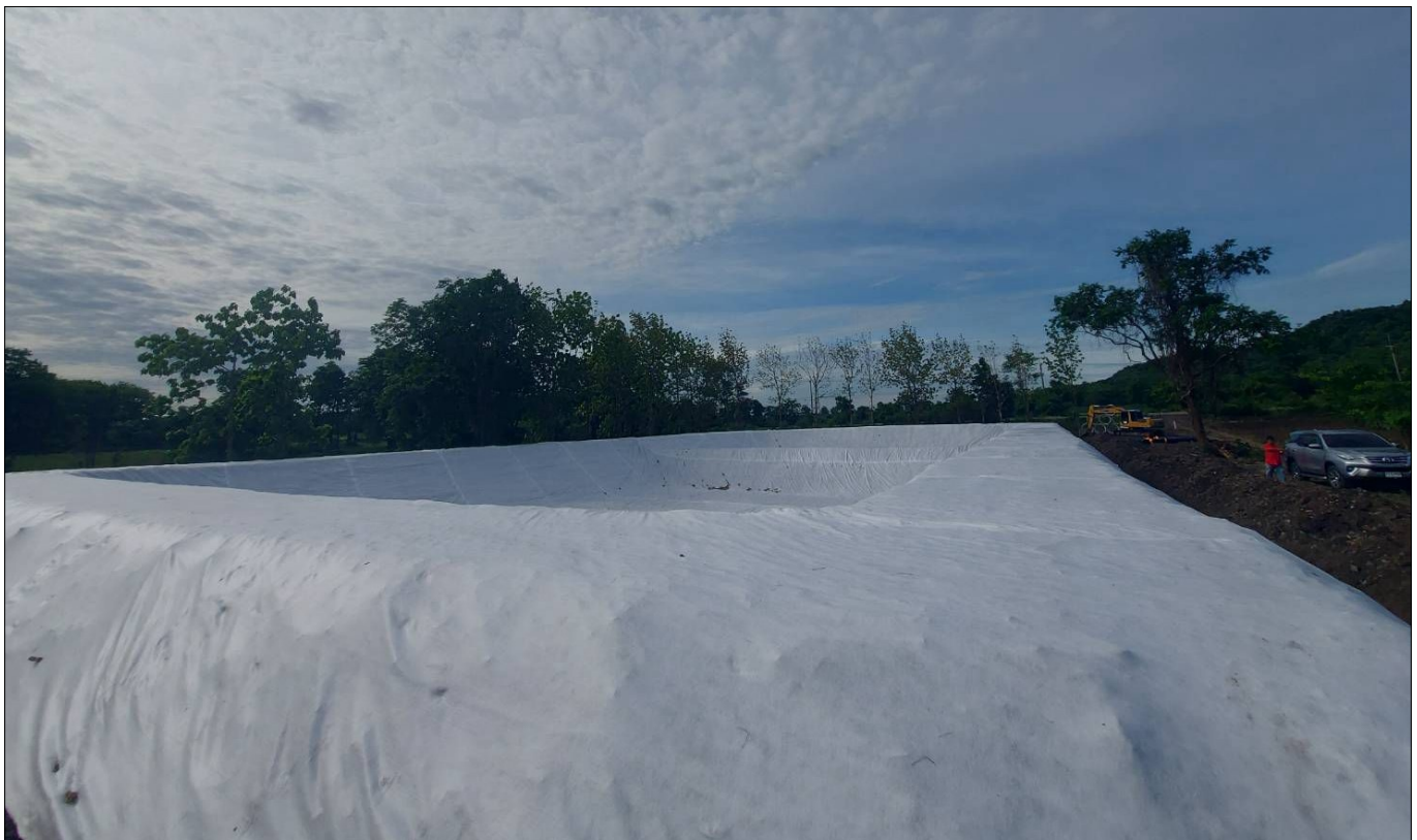
Photo 1 : TechGeo Nonwoven Geotextile Installation
