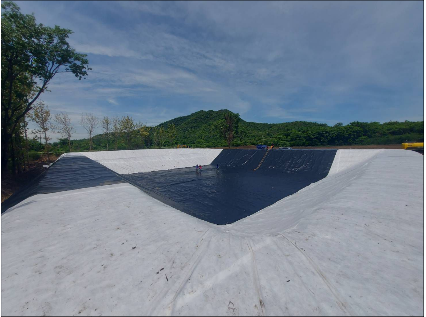
Photo 2 : Geomembrane Installation Over Nonwoven Geotextile
