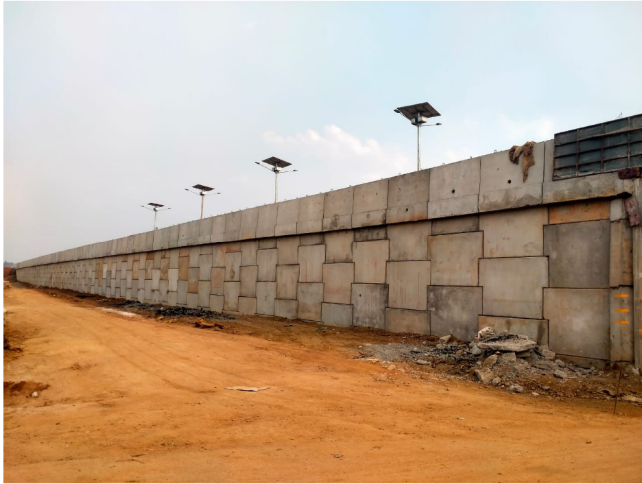
Photo 6: Completed Reinforced Soil Wall with Panel Facia and TechStrap
