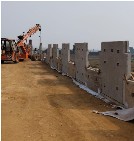
Photo 2: Erection of RCC Facia Panel
