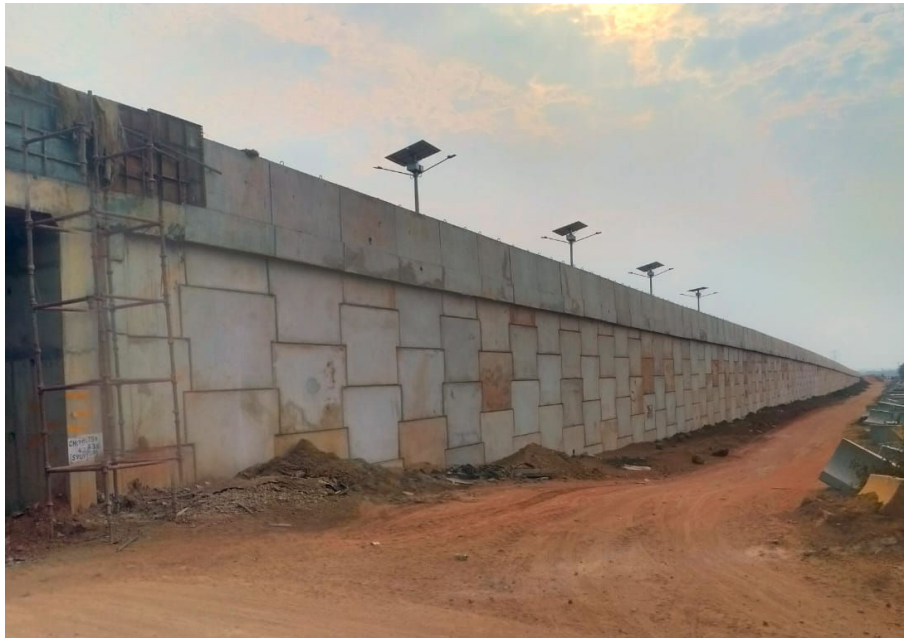
Photo 1: Elevation view of RS Wall
