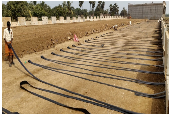
Photo 3: Installation of TechStrap Polymeric Strip
