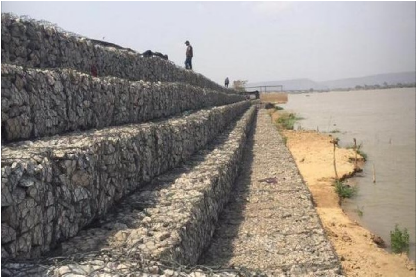
Completed Structure of Gabion Wall
