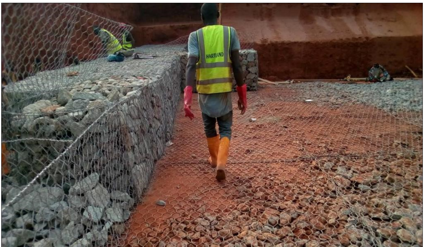
During Construction Photographs - Gabion filling with boulders
