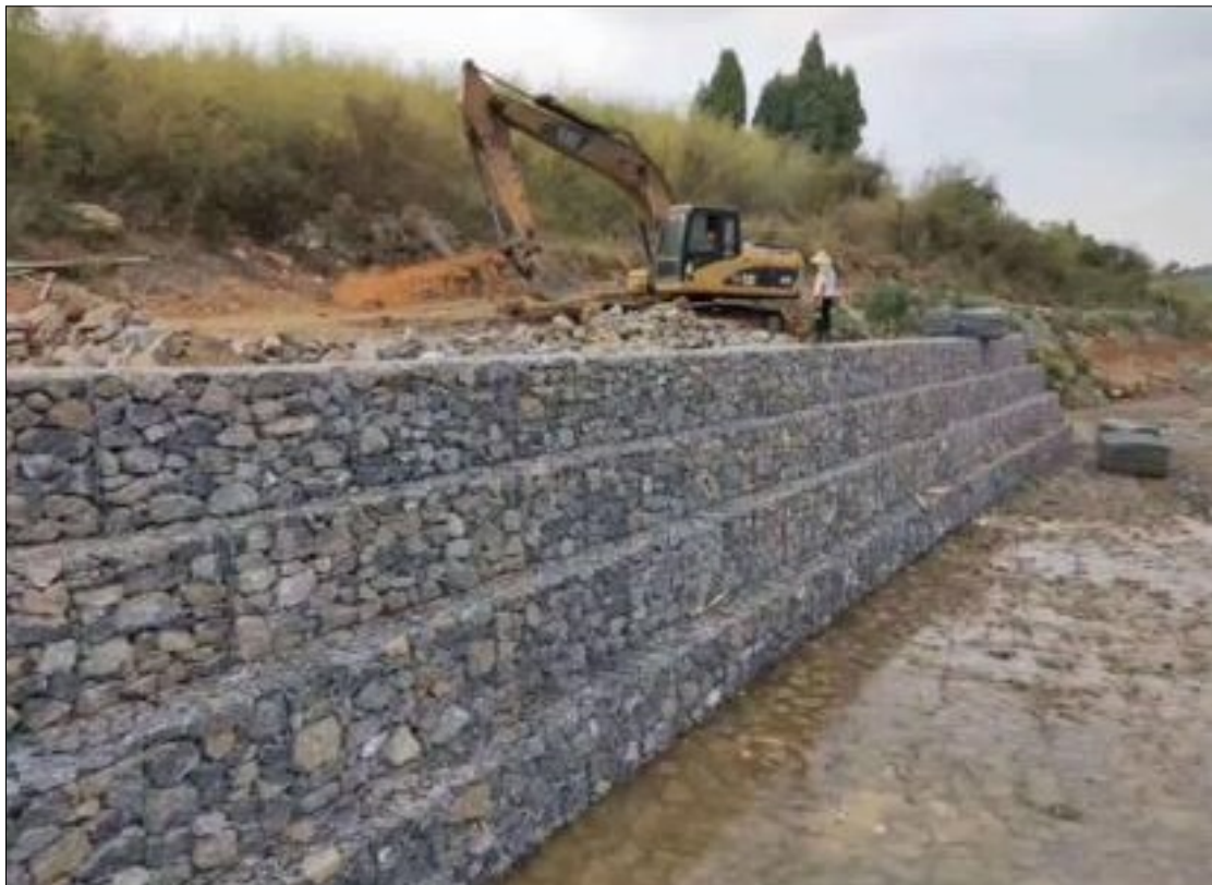
During Construction Photograph
