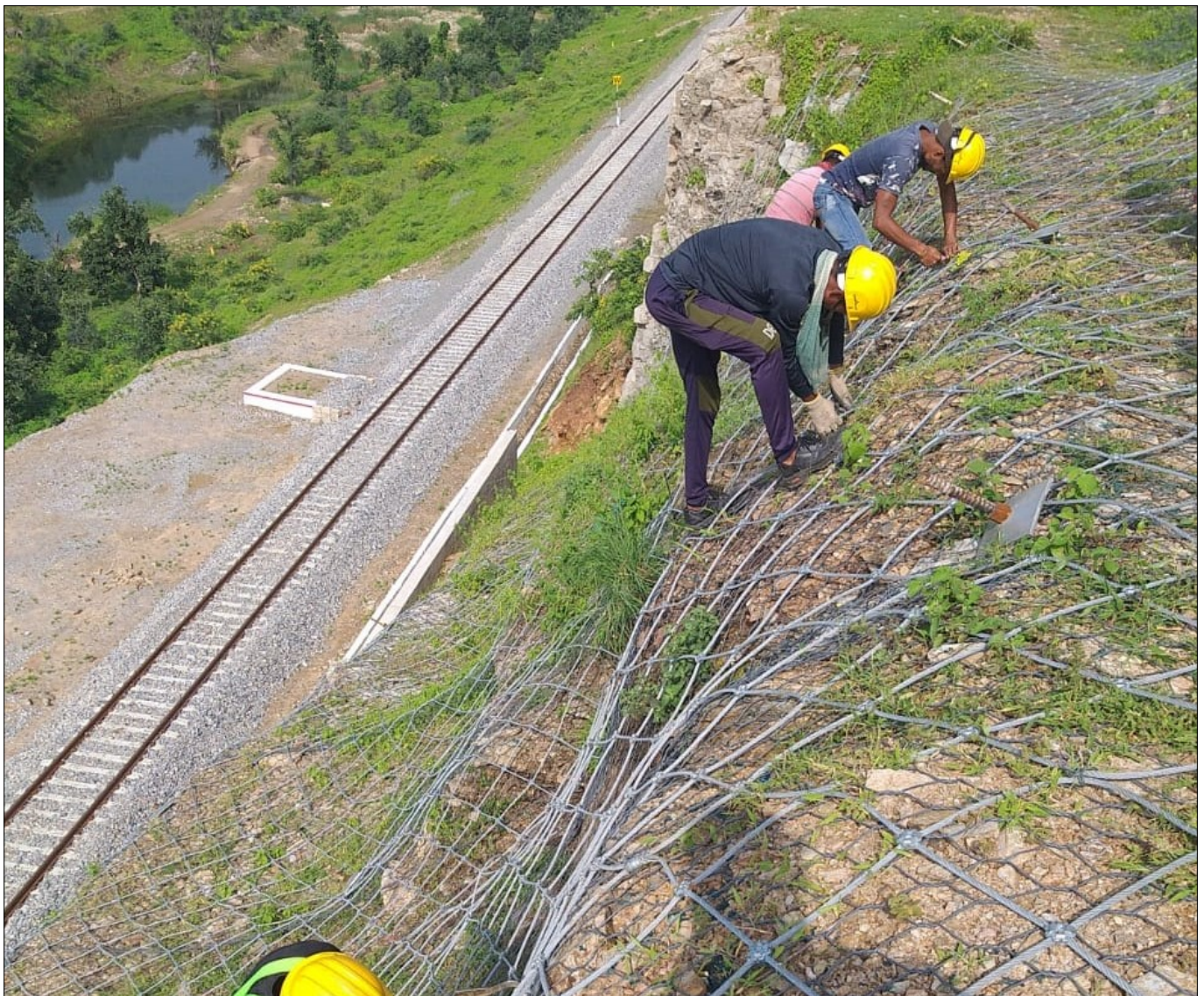
Photo 3 : Ensuring Safety: Installation of Rockfall Protection Systems
