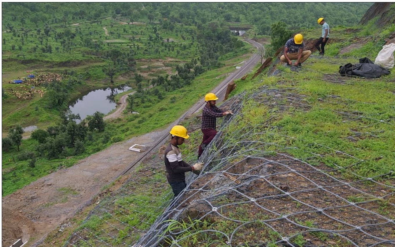
Photo 7 : Ensuring Proper Installation
