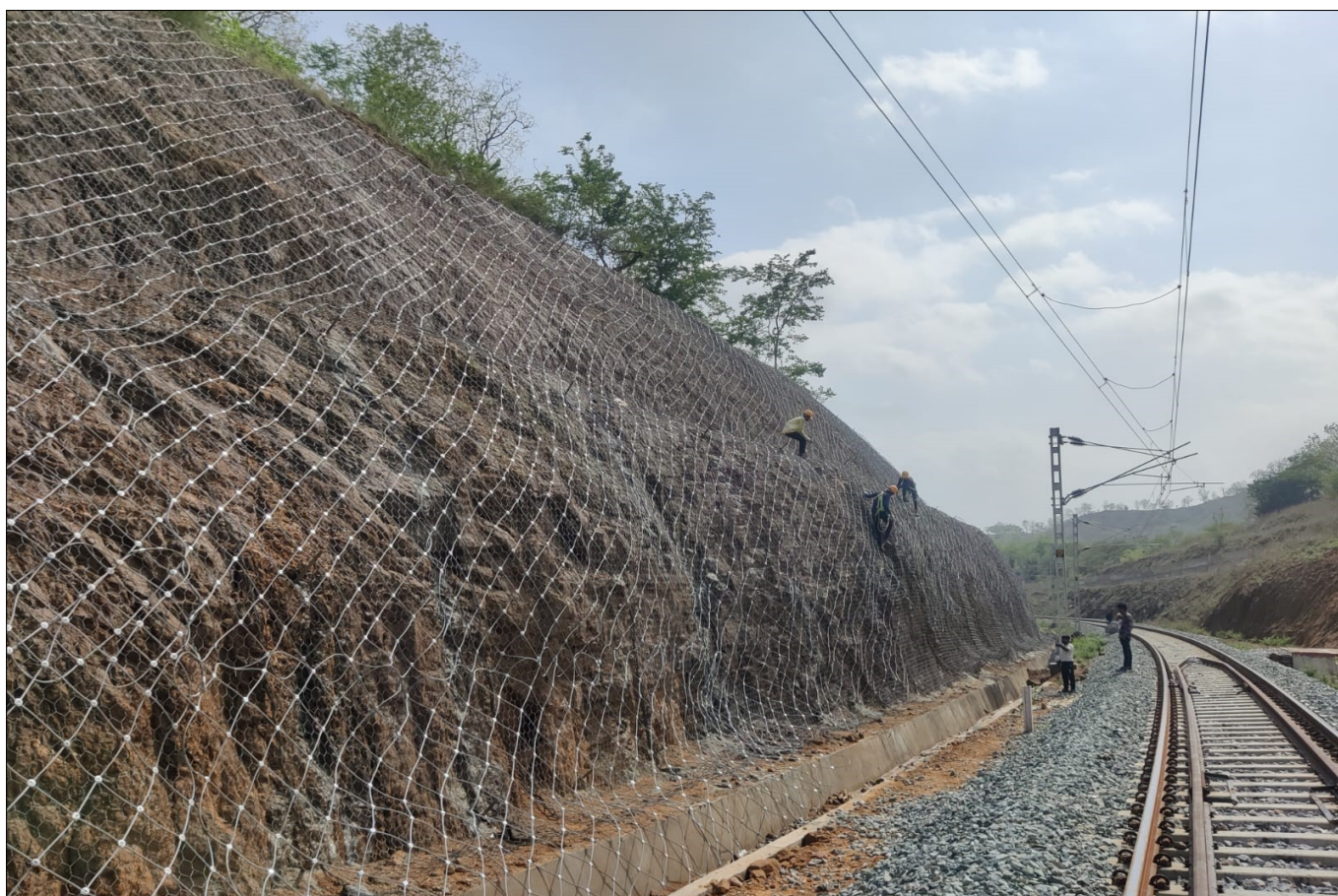
Photo 8 : Secured Slope : Post-Installation of Rockfall Protection Measures
