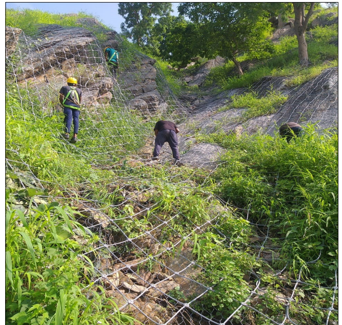
Photo 1 & 2 : Construction Progress: Primary and Secondary Mesh Integration
