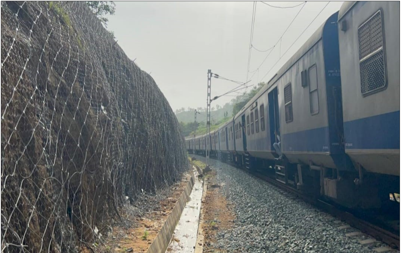
Photo 9 : Open for Traffic: Completed Structure
