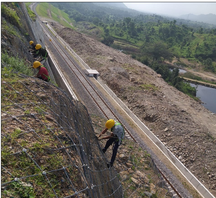
Photo 1 & 2 : Construction Progress: Primary and Secondary Mesh Integration
