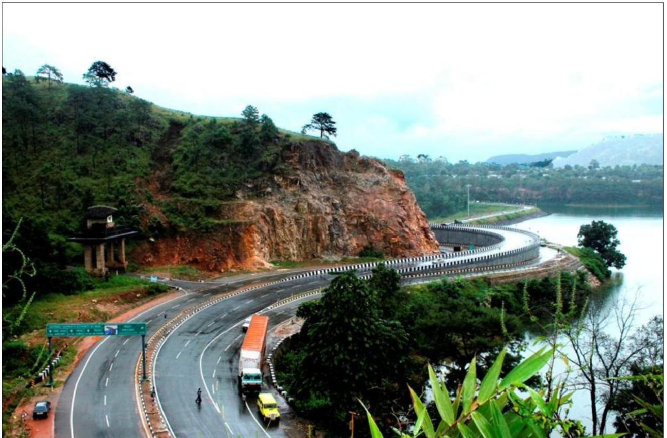
Before implementation of Rockfall Netting
