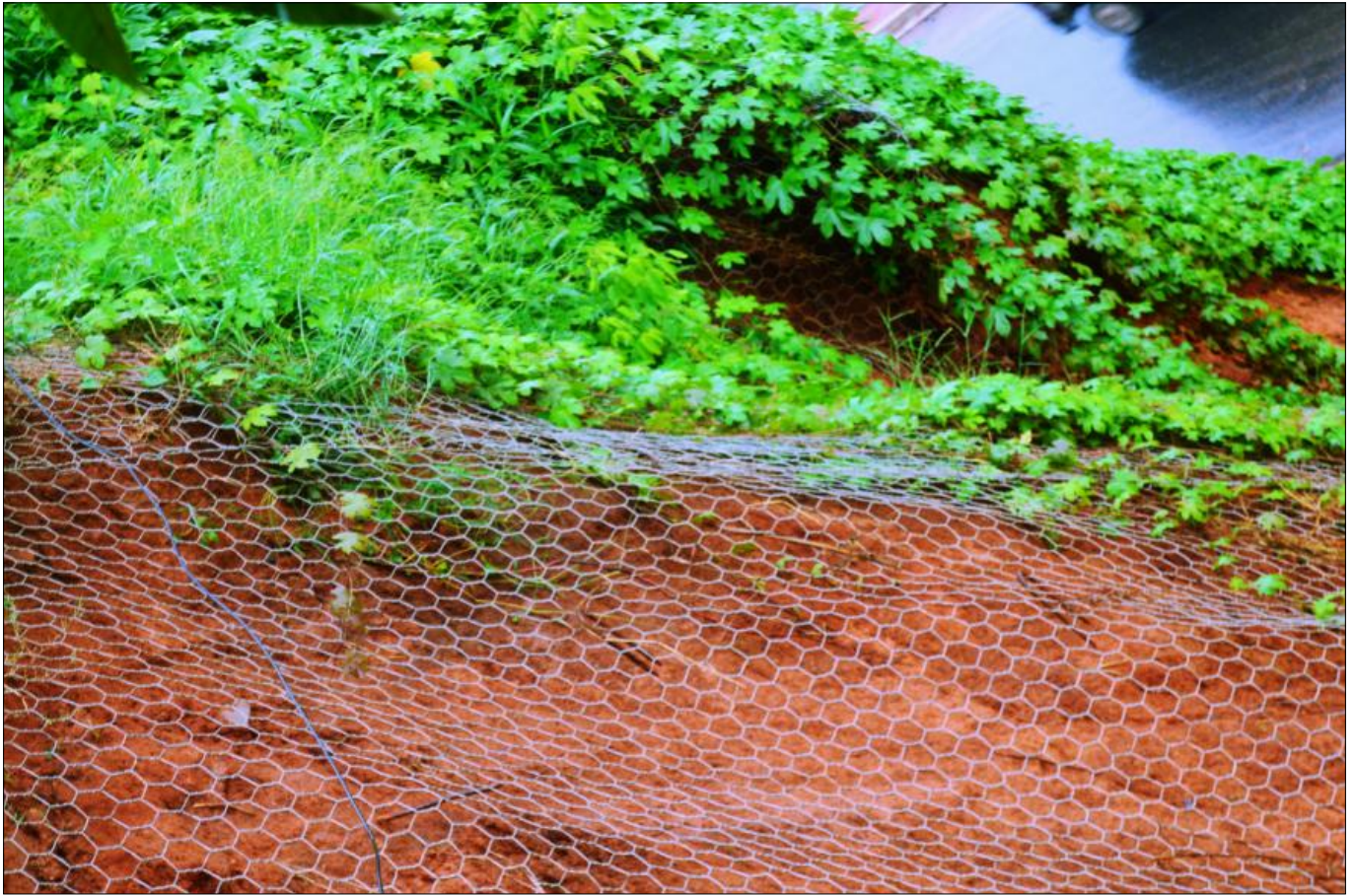
Structure after 7 years
