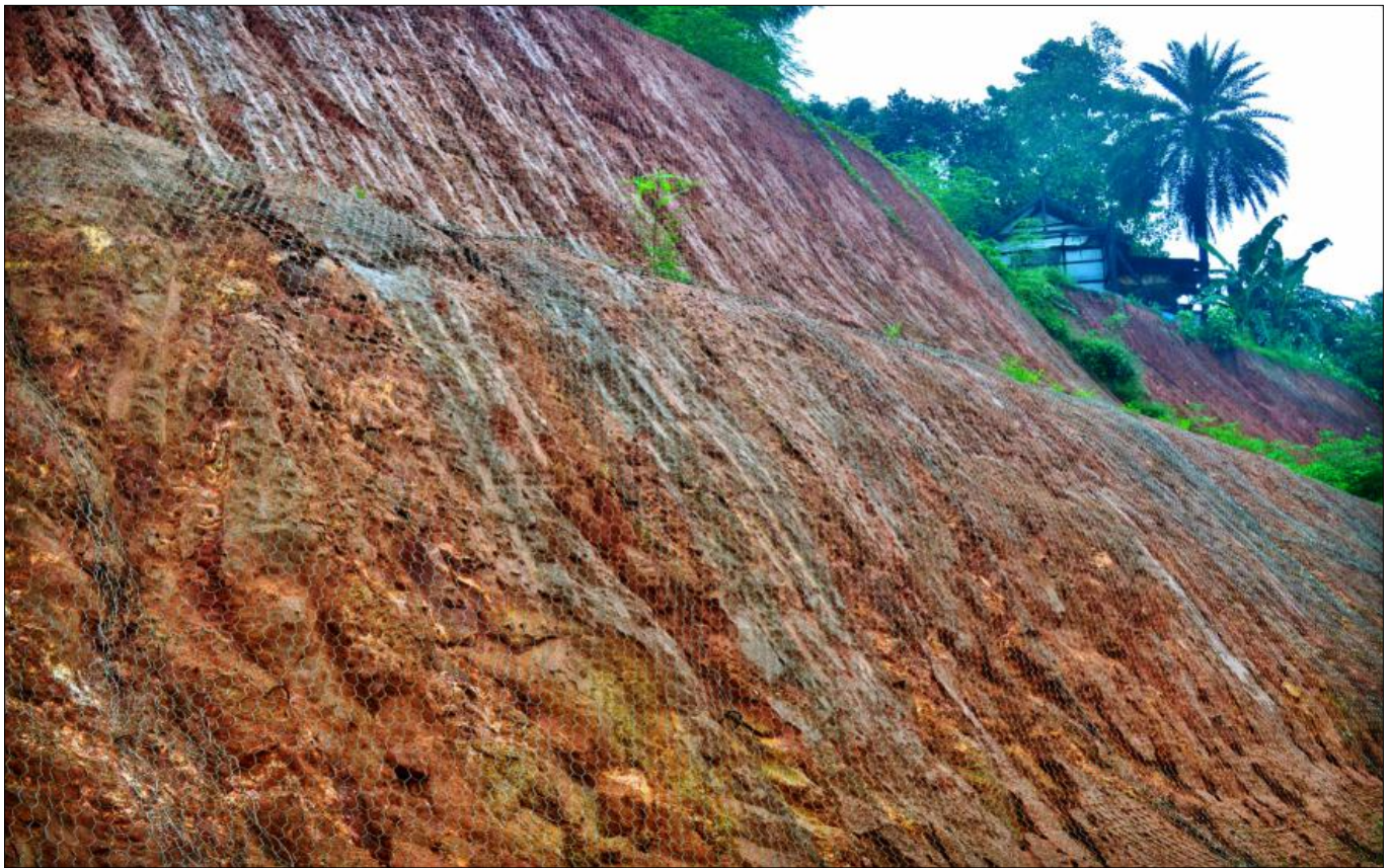
Slope after installation of Rockfall Netting
