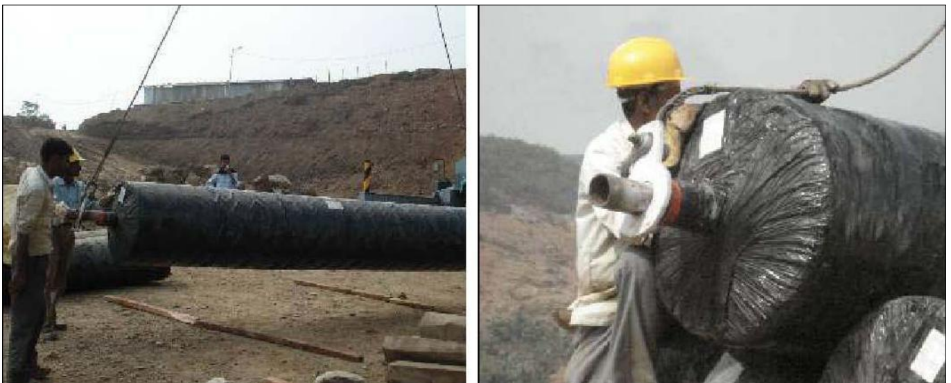
Handling of Geosynthetic Rolls
