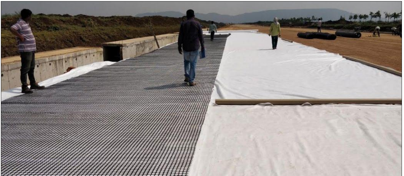
Unrolling of Geogrid & Geotextile and Inspection for any wrinkles
