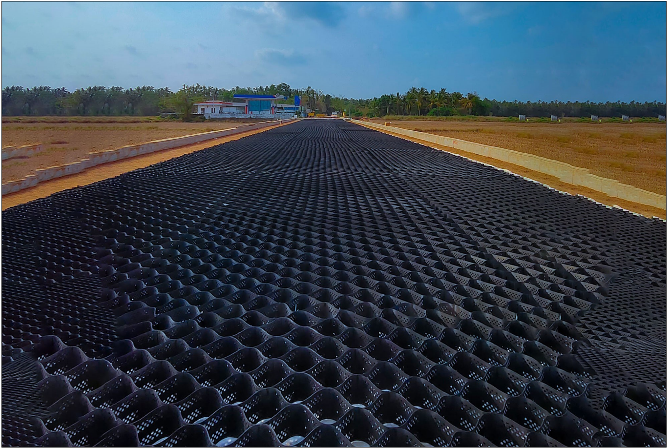
Photo 2 : Spreading of TechCell Geocell
