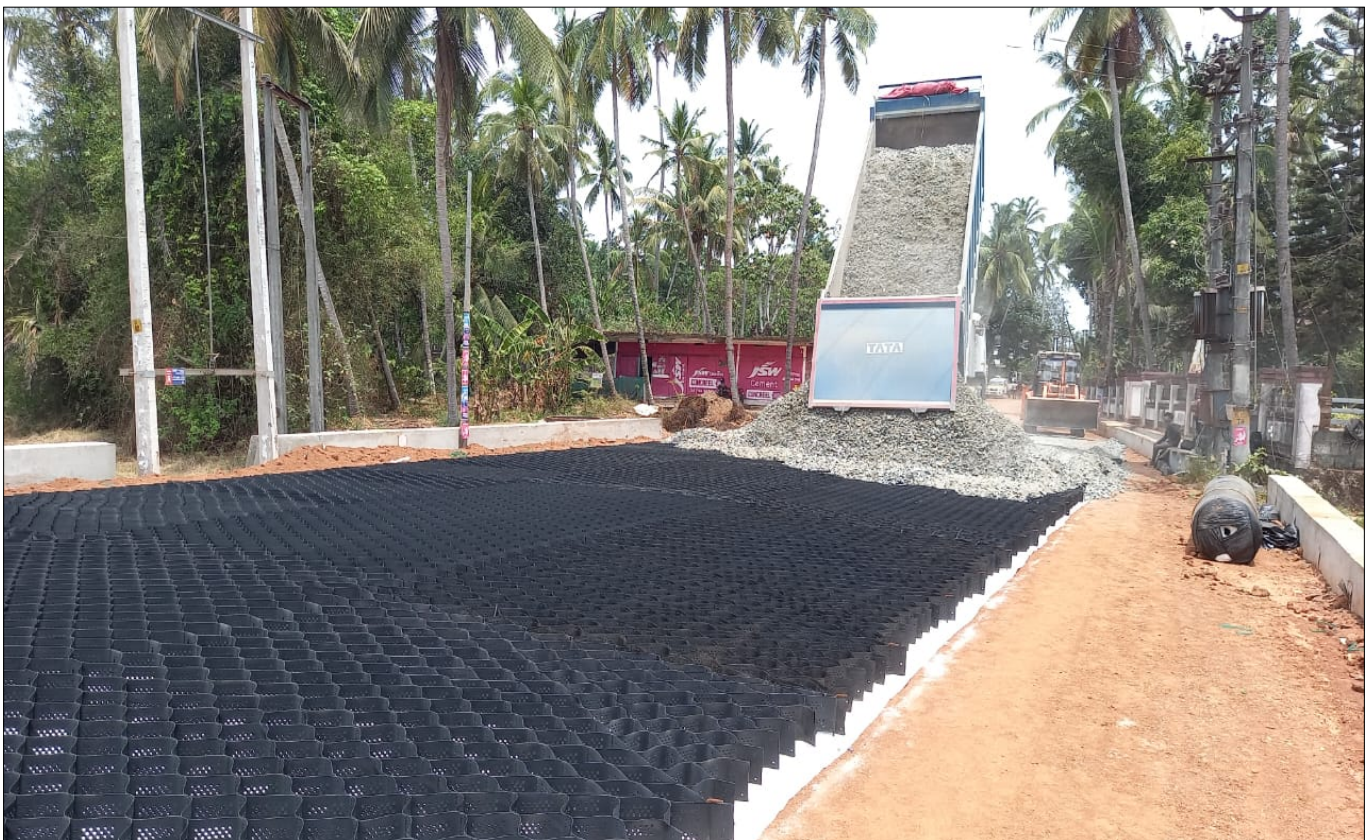
Photo 3 : - Filling of granular material into the TechCell Geocell
