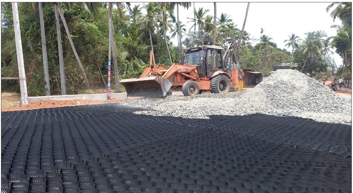
Photo 4 : - Compaction of granular material
