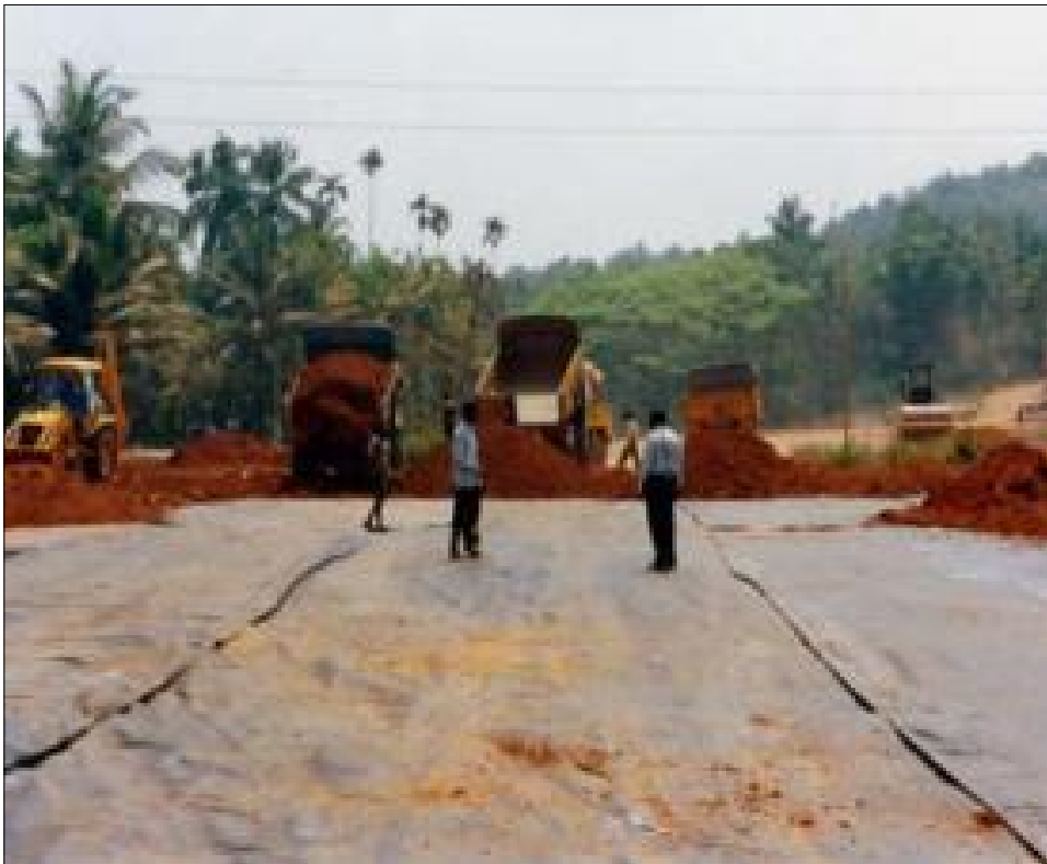
Installation of Techfab TPP 250 Woven Geotextile
