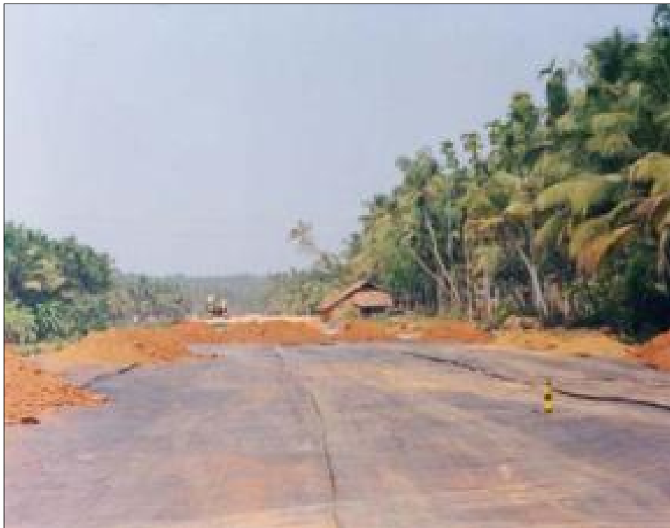
Installation of Techfab TPP 250 Woven Geotextile
