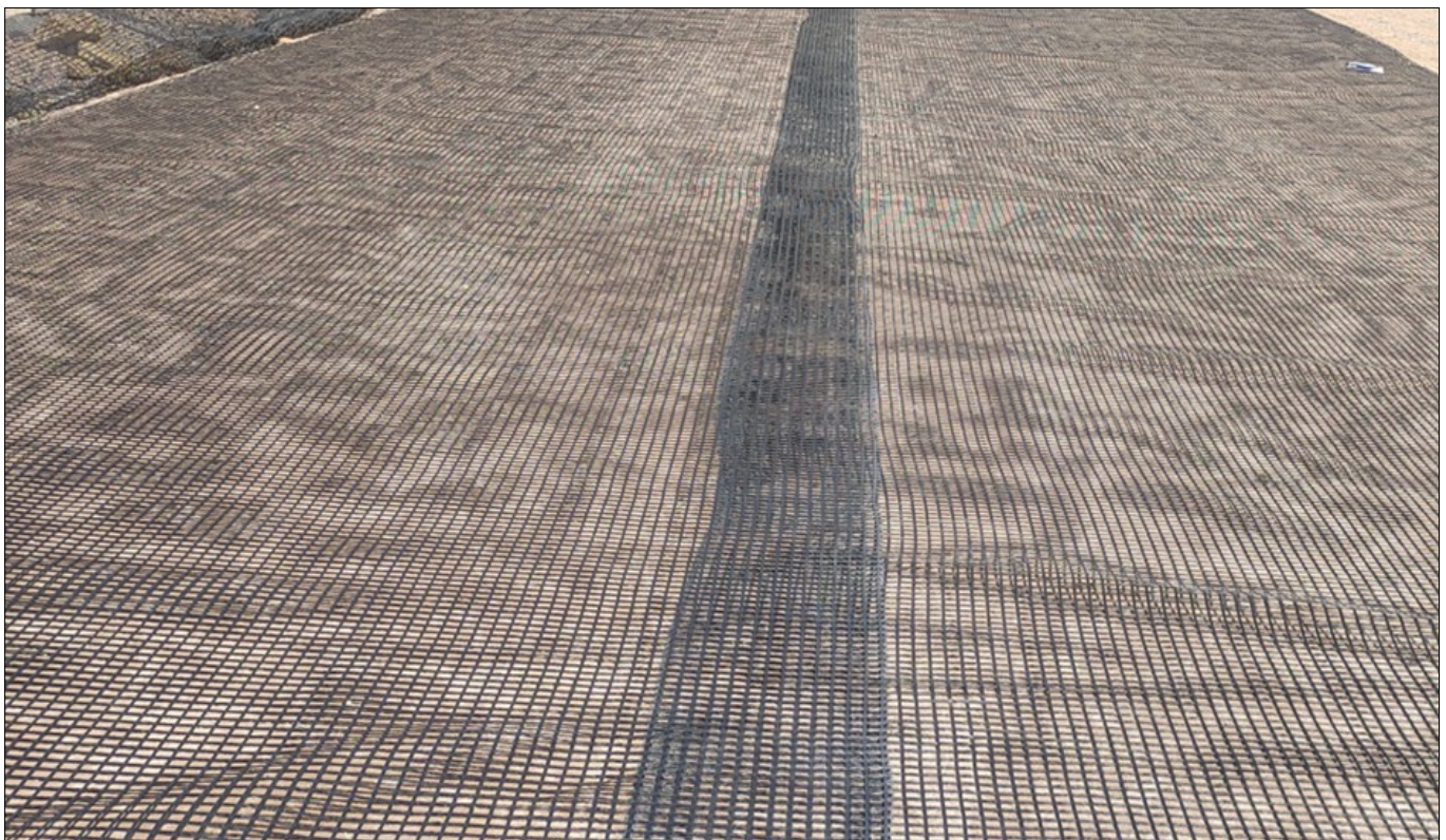
Photo 3 : Securing the ends of the geogrid with “J” hooks
