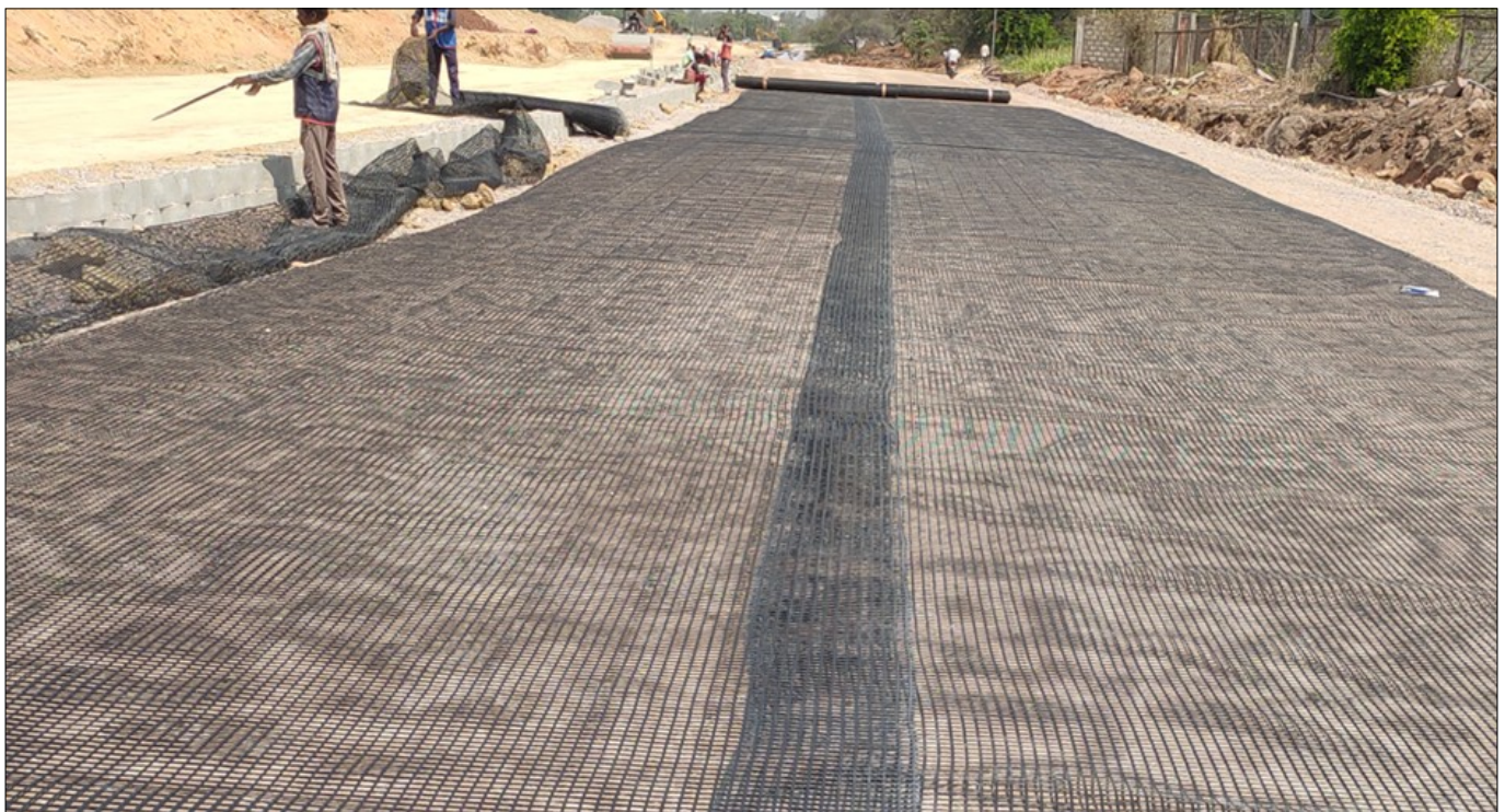
Photo 2 : Unrolling of geogrid over finished GSB layer with lateral overlap of 300 mm
