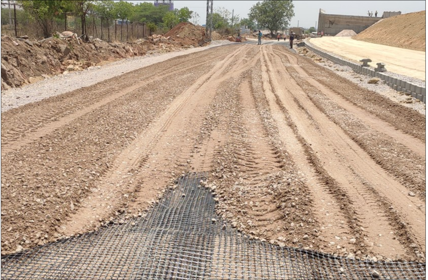
Photo 4 : Spreading of first layer of WMM material over Geogrid
