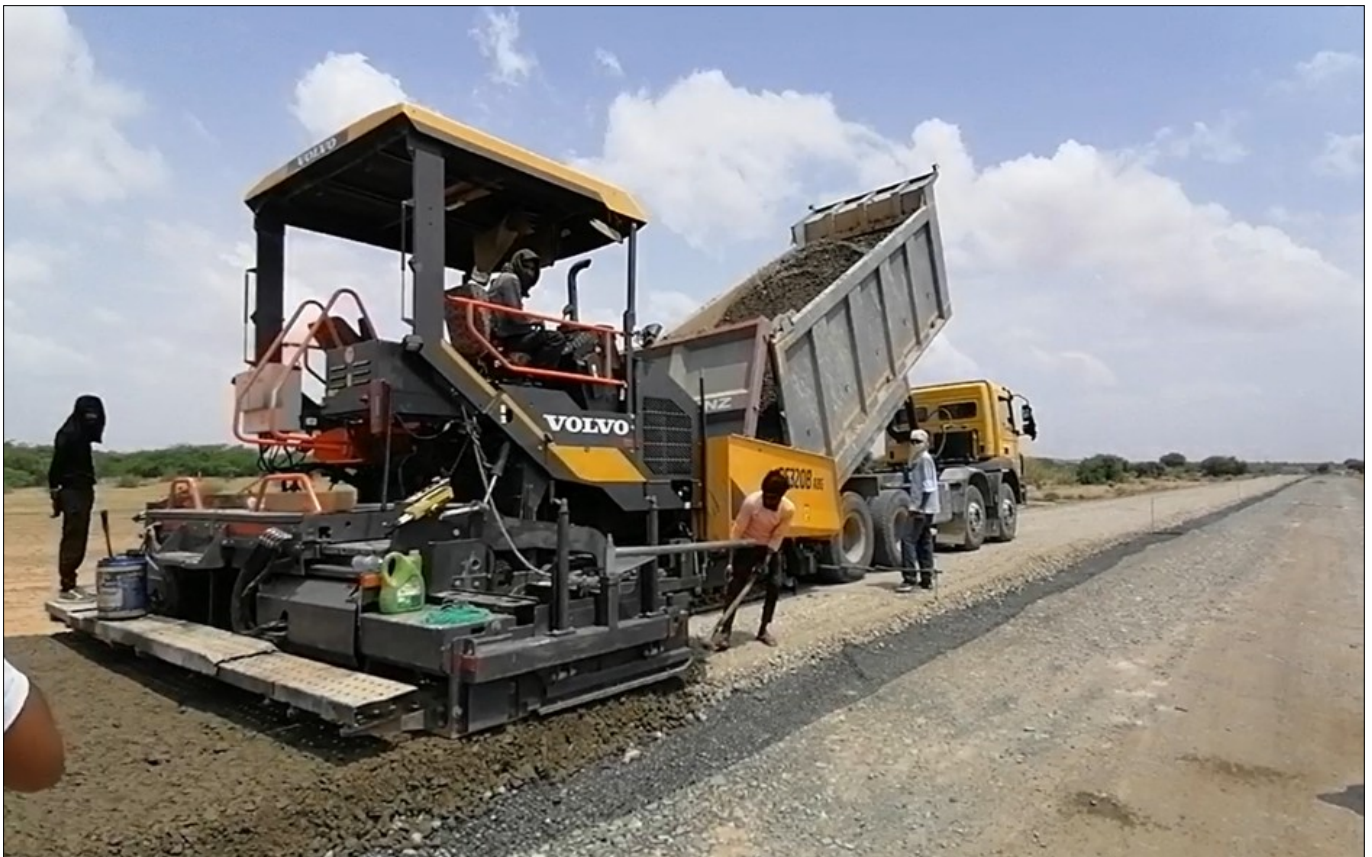
Photo 5 : Laying of second layer of WMM material
