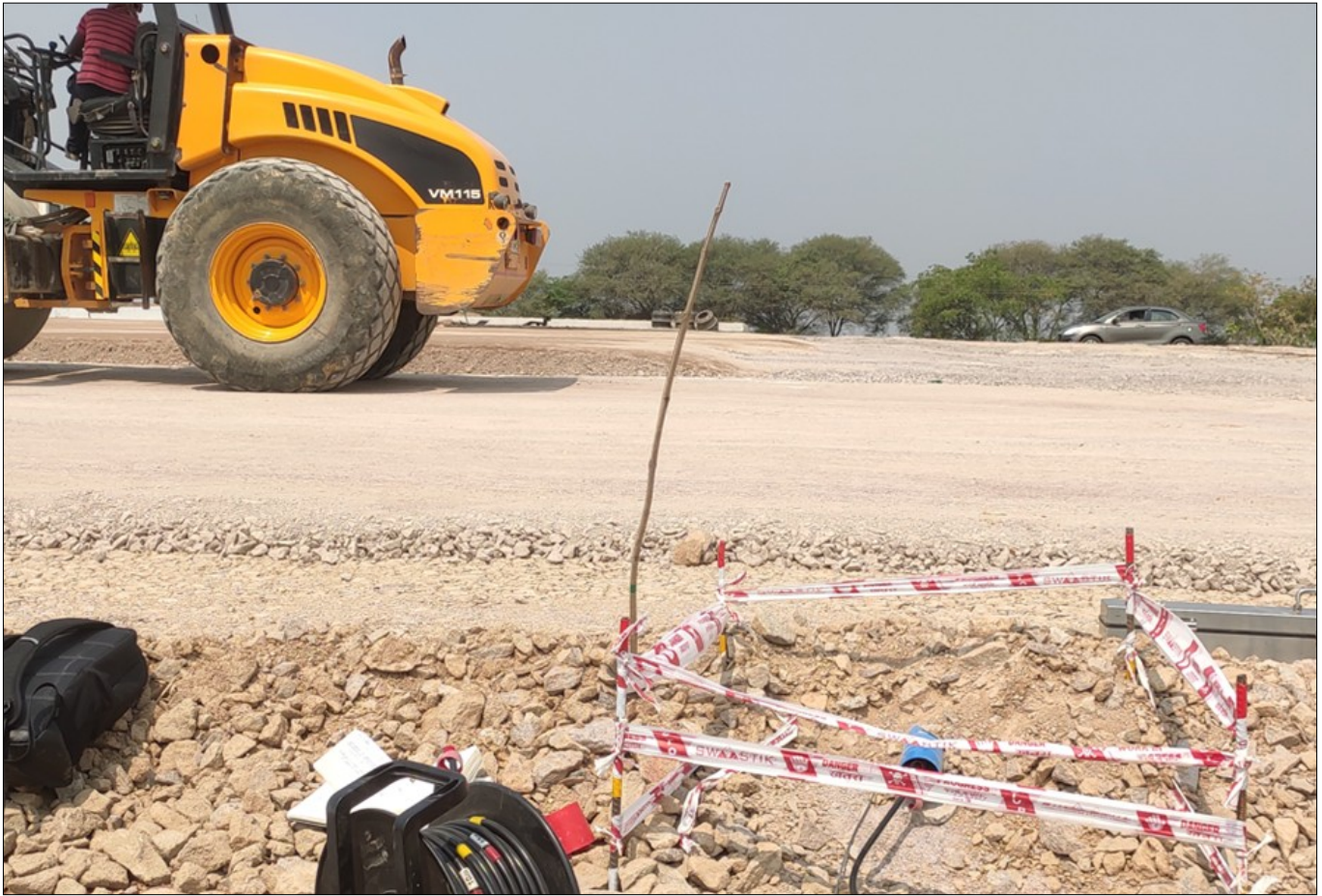
Photo 6 : Finished pavement surface
