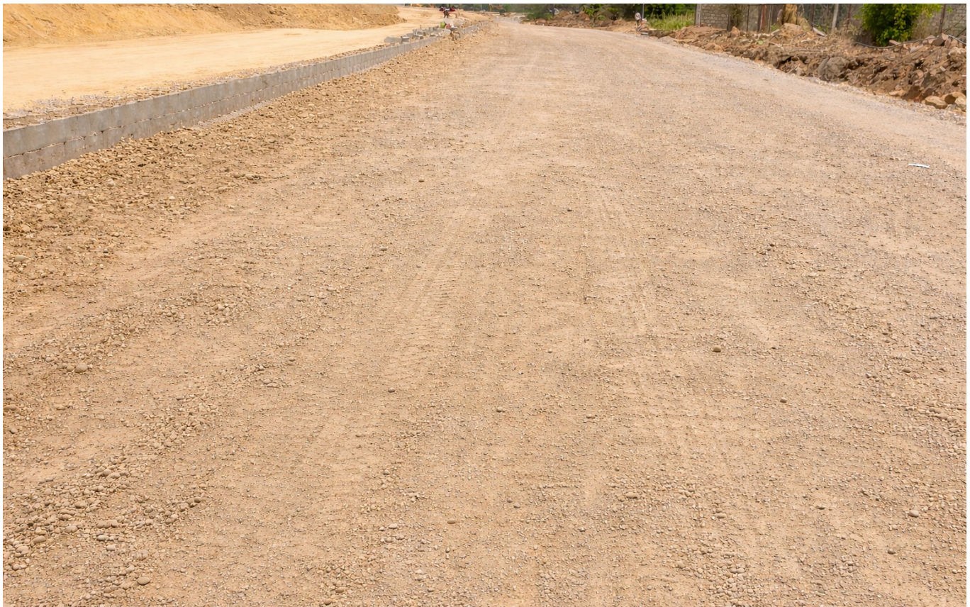
Photo 1 : Initial Site Condition Prior to Pavement Stabilization Works
