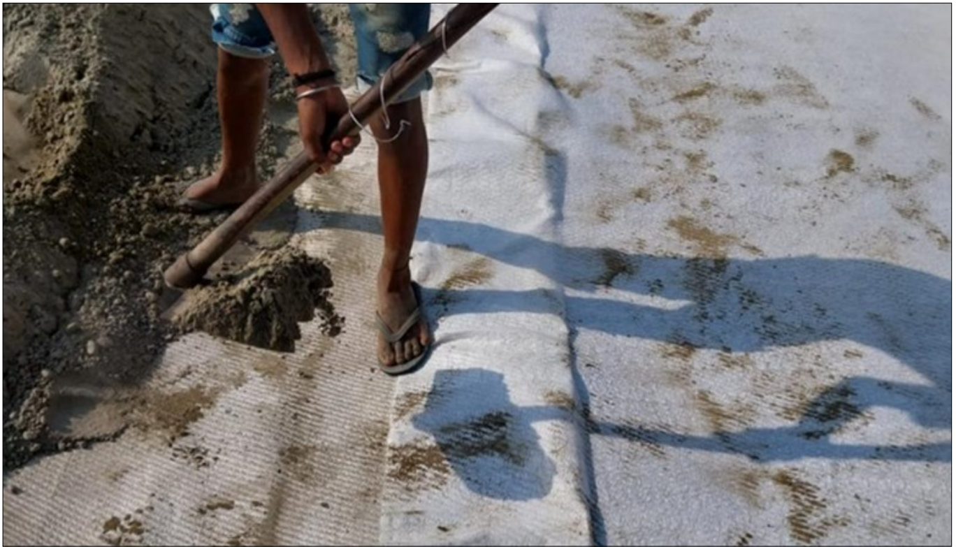
Figure 5 : Overlap of 300 mm maintained for adjacent rolls
