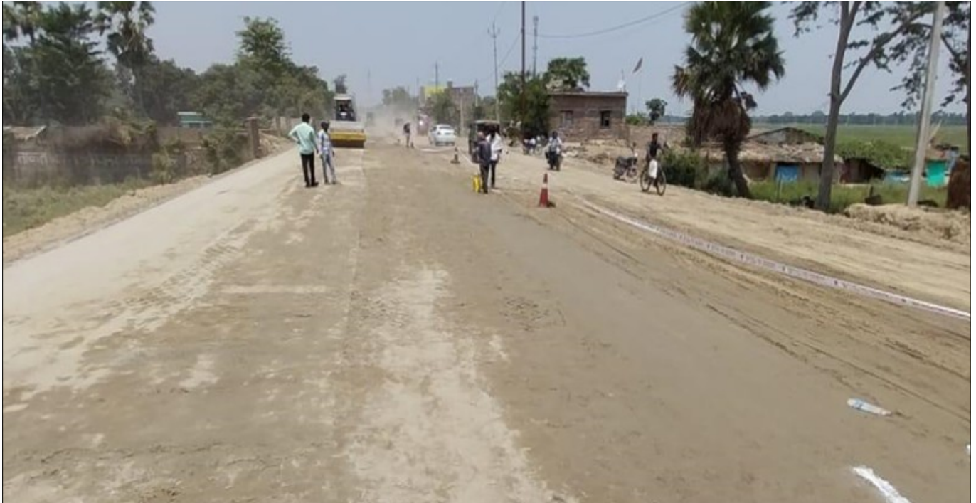
Figure 3 : Prepared subgrade by removing vegetation and unsuitable material
