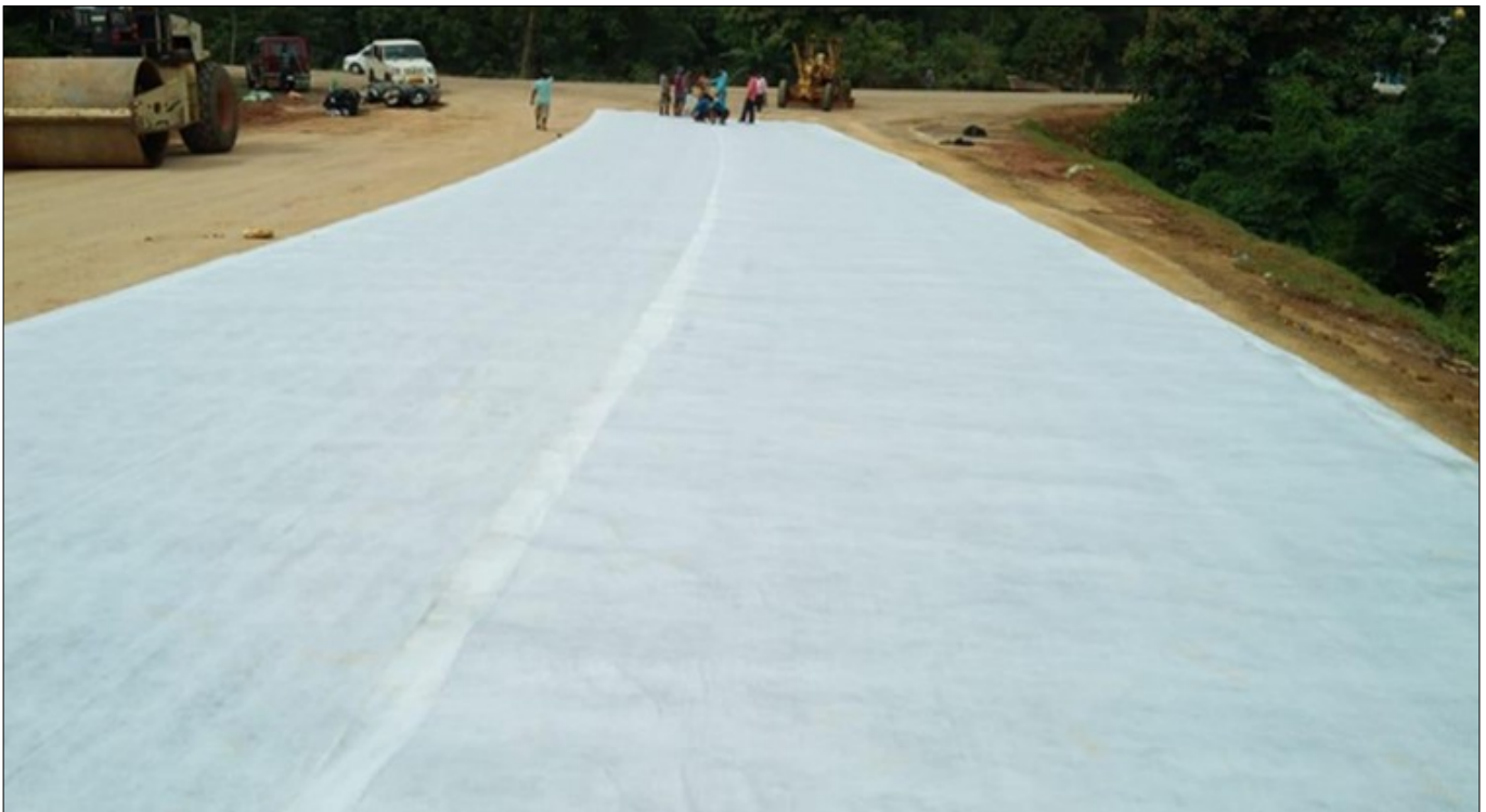
Figure 6 : Site inspection of installed drainage composite
