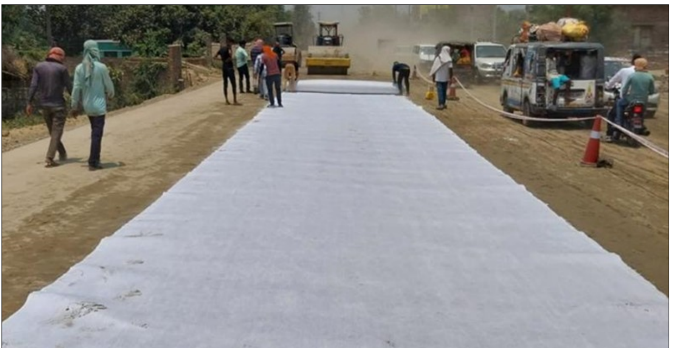
Figure 4 : Unrolling of drainage composite over prepared subgrade
