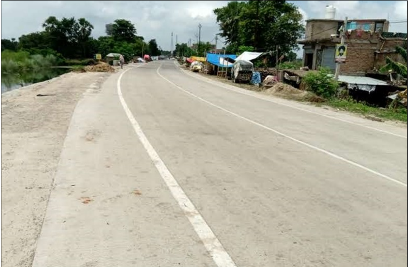
Figure 9 : Completion of project
