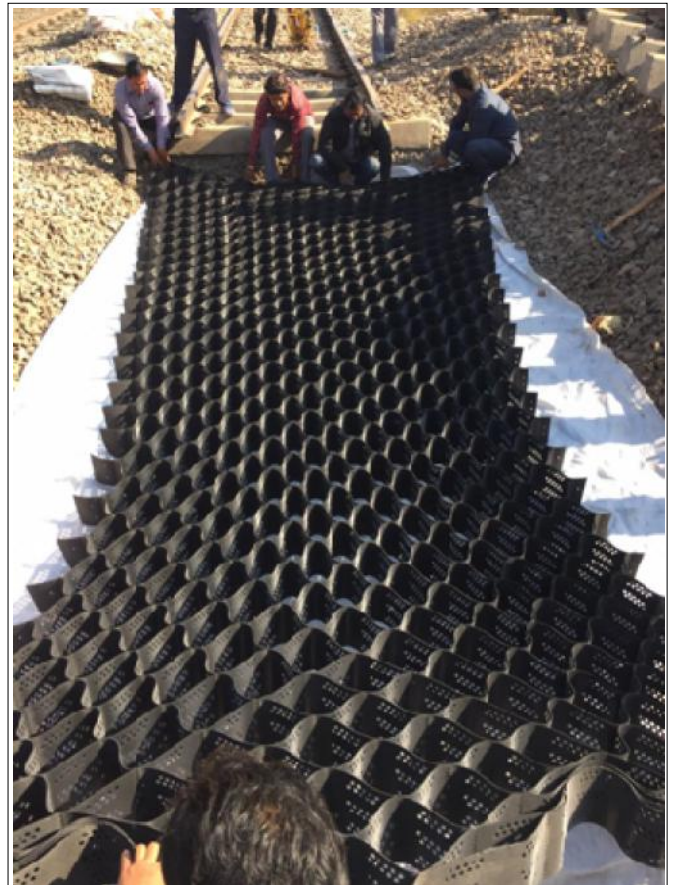
Laying of Techcell Geocell in Progress
