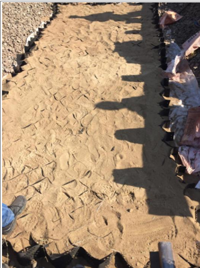
Filling of Techcell Geocell in Progress
