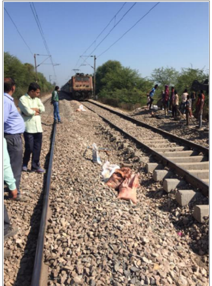
After laying of track in completed stretch
