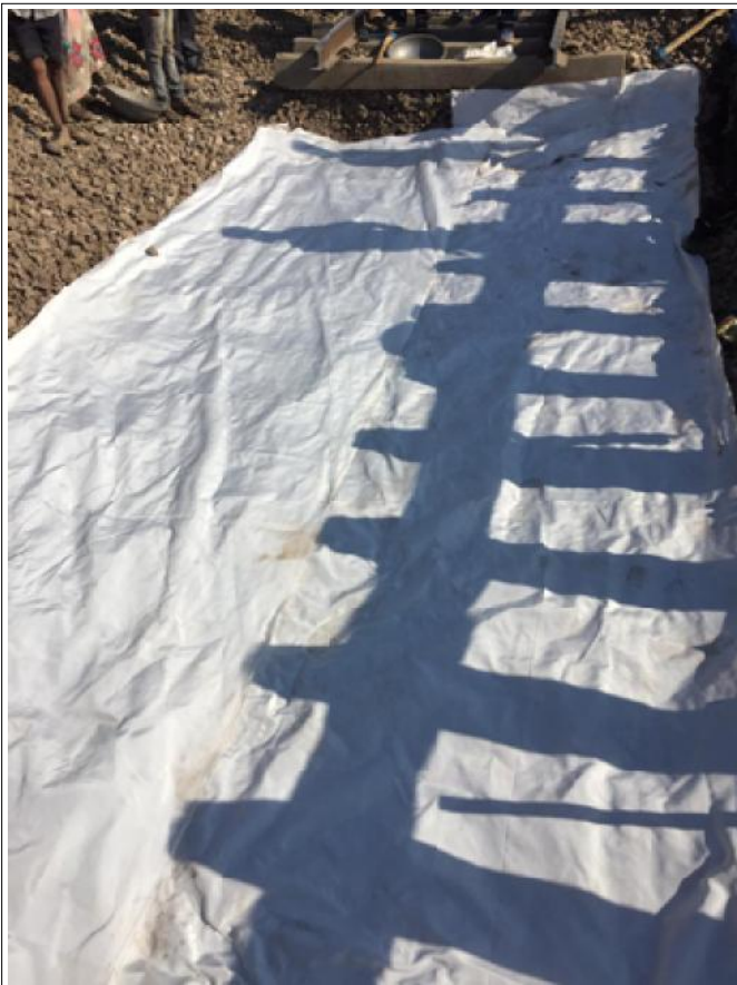
Laying of Woven Geotextile
