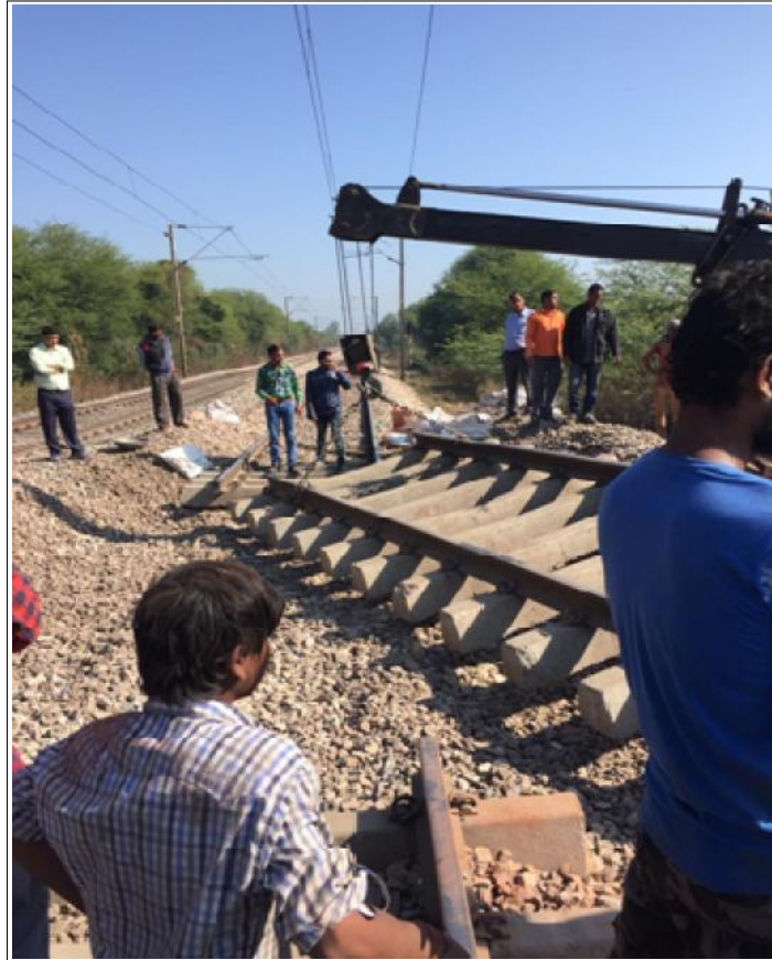
Removing another track panel
