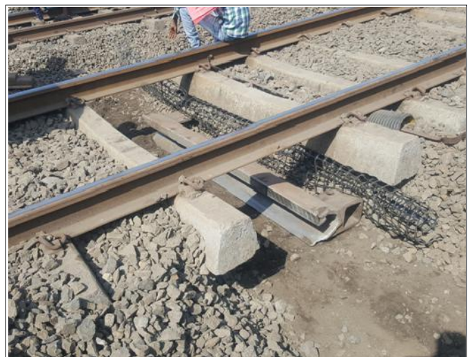
Placement of Sleeper Blade
