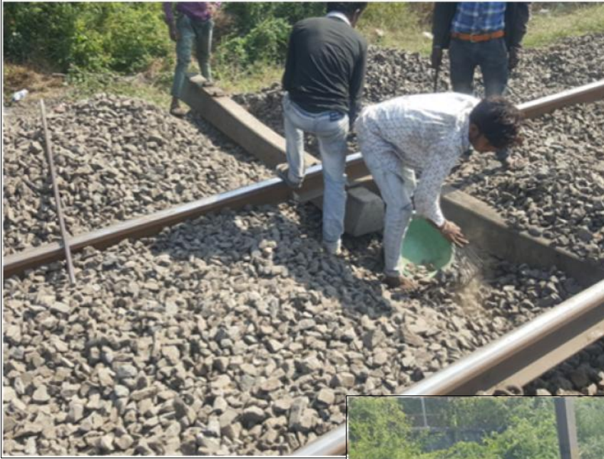
Placement of sleeper back to position
