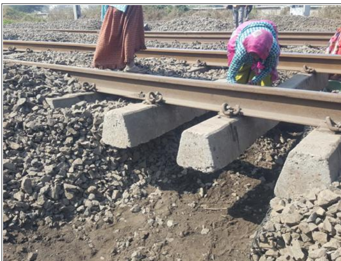
Manual Removal of Ballast in Progress
