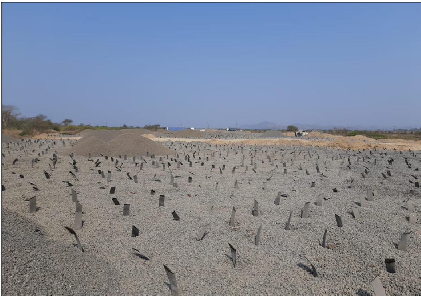
TechDrain PVD installed with preloading in progress
