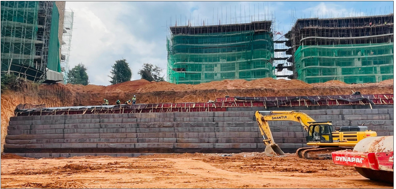
Photo 5 & 6 : During Construction – Reinforced Soil Wall Execution in Progress
