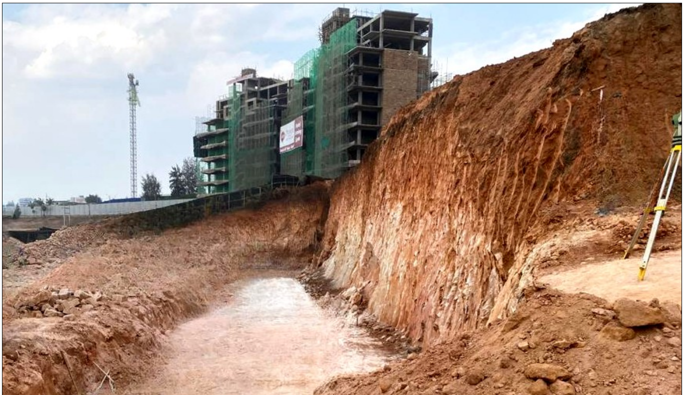
Photo 1 : Site Condition Before Reinforced Soil Wall Construction
