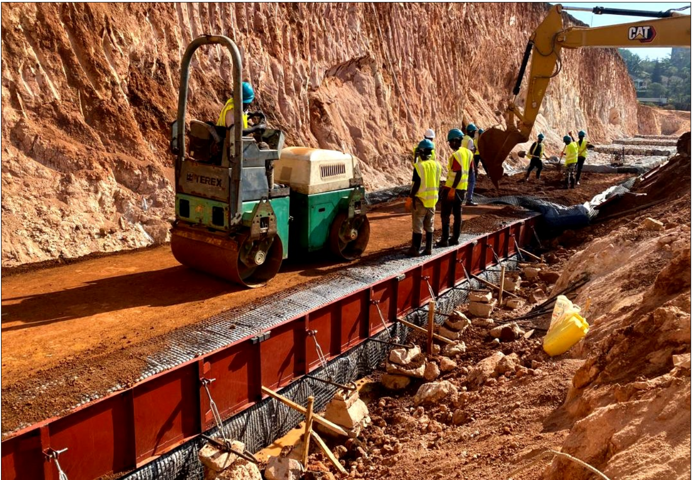
Photo 3 & 4 : Structural Filling and Compaction Works in Progress
