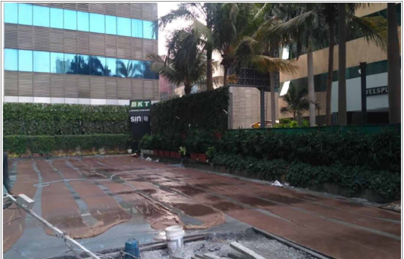
Concrete flooring above Techcell Geocell
