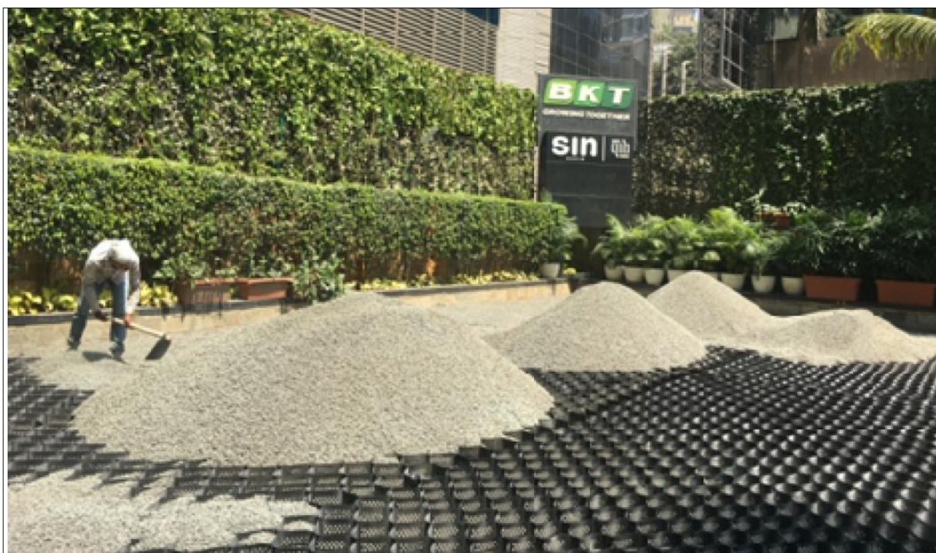
Filling of Geocell with Crushed stone/ Grit
