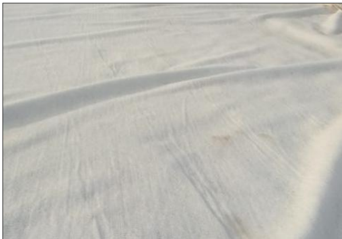
Photo 2 & 3 - Laying of Geotextile is in progress
