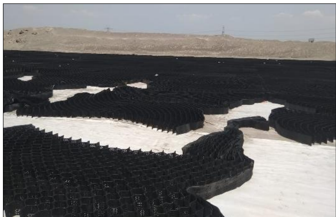
Photo 5 - Laying of Techcell Geocell
