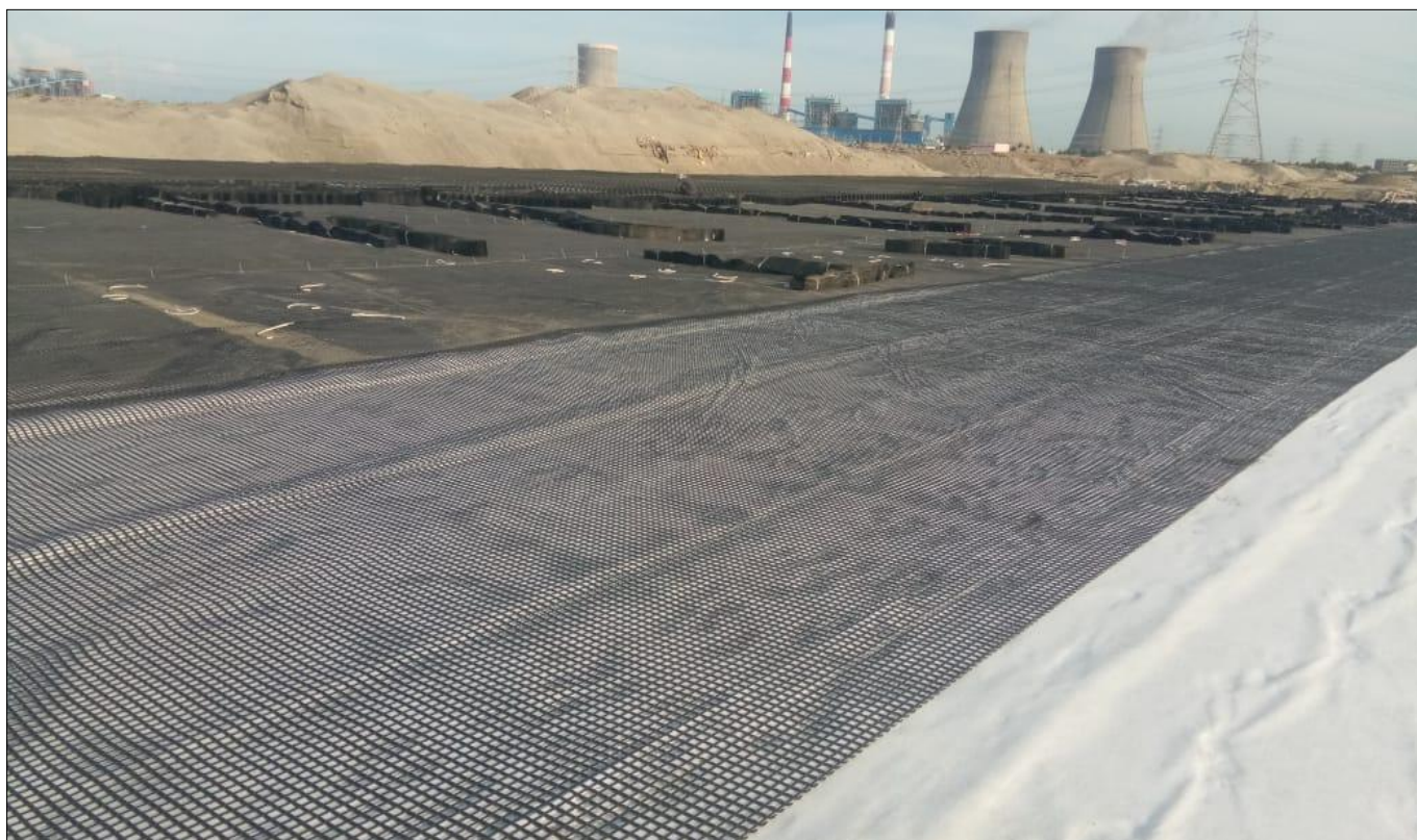
Photo 4 - Laying of TechGrid Biaxial Geogrid over geotextile
