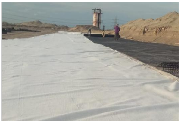
Photo 2 & 3 - Laying of Geotextile is in progress
