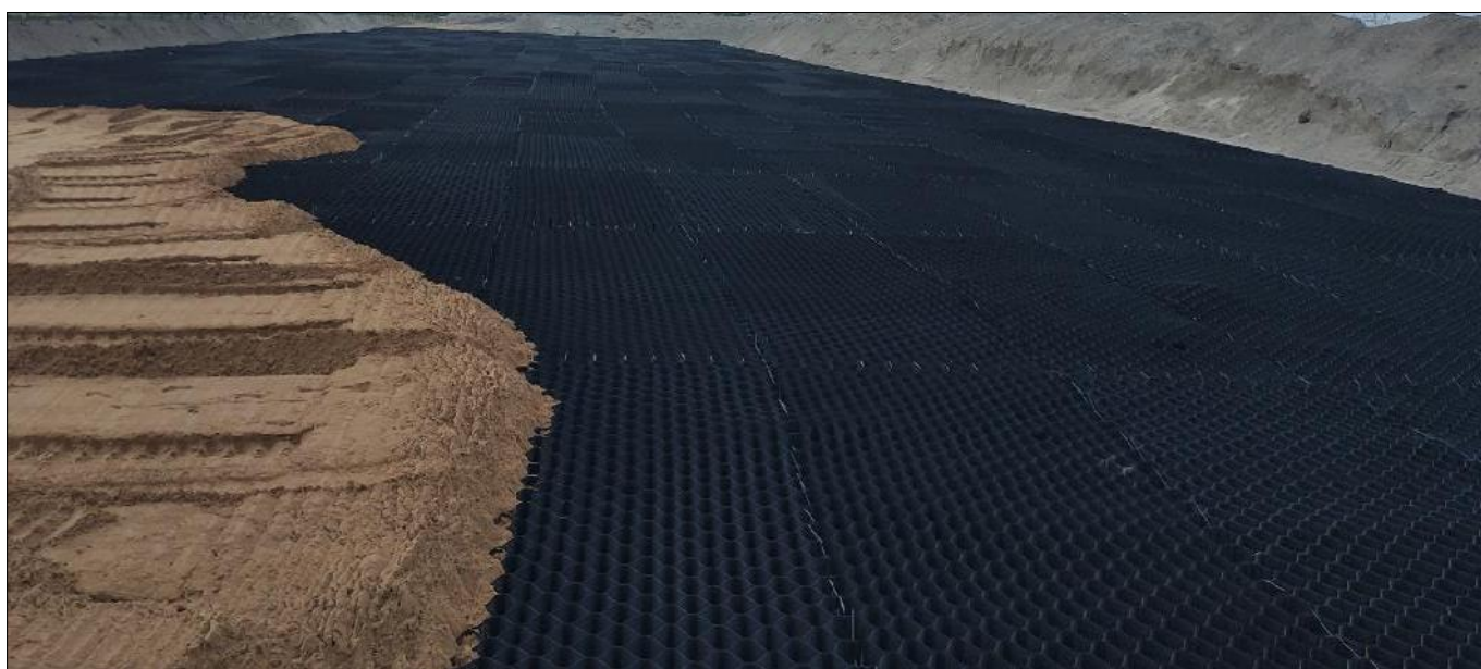
Photo 9 - Filling the Techcell Geocell with the infill material
