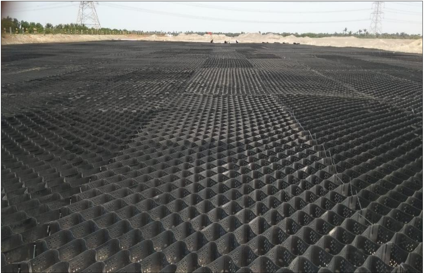
Photo 7 - Spreading of Techcell Geocell is in progress
