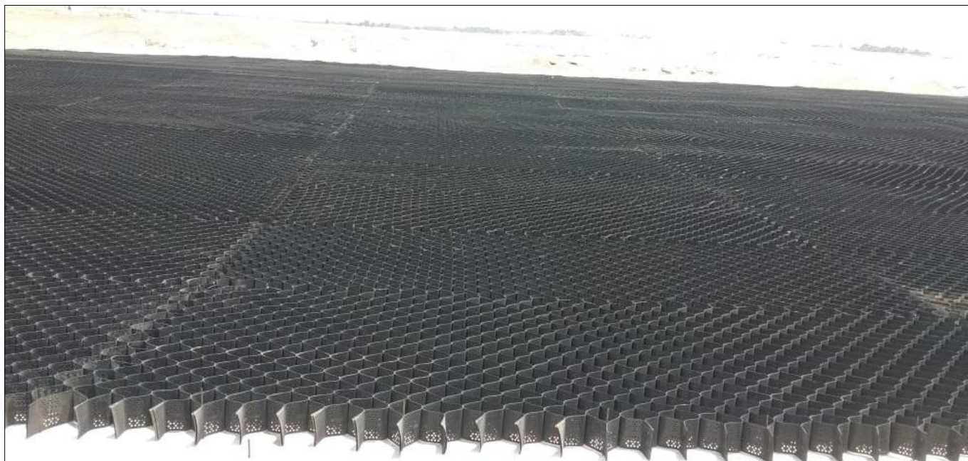
Photo 8 - Expanded Techcell Geocell
