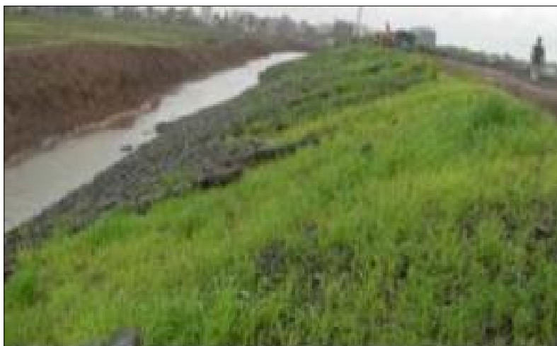
Embankment work in progress & partially completed
