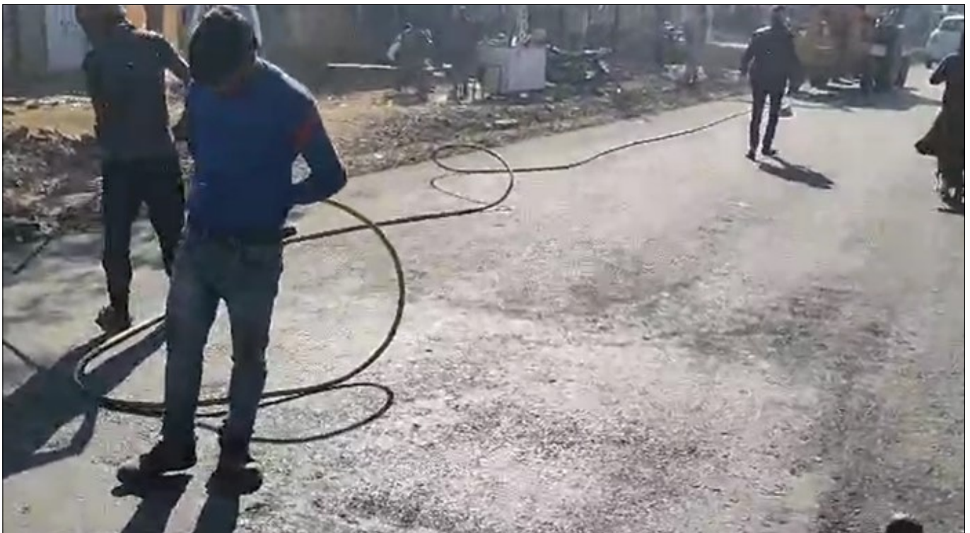
Photo 1 : Surface Cleaning & Potholes Filling
