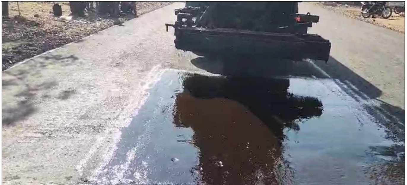
Photo 2 : Laying of Tack Coat on prepared surface
