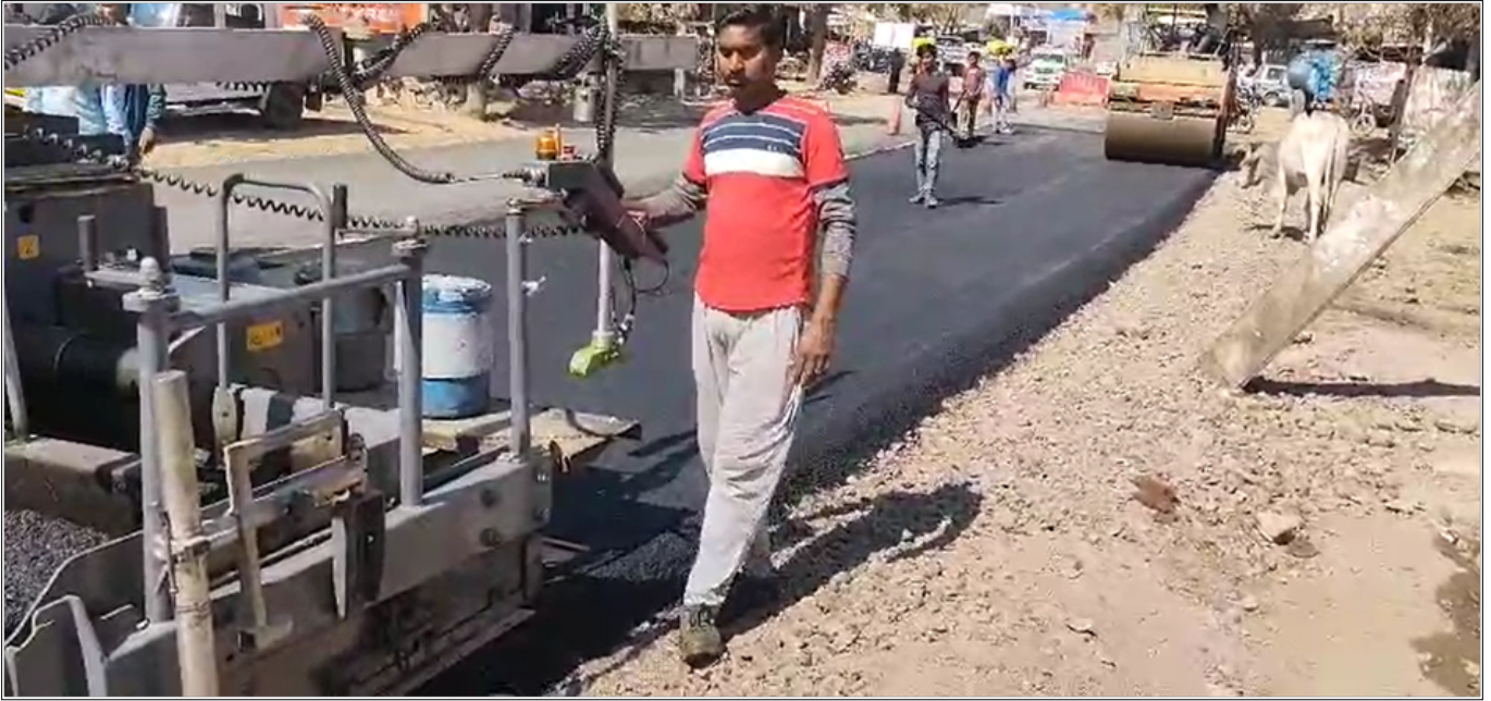
Photo 5 : Compaction of BC (Bituminous Concrete) Layer
