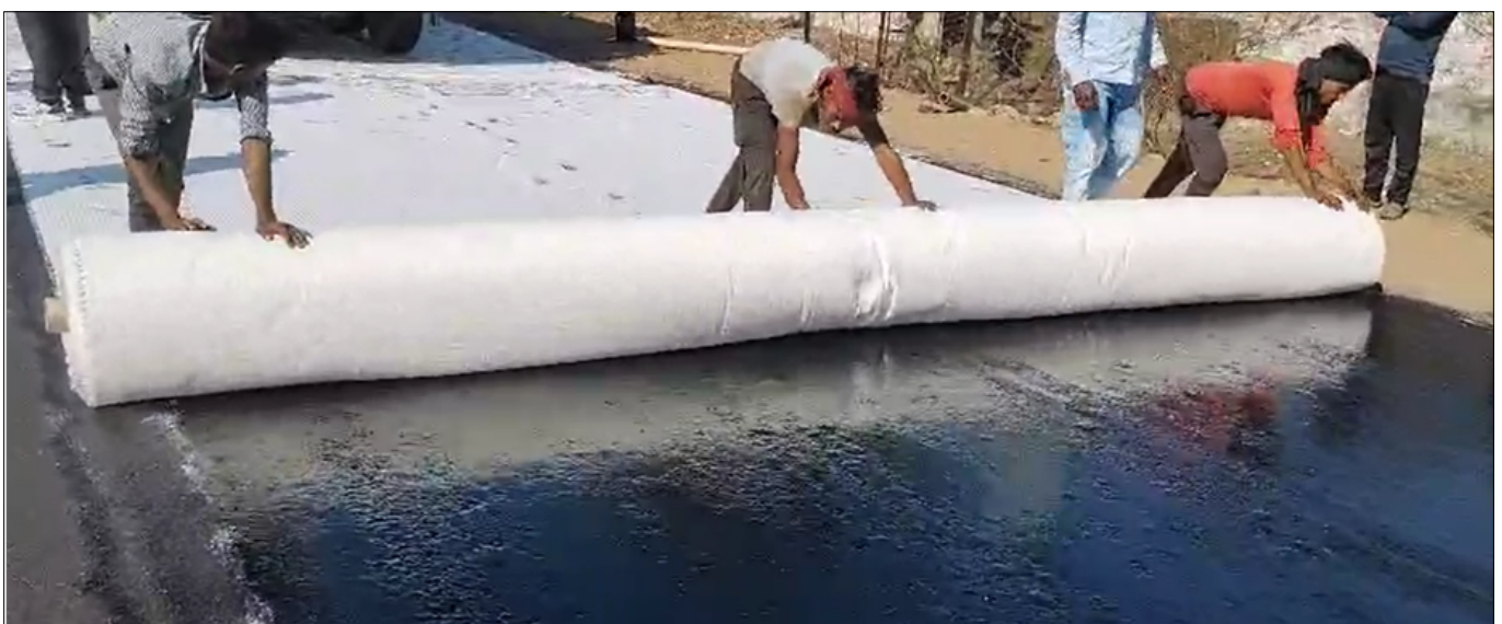
Photo 3 : Laying of AIC Fabric on Tack Coat
