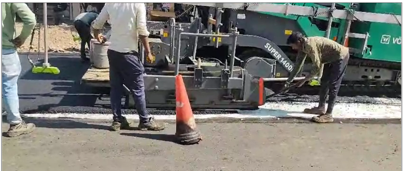
Photo 4 : Preparation of BC (Bituminous Concrete) Layer
