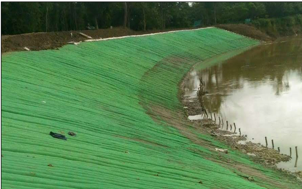
Figure 3: After Completion Photograph
