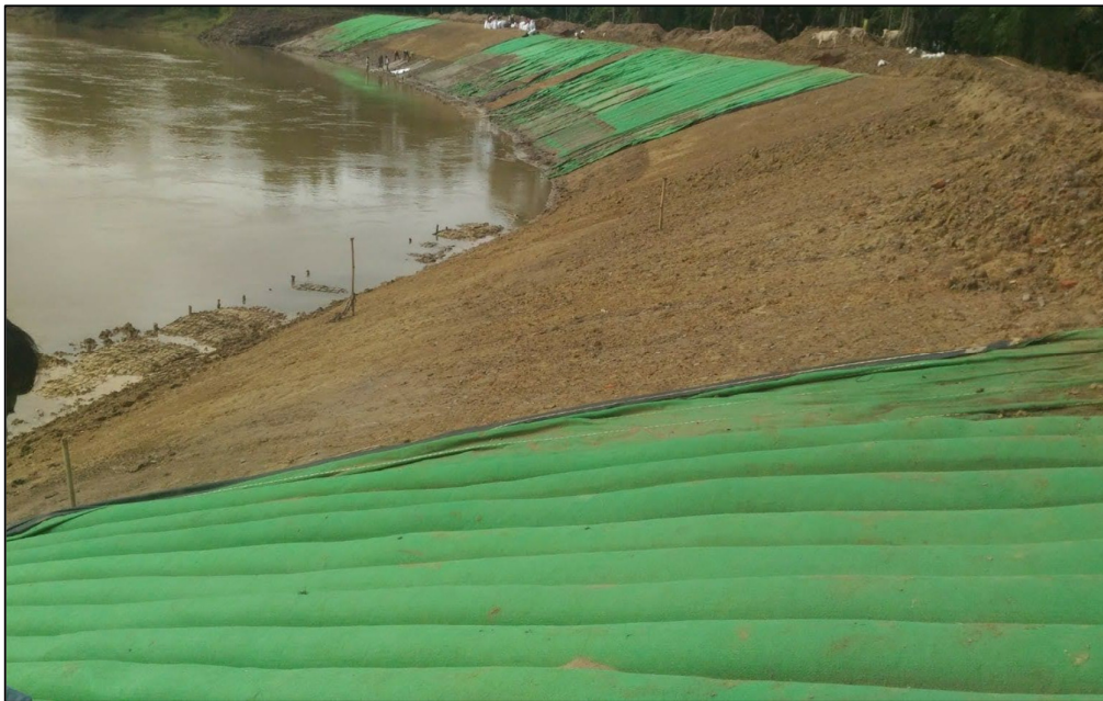
Figure 3: Laying of TechGeo Mattress on Dressed Slope
