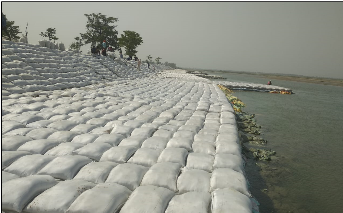
Figure 3 Photograph after Construction
