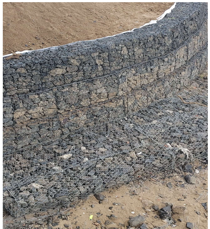
Photo 3 & 4 : Completed Structure - TechFab Metal Gabion & Mattress
