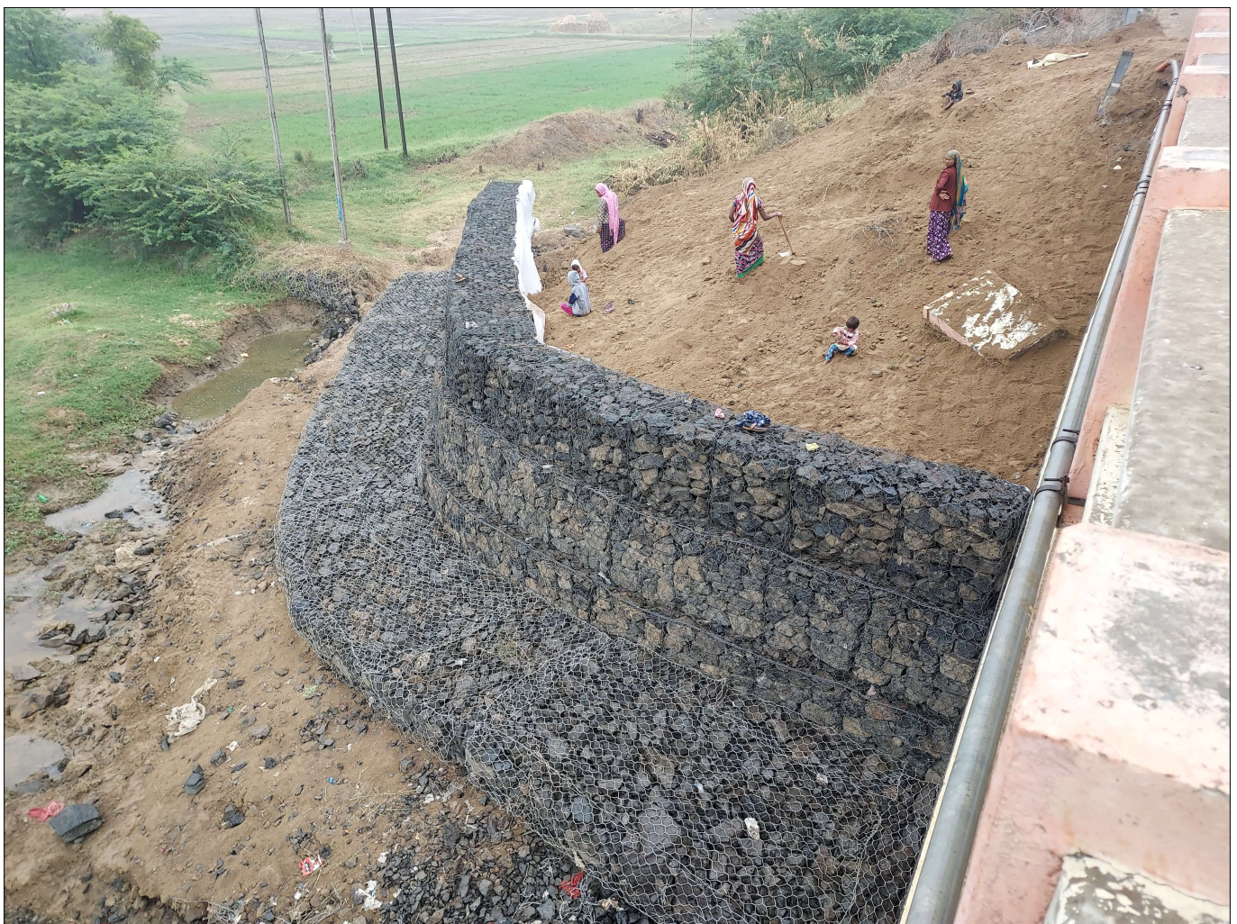
Photo 2 : During Construction Photographs
