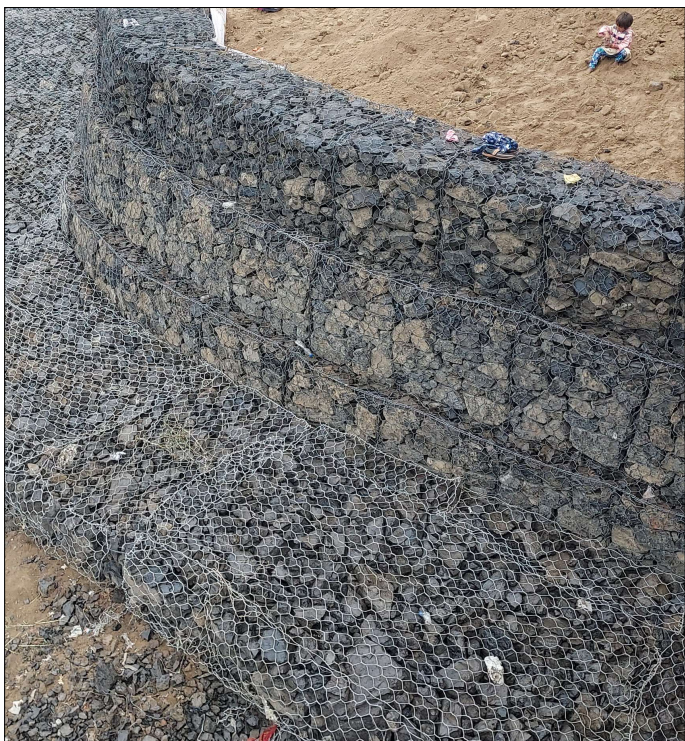
Photo 3 & 4 : Completed Structure - TechFab Metal Gabion & Mattress
