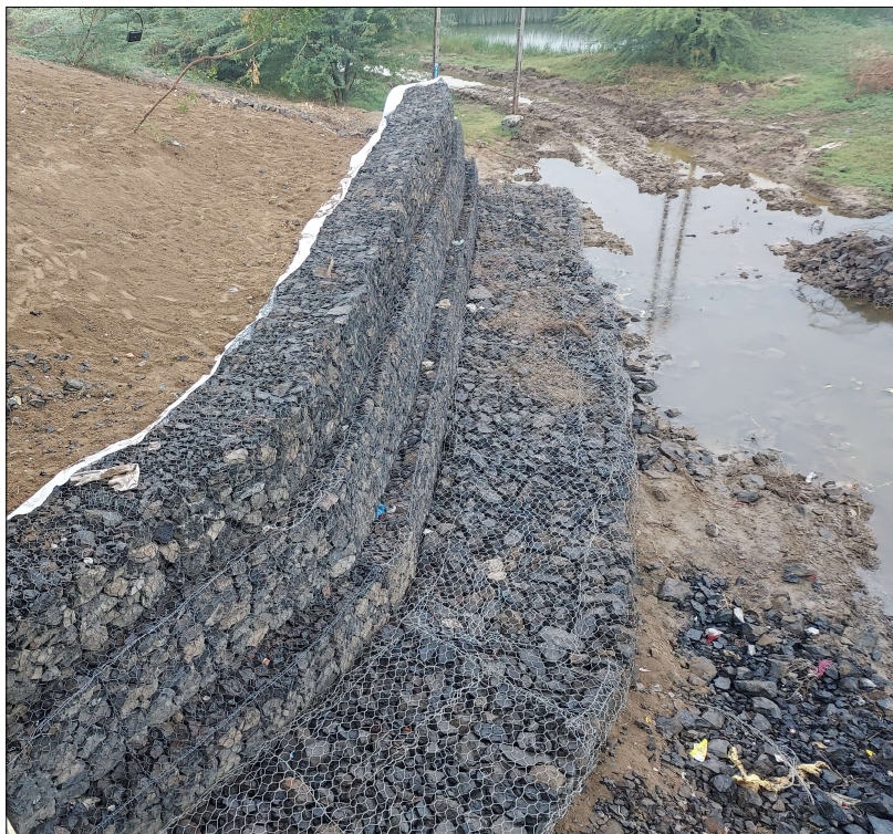
Photo 1 : During Construction Photographs
