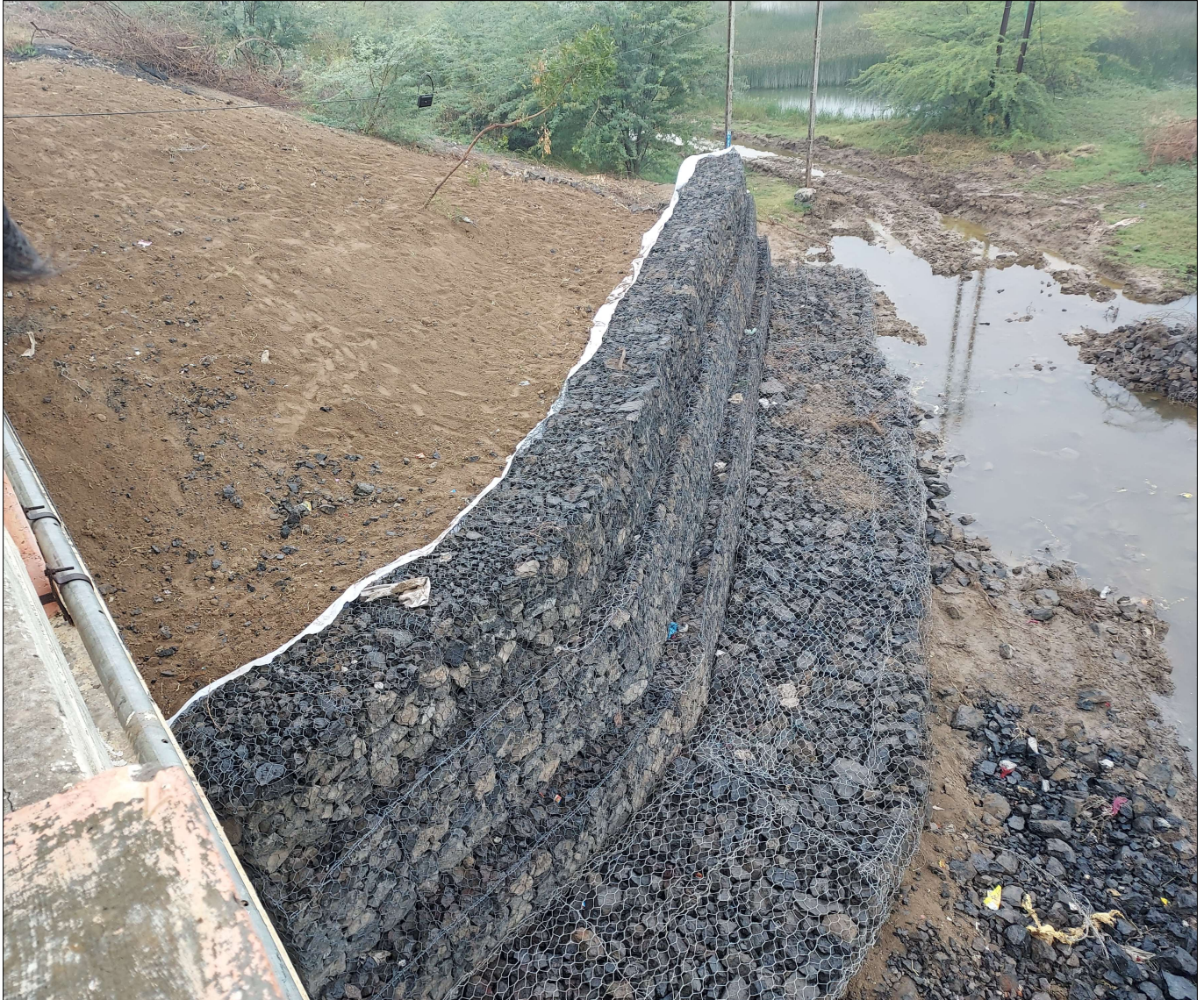
Photo 5 : Structure After Construction
