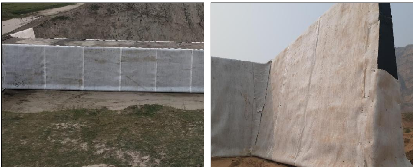
After Installation of TFI Drainage Geocomposite - TechDrains
