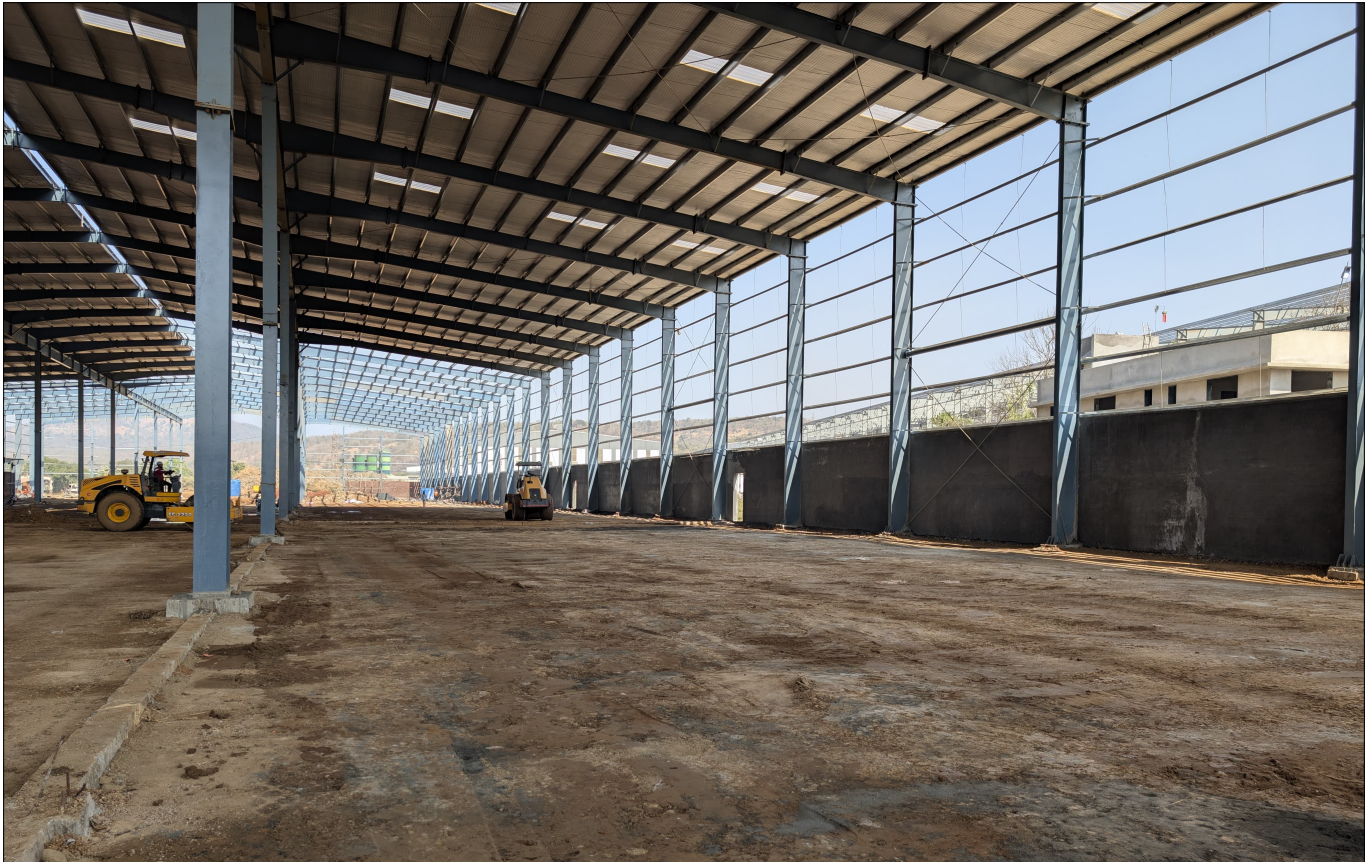
Photo 1 : Proper compaction of subgrade fill at OMC & MDD.
