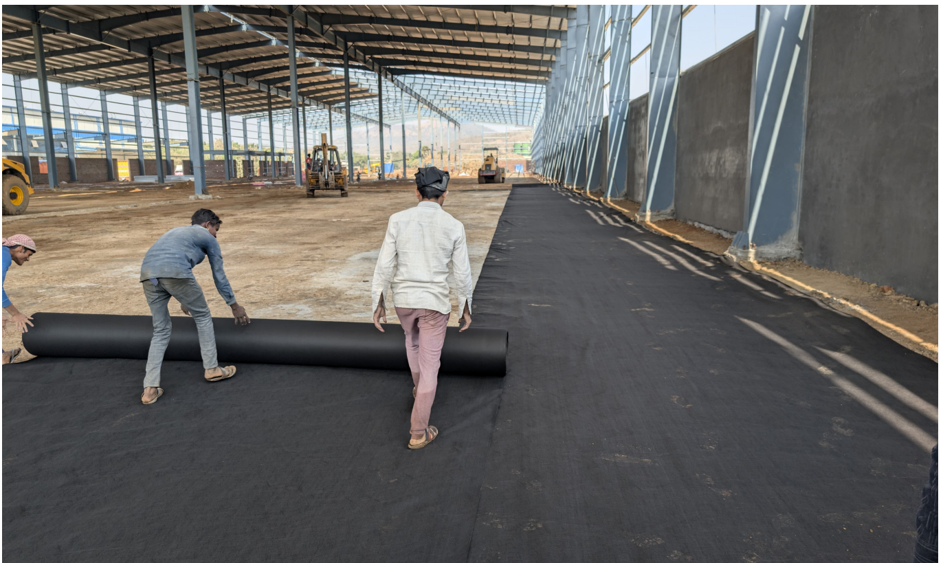
Photo 2 : Lying of Non woven Geotextile PR20 above the subgrade.
