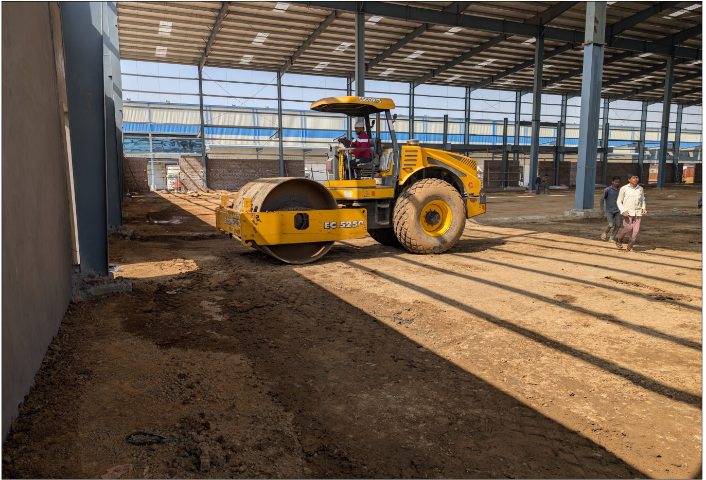
Photo 5 : Compaction and finishing of the cover layer.
