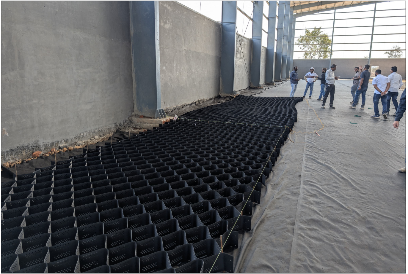
Photo 3 : Laying and fixing of Geocell over the non woven geotextile.
