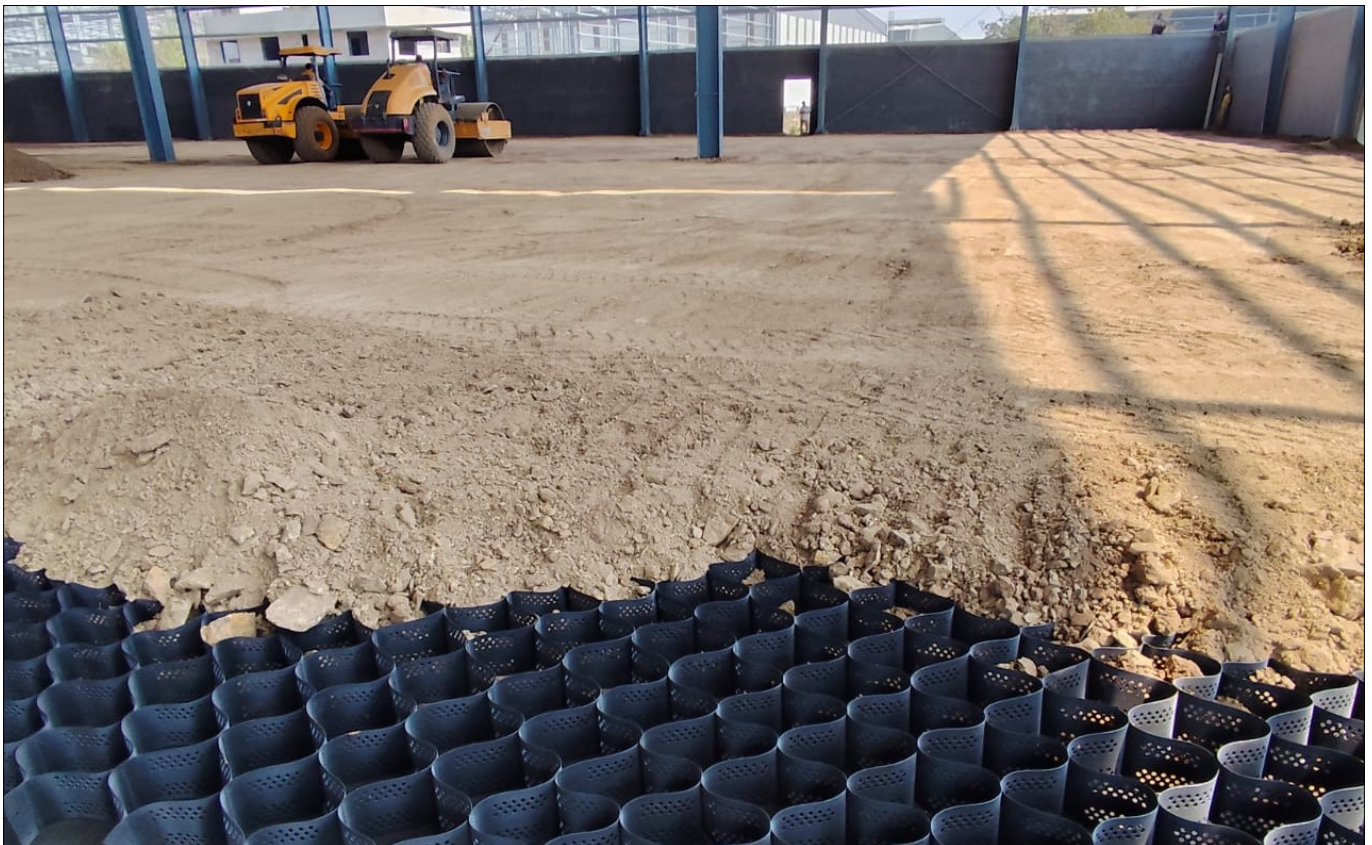
Photo 4 : Filling of Geocells with granular fill and compaction.
