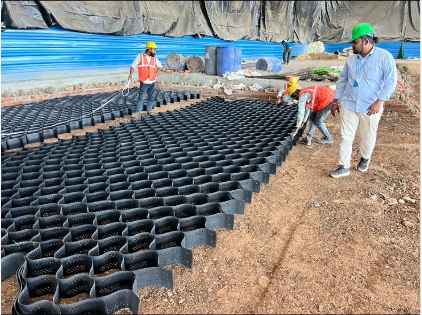
Figure 3 : Installation of TechCell Geocell
