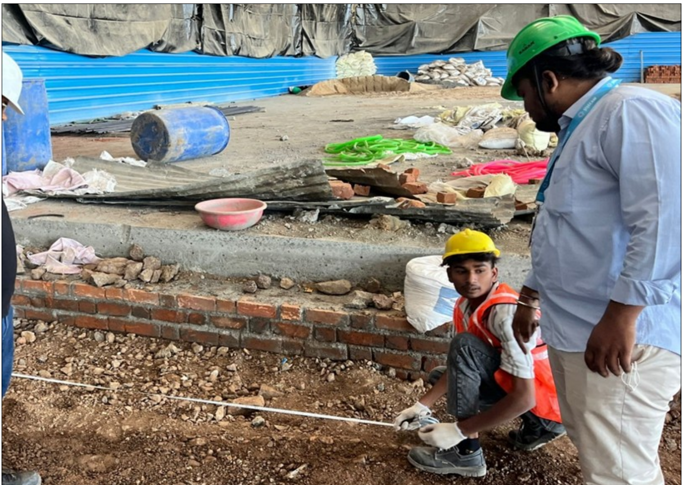
Figure 2: Line Marking for TechCell Geocell Installation
