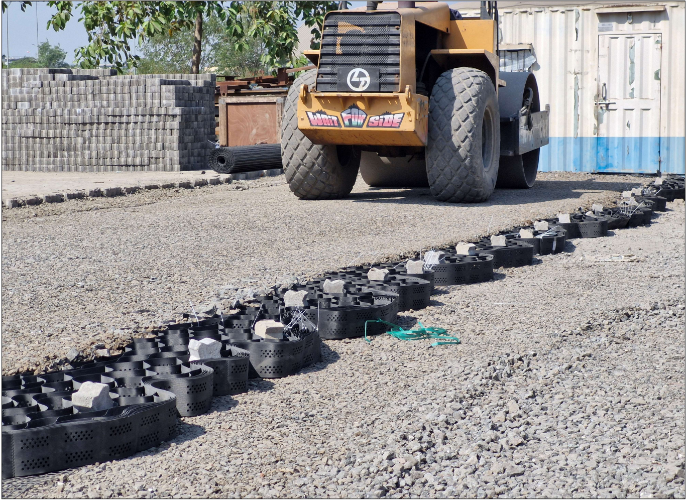
Figure 5 : Installation of Products at the site
