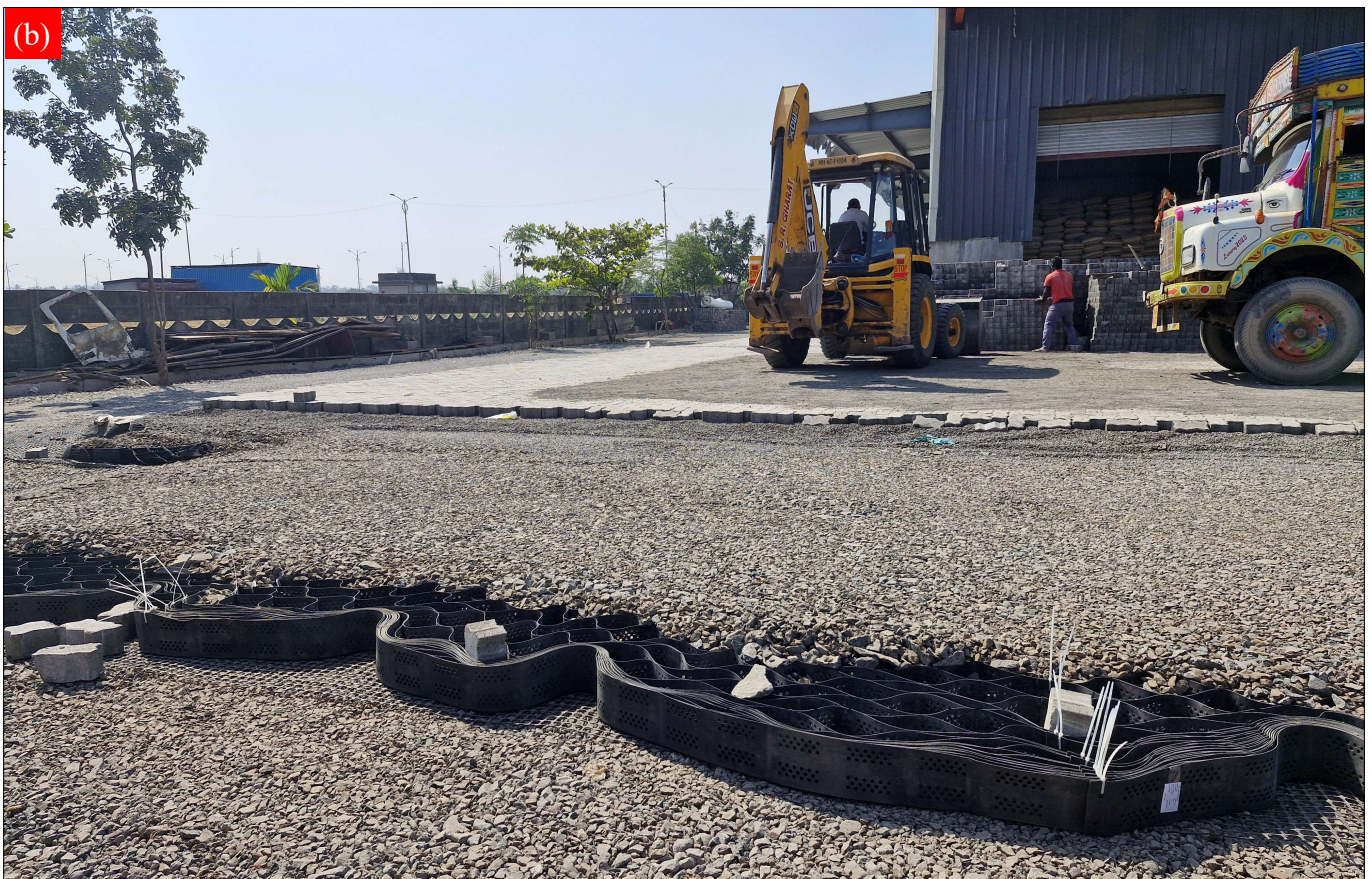
Figure 4 a & b : Installation of Products at the site
